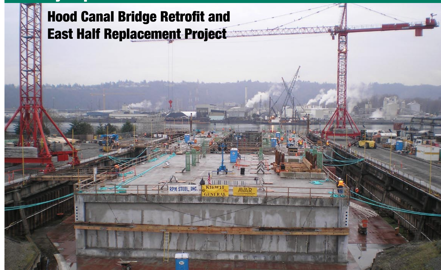
Workers prepare for the first cycle pontoon float-out. December 5, 2006
