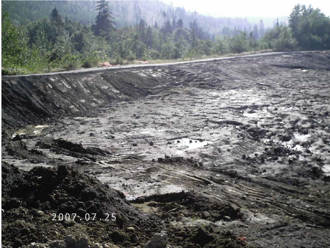
25-July-2007. Dirt removed from Shotwell Recycling Facility
