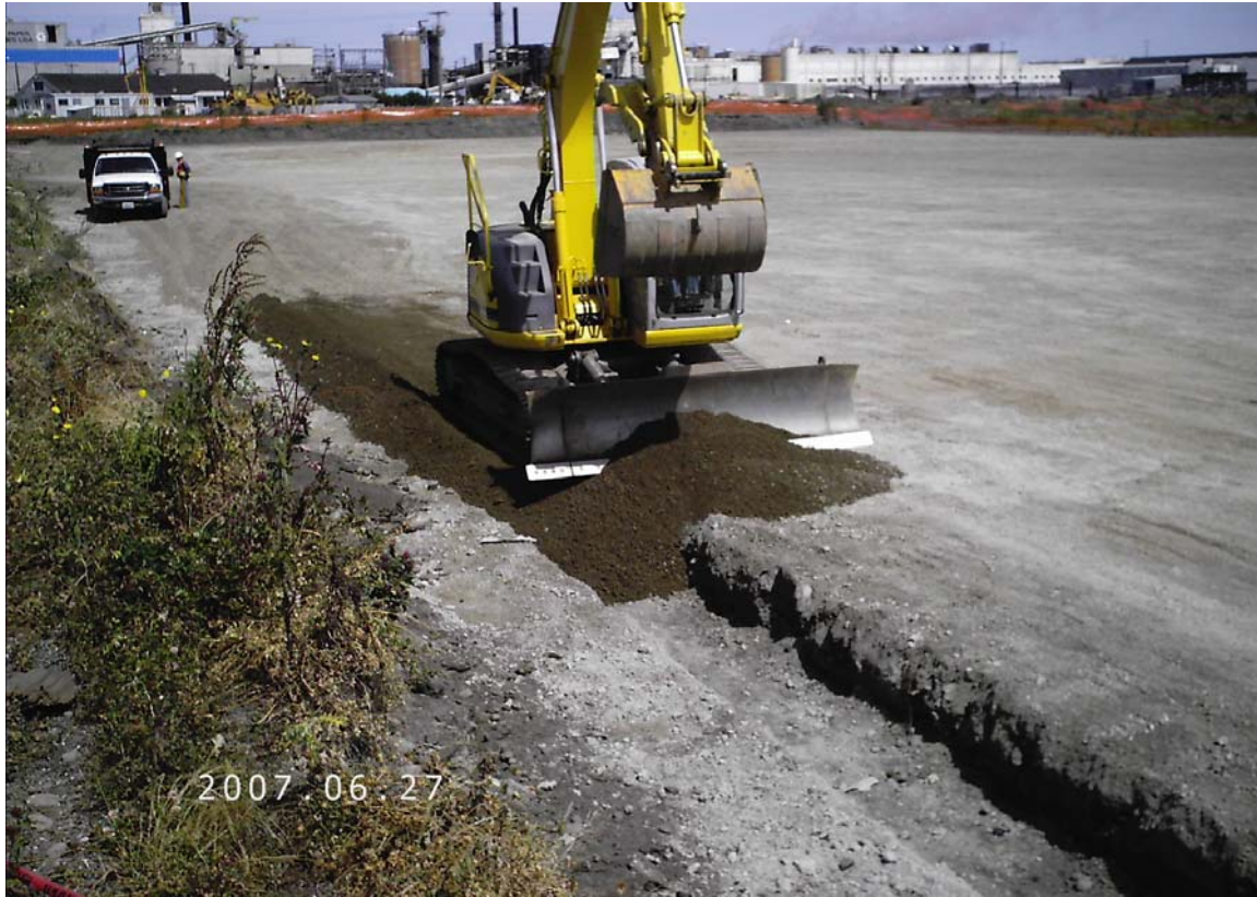
27-June-2007. Backfilling area where trench drain was removed.
