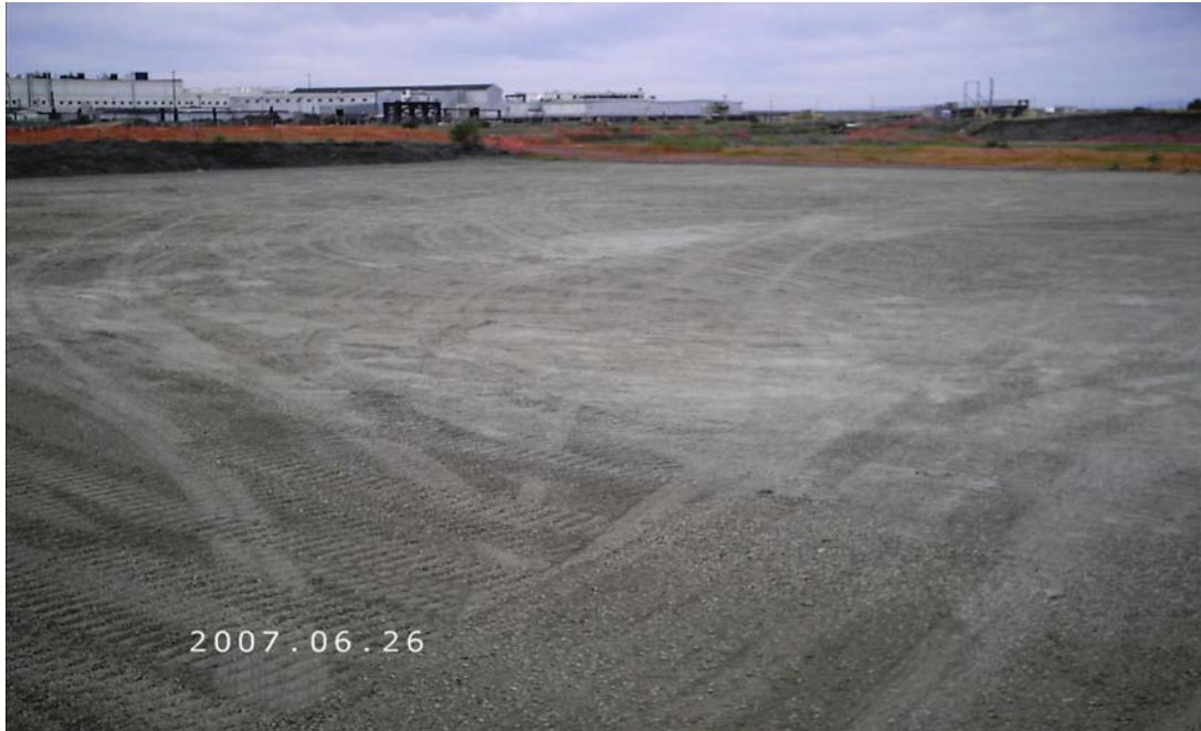
26-June-2007. View of area where concrete pad once was.
