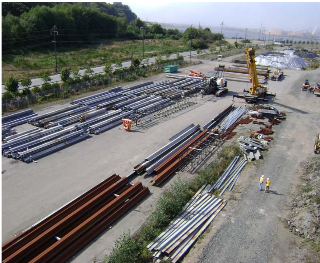
10-September-2007. Stacking sheet pile for removal from site.
