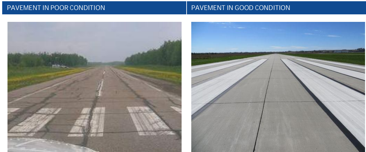
Figure 6-1. Example of Pavement Conditions
