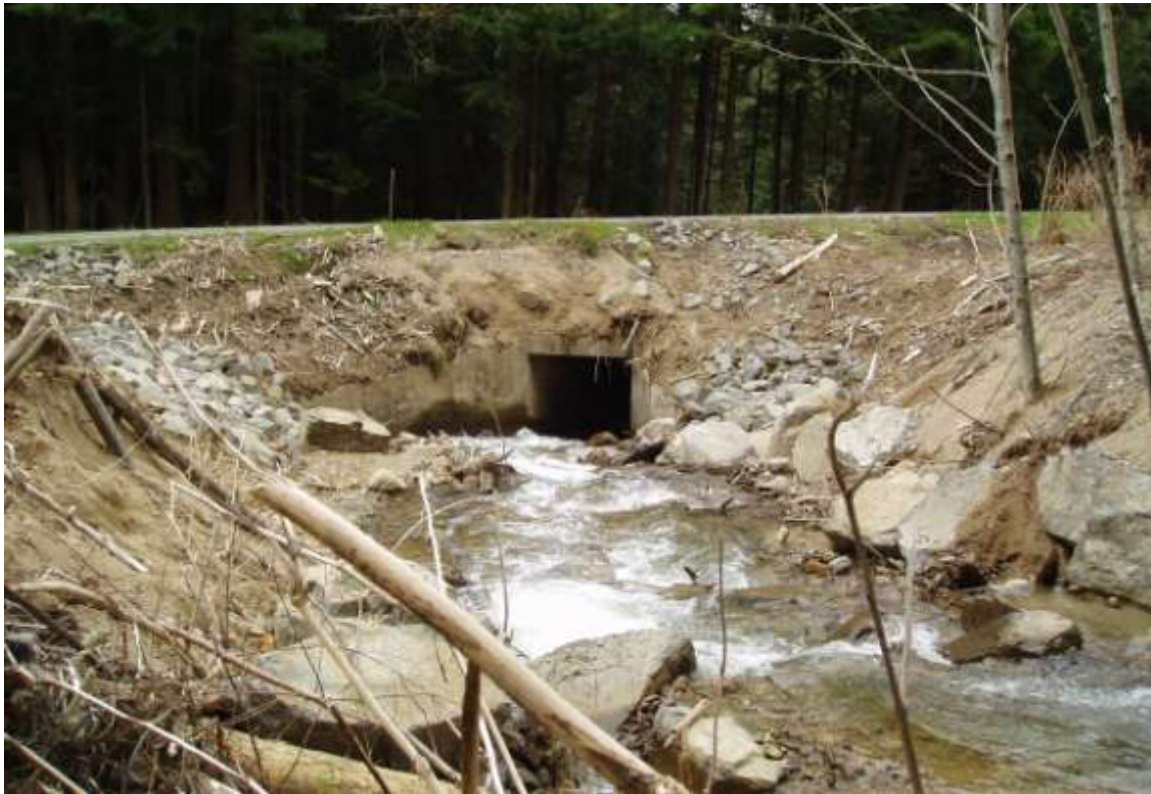
Figure 1. Photo of the Culvert Inlet after the 2009 Repair.
