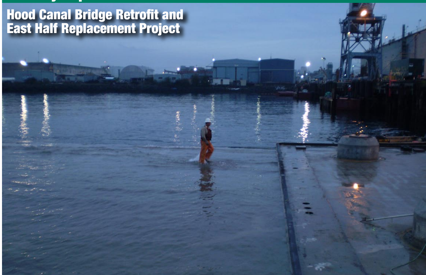
Water washes over pontoon YF as it descends during test procedures, November 7, 2007.
