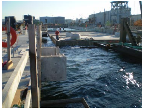
A tugboat tows pontoon YF away from the pier before mating to pontoons PA and PB, November 5, 2007.
