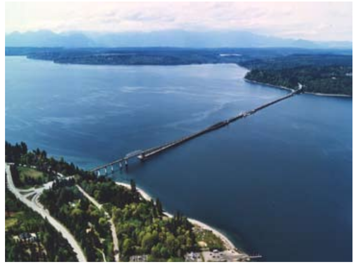
An aerial view of the Hood Canal Bridge.
