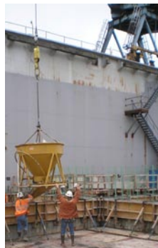
Crews pour concrete into a 46-foot anchor, March 12, 2007
