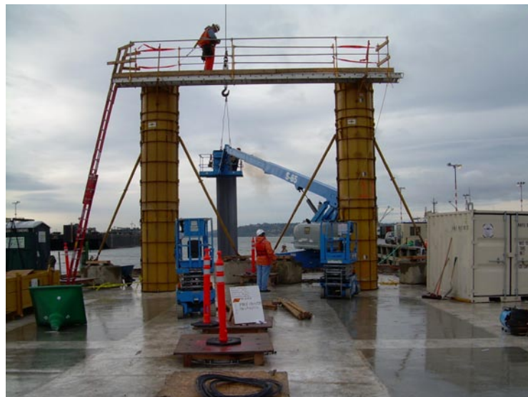
Steel forms in place for pontoon T columns, March 23, 2007.
