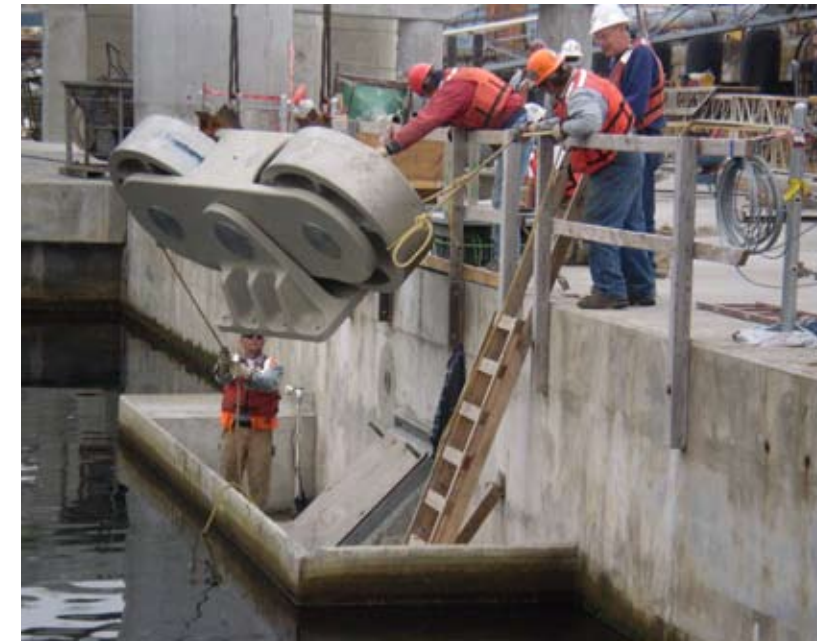
(left) Pilebucks install a lower roller guide assembly on the new east half draw span. May 13, 2008. (right) K-G crews place concrete for the bottom slab of pontoon U. May 1, 2008.
