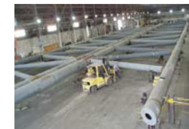
OIW workers position the diagonal supports for weldings. May 19, 2008.
