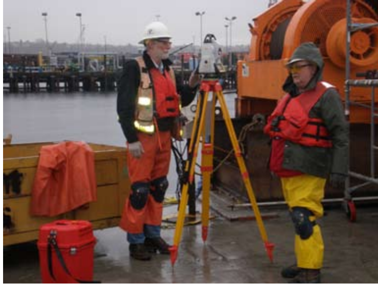
Survey crews at TPS take measurements to determine the precise locations and elevations for the pontoon columns and roadway. Jan. 3, 2008 and Feb. 28, 2008, respectively.
