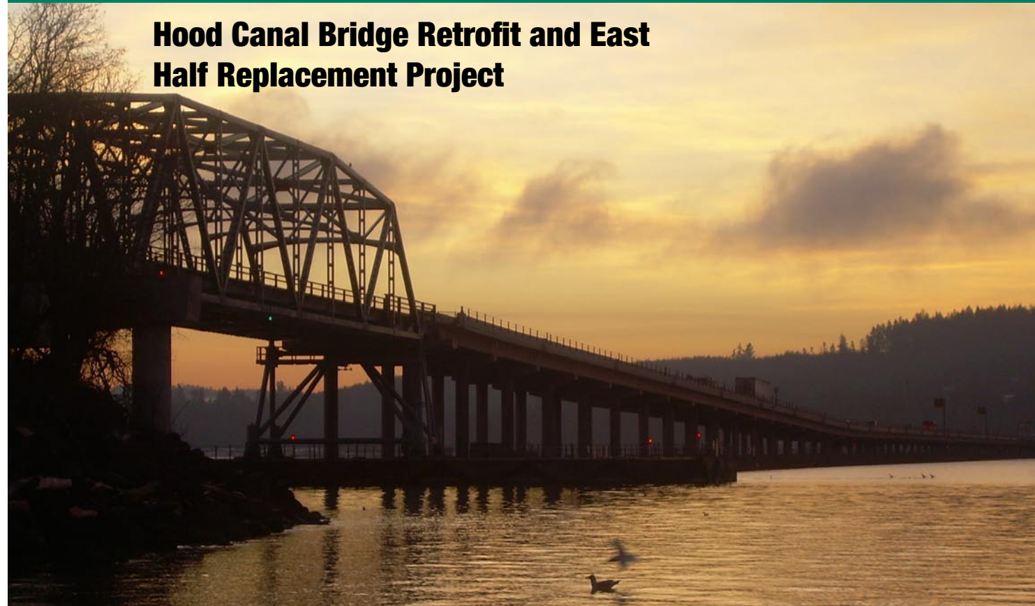
Hood Canal Bridge at sunrise, Feb. 2, 2007.
