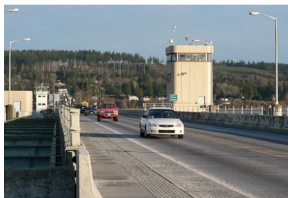
Drivers cross Hood Canal Bridge, Sept. 19, 2006.
