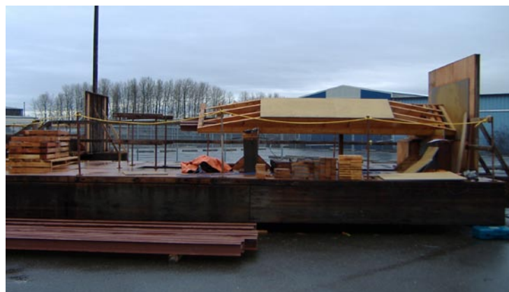
Flat panel form being built on a raised fabrication bed, Jan. 13, 2006.
