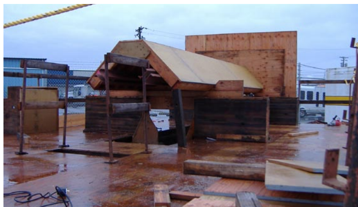
Corner forms being built on a raised fabrication bed, Jan. 13, 2006.
