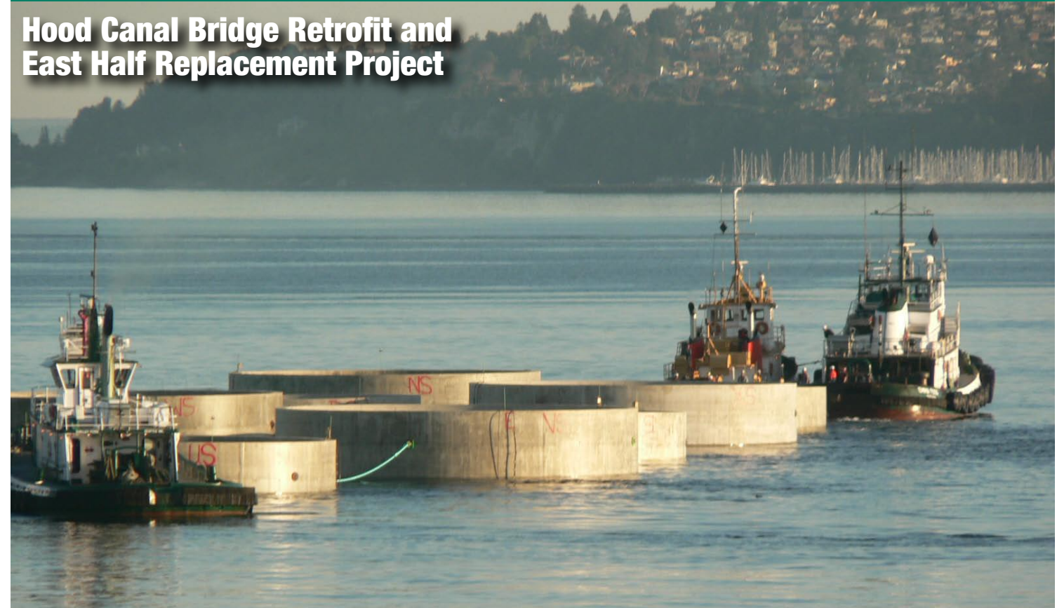
Tug boats tow the anchors out of the dry dock. June 20, 2007.
