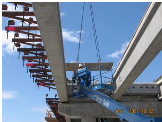
Workers set a deck panel on pontoon S. June 11, 2007.
