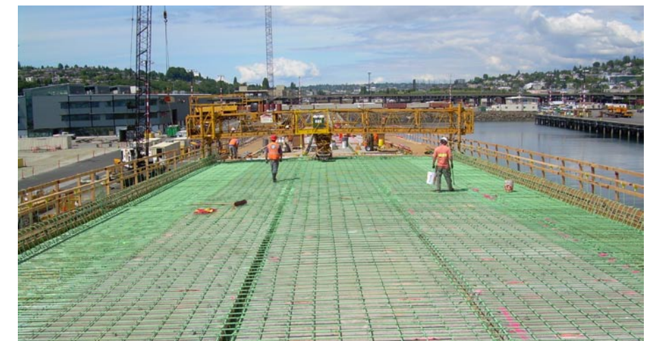
Workers check the rebar on pontoon T. June 14, 2007.
