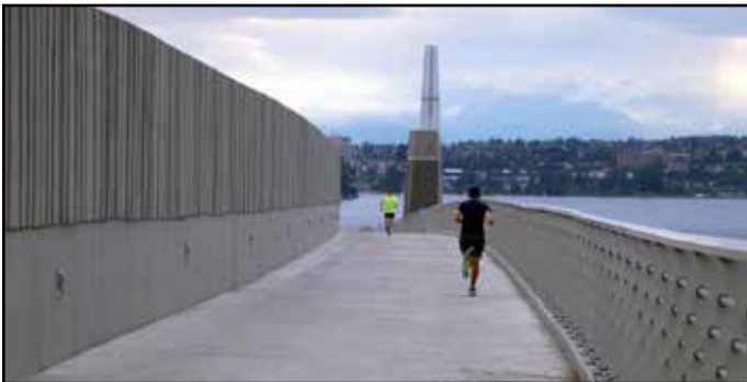
Runners enjoy the new SR 520 regional shared-use path, now open from Bellevue to Seattle.
