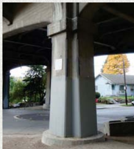
Figure 2. Cruciform-Shaped Bridge Column.
