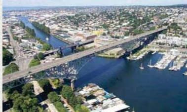
Figure 1. Aurora Avenue Bridge in Seattle.
