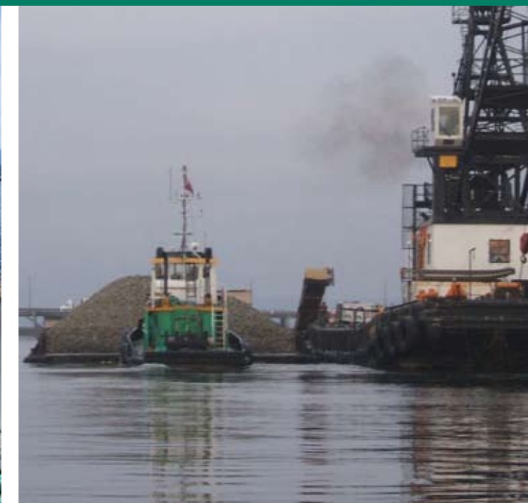
Barge maneuvers into place above underwater anchor, August 2007.
