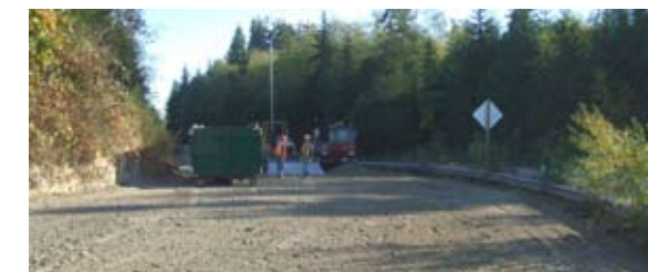
Workers smooth surface for Park-and-Ride lot, October 11, 2006.
