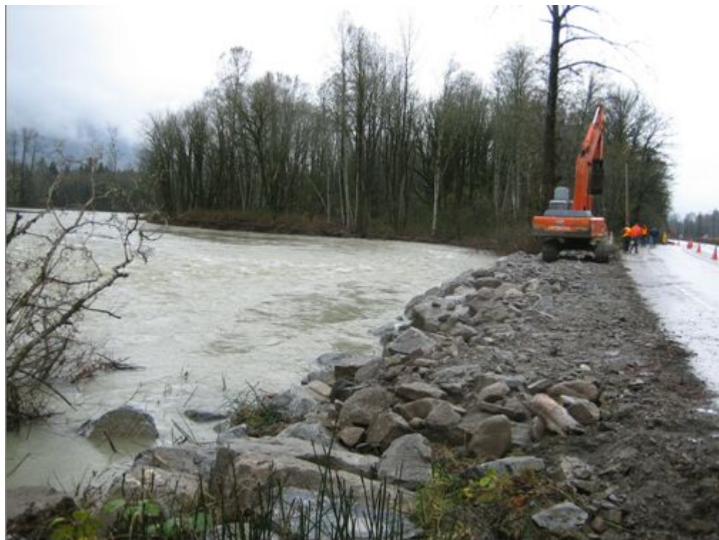
Figure 6. 2006 repair, looking downstream.
