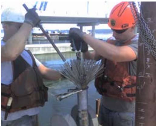
(Upper left) Crews wrap the anchor cables with wire – a process that keeps the cable strands from unraveling when any excess is cut off. June 17, 2009. (Lower left) Once the cable is wrapped, crews “broom” the ends in preparation for the socket installation. Molten zinc is then poured into the socket to protect the cable from corrosion. July 22, 2009. (Right) WSDOT and Kiewit-General completed anchor cable connections on the new east half of the SR 104 Hood Canal Bridge Aug. 18, preparing the bridge for winter weather. Aug. 7, 2009.
