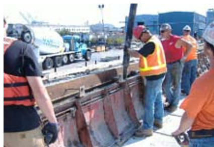
Crews place concrete on Z pontoons spans. Sept. 16, 2008.
