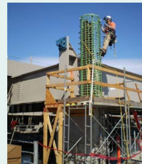
A worker installs a spiral rebar cage for a column. Sept. 4, 2008.
