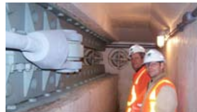
Anchor cable sockets are filled with molten zinc to give them additional protection.
