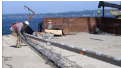
Crews replace anchor cables and jewels.
