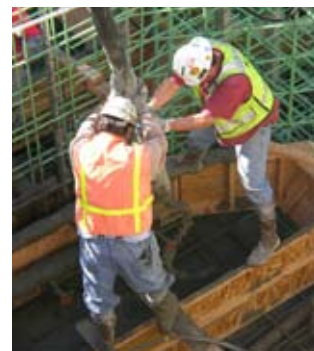
(Left) A K-G crew member clamps jewelry – including zinc anodes – onto an anchor necklace. May 2005. (Center) Epoxy-coated rebar covered with concrete is designed to protect the bridge's mechanical and electrical. Sept. 11, 2006. (Right) Charging anchor cables with a small electrical current provides cathodic protection and resistance against rust. Sept. 11, 2006
