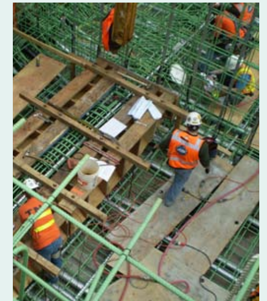
K-G crews place rebar and forms on pontoon U. March 20, 2008.
