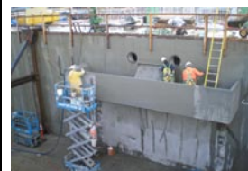
Port of Tacoma—Concrete Technology: Pontoon Construction (33% complete) Workers finish concrete surfaces on roller guide platform walls on pontoon PB after concrete pour, Nov. 22, 2006.
