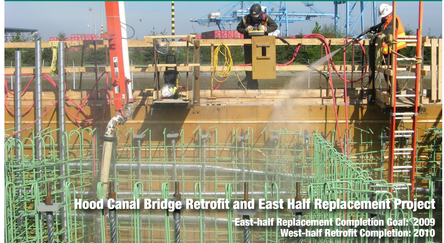
Operator carefully moves truck boom within the pontoon cell to place concrete in just the right location while worker sprays water over concrete as part of the curing process.
