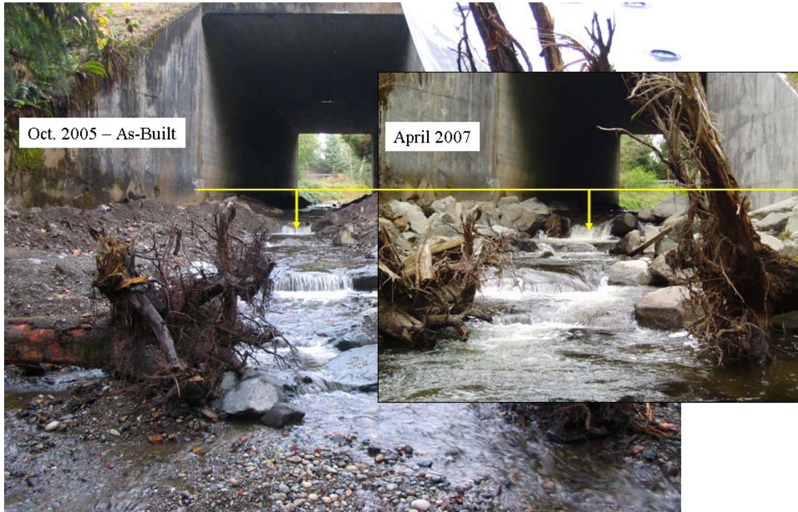
Figure 4. Photos of As-Built and Current Conditions at the Culvert Outlet
