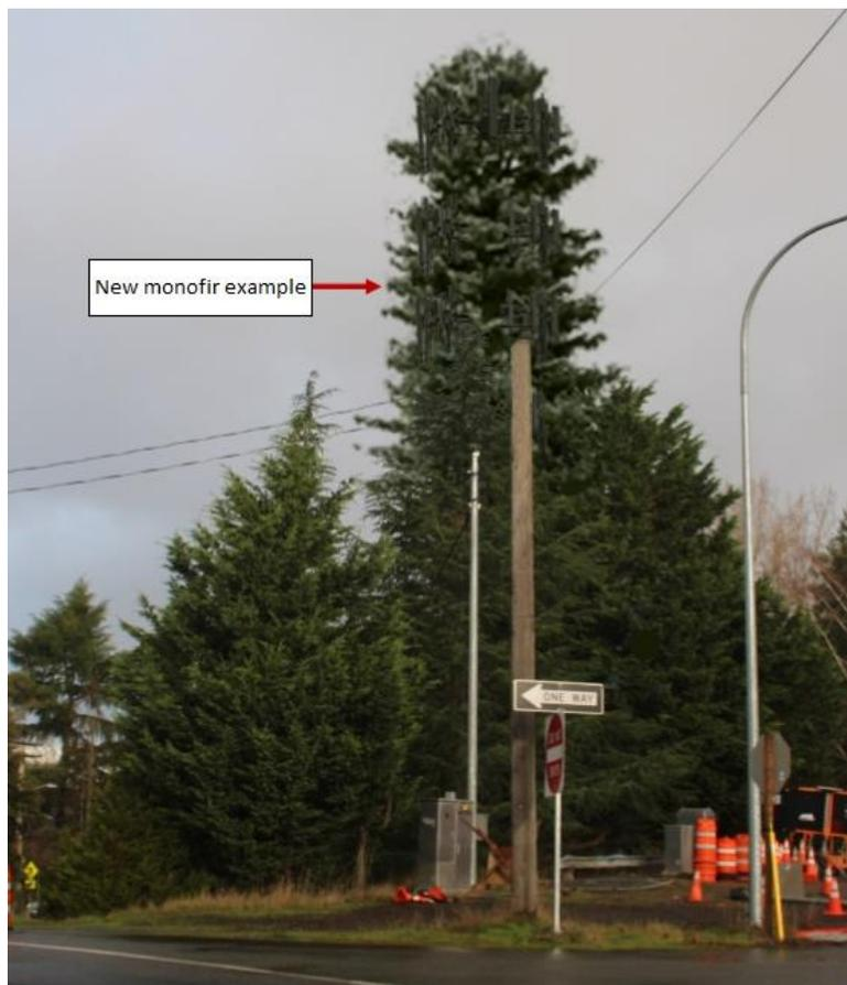
*Photo rendering of the new "monofir" cellular communications facility, looking north.*
