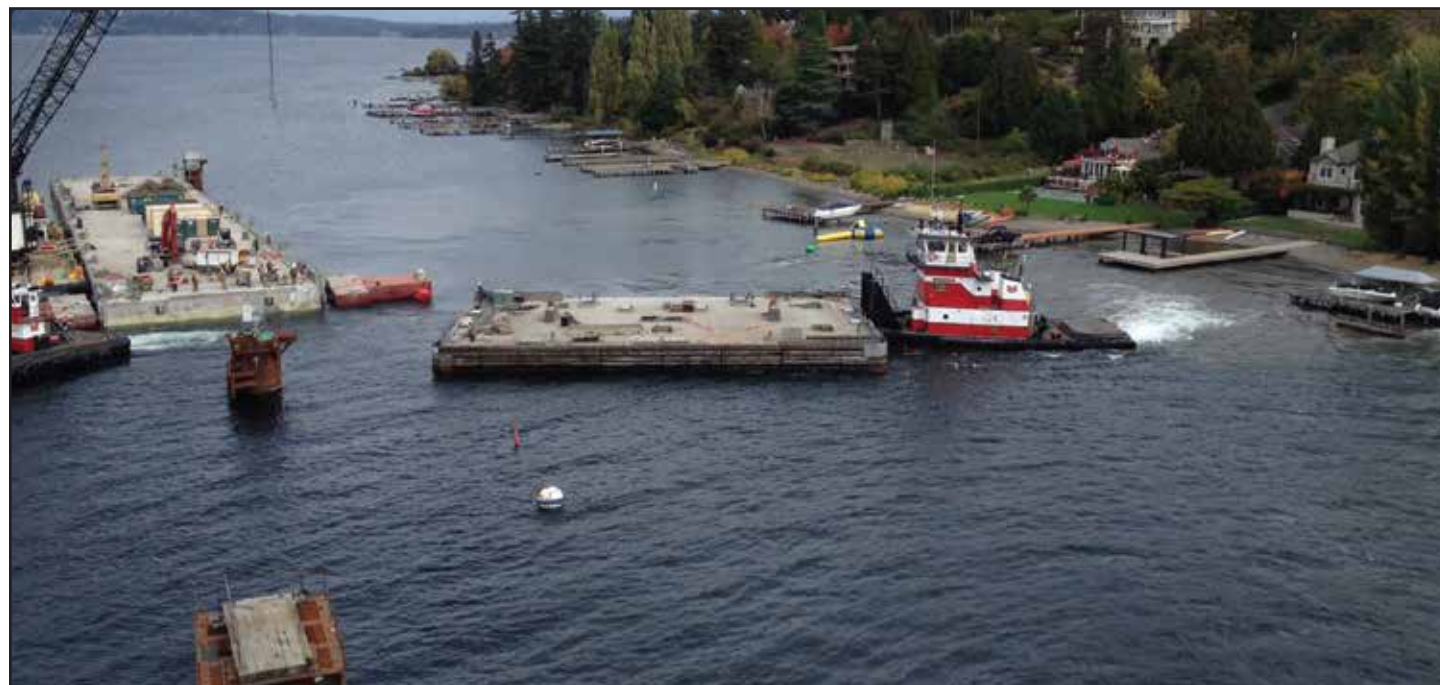
Pontoon A, the westernmost pontoon of the old floating bridge, is separated from longtime neighbor Pontoon B. Both pontoons were later towed intact off Lake Washington through the Ballard locks. Photo taken: Oct. 6
