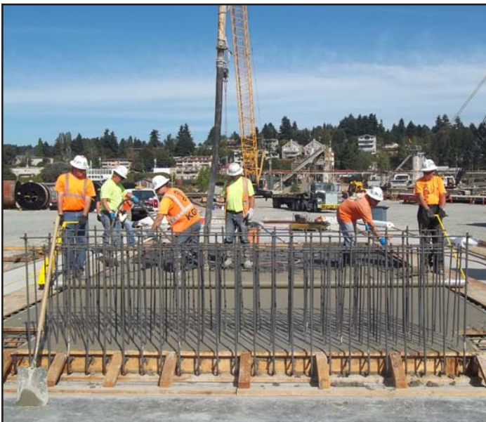
Crews place concrete at the construction site in Kenmore, WA.
