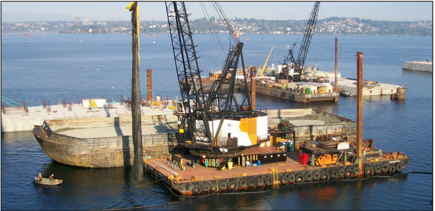
Construction barges complete work alongside new pontoons on Lake Washington.
