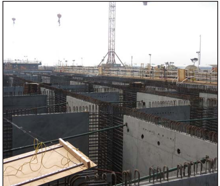
Precast interior walls in a pontoon in Aberdeen, WA.
