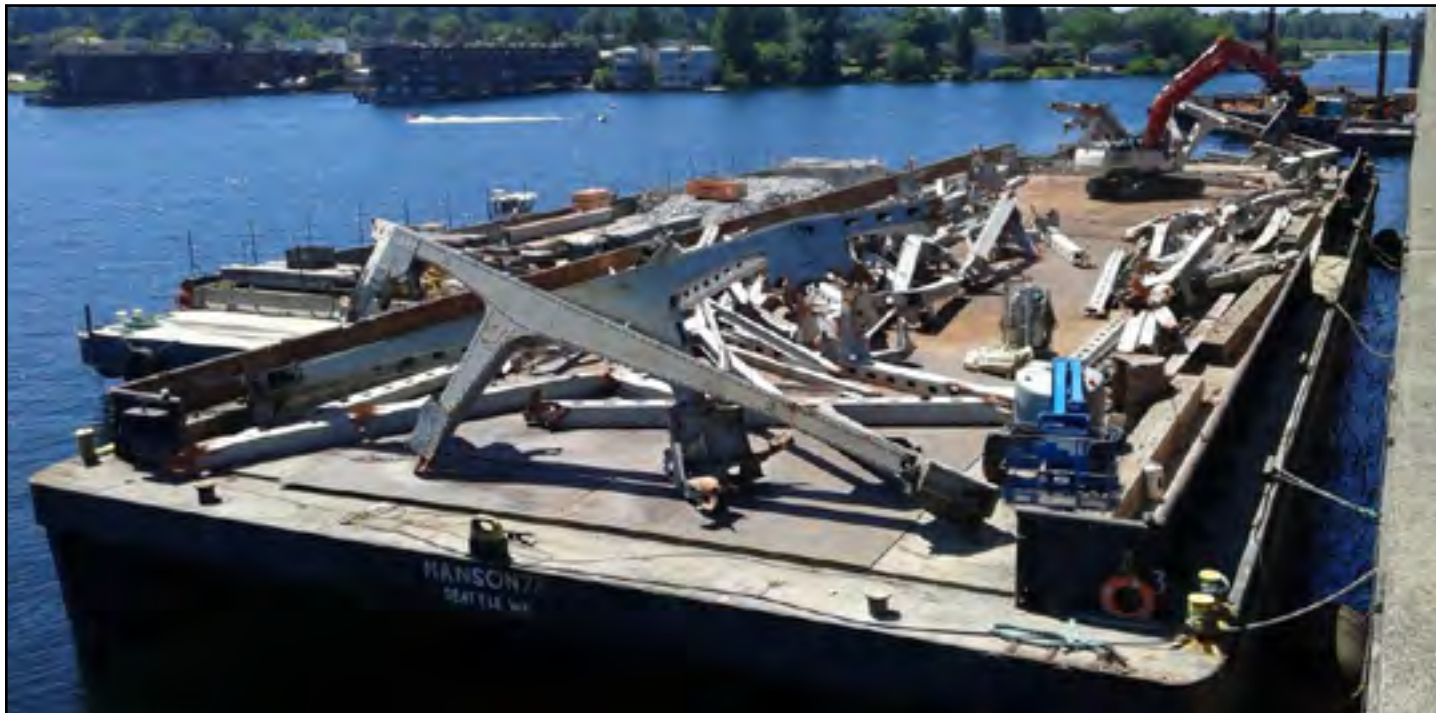
Barge cranes begin taking apart the west truss of the old SR 520 floating bridge for recycling. Photo taken: May 31.
