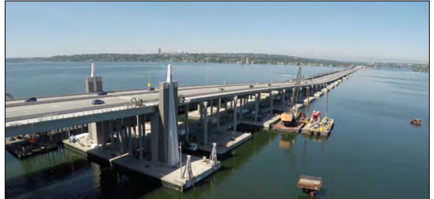
View of the new SR 520 floating bridge after it opened to traffic. Photo taken: May 12.
