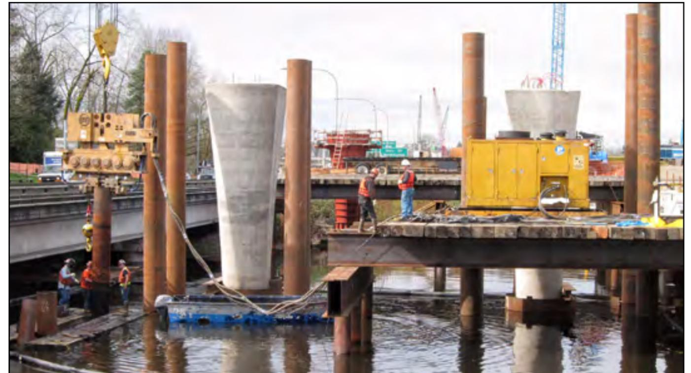
In March, crews began removing finger piers on the temporary WABN work bridge. They reused the steel piles that were removed to build new work-bridge finger piers near the project's Montlake staging area. Photo taken: March 11.
