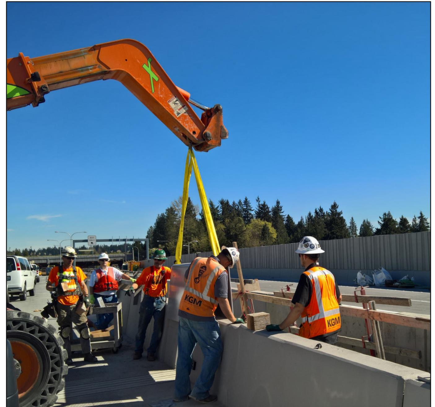
Crews carefully lift the steel barrier for the expansion joint into place at the east end of the bridge. Photo taken: March 30.
