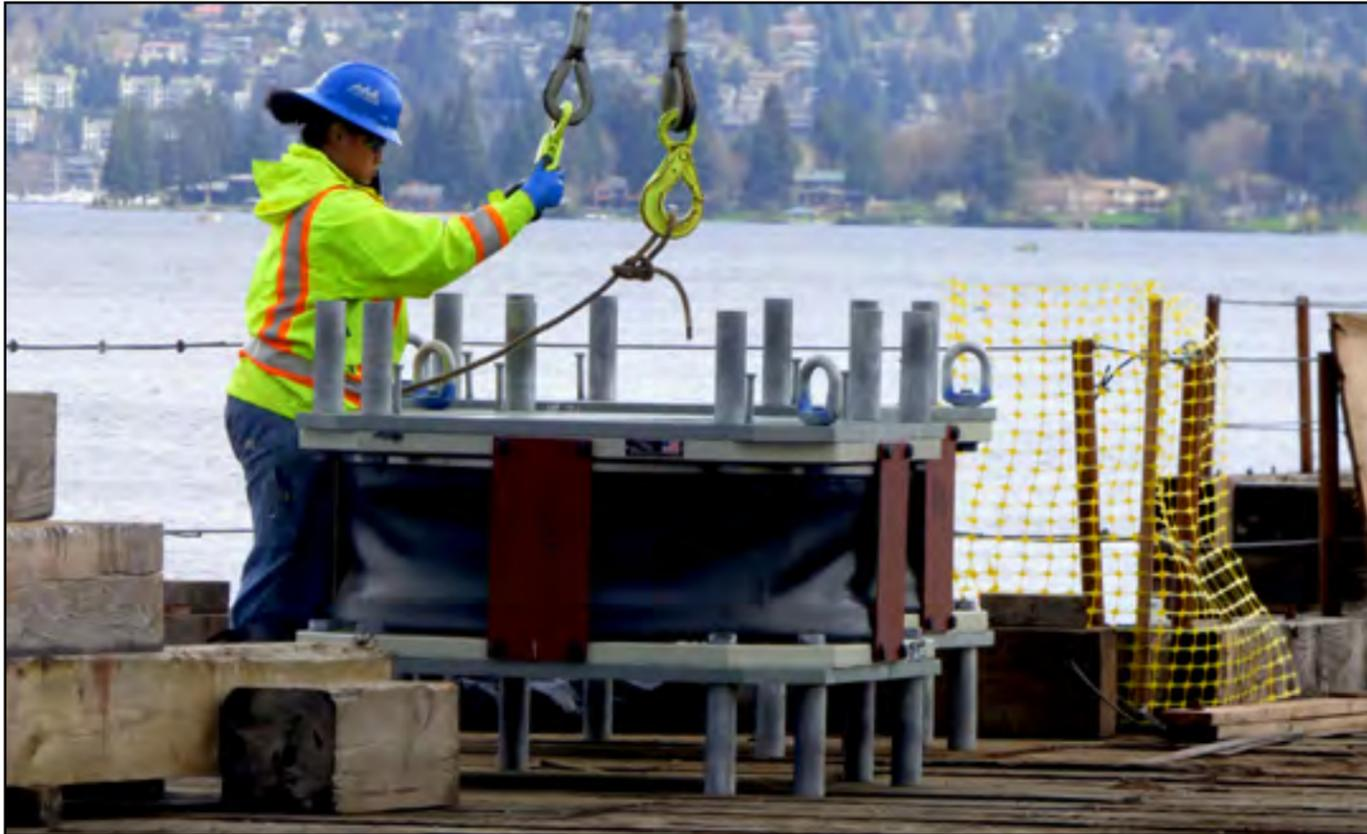
A crew member on the West Approach Bridge North Project prepares a seismic isolation bearing for placement. Photo taken: March 3.
