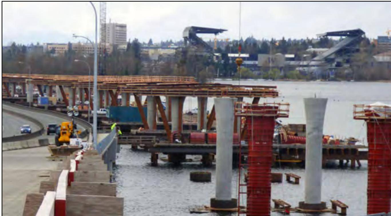
Crews continue to make progress on the West Approach Bridge North Project. By the end of March, crews had installed 58 casings, 53 shafts, 46 columns and 32 isolation bearings. Photo taken: March 3.
