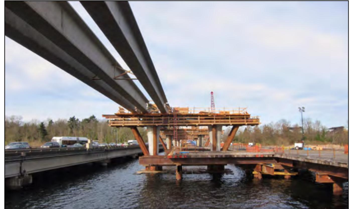
On March 15, crews placed the first girders for the West Approach Bridge North. By the end of March, crews had placed 45 girders. When completed, the new bridge will have 353 girders. Photo taken: March 18
