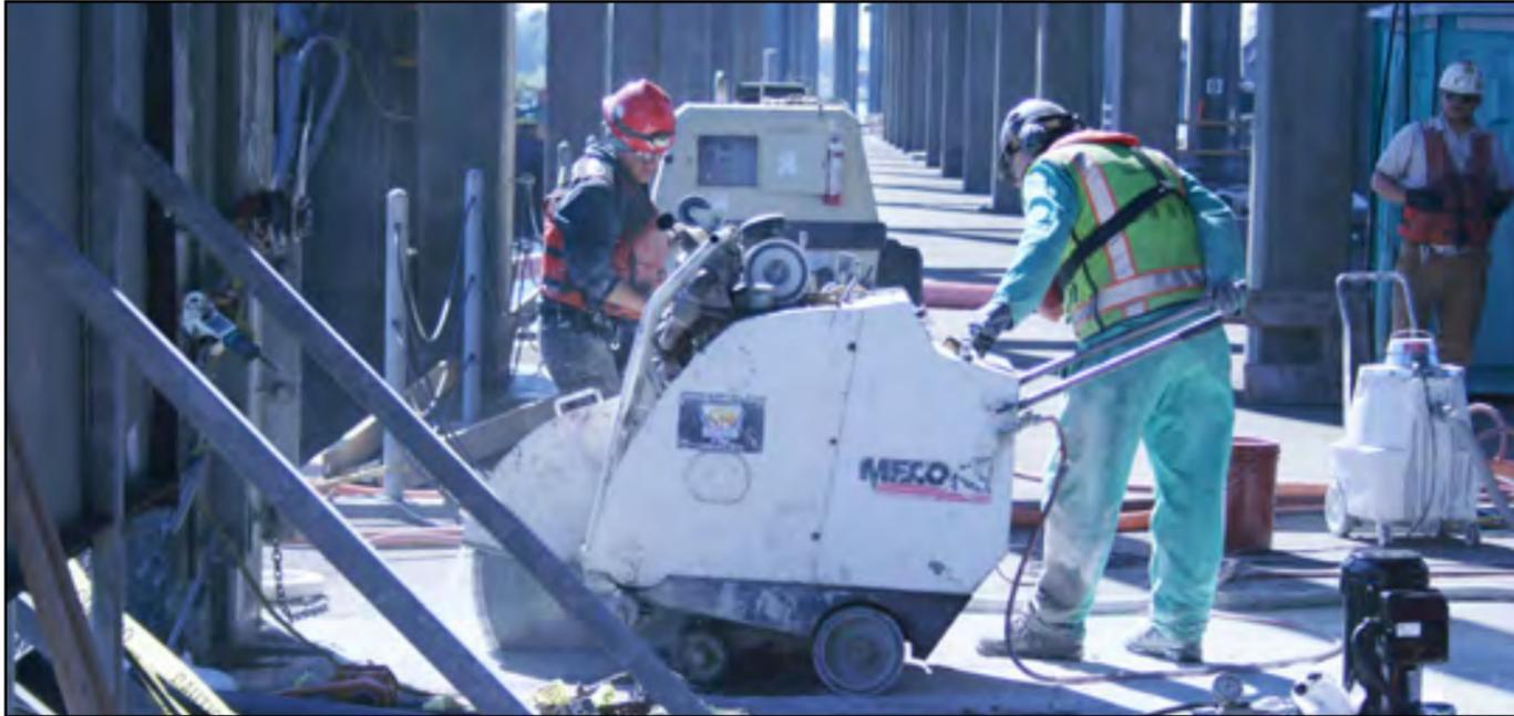
Crews use an industrial saw to cut through the top layer of concrete connecting pontoons on the old floating bridge. Photo taken: June 28.
