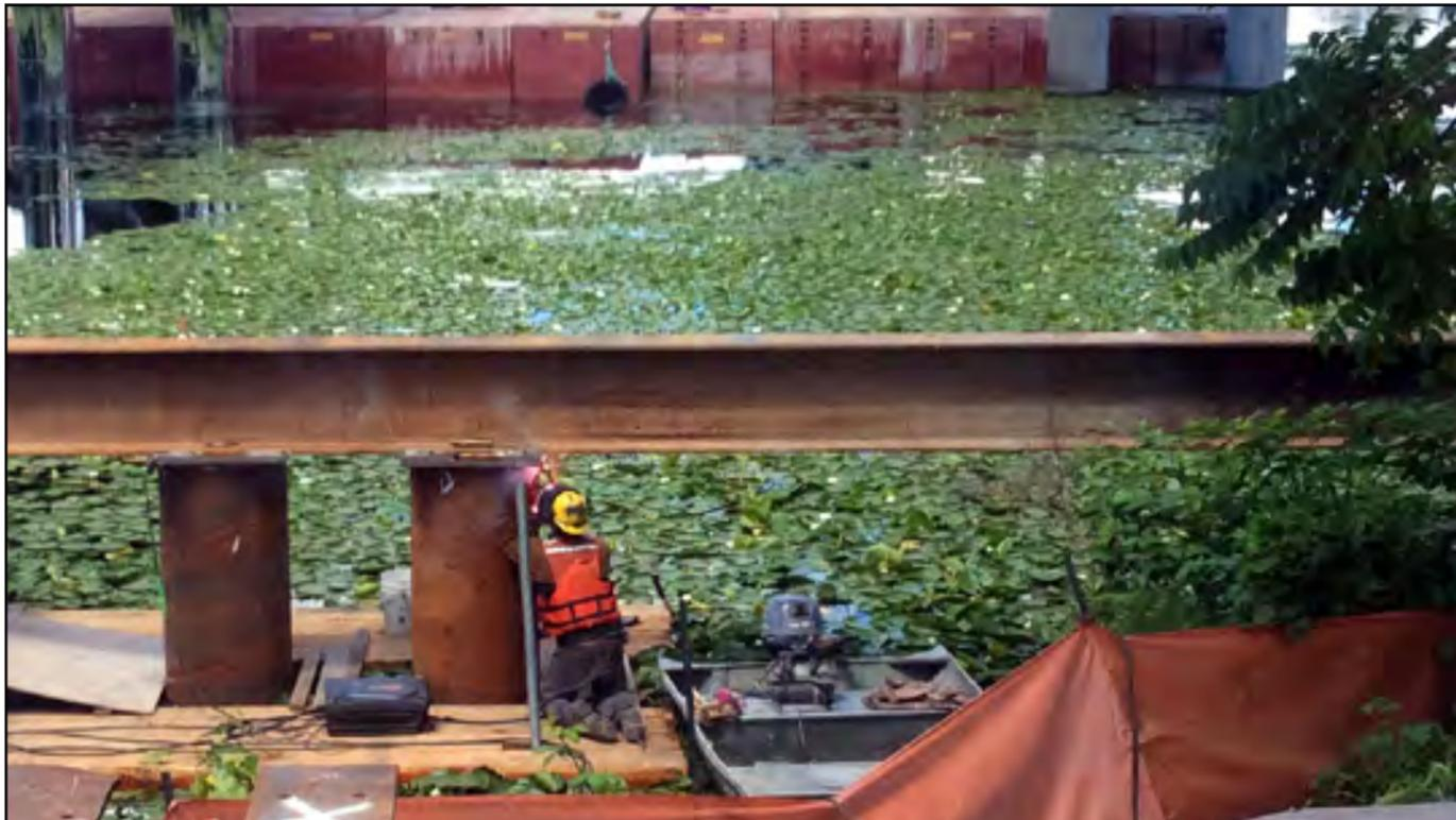
A crew member welds a steel pile to a girder for the temporary work bridge that will be used to off-load demolition debris from the westbound SR 520 off-ramp to Lake Washington Boulevard East and the R. H. Thomson "Ramps to Nowhere." Photo taken: June 14.
