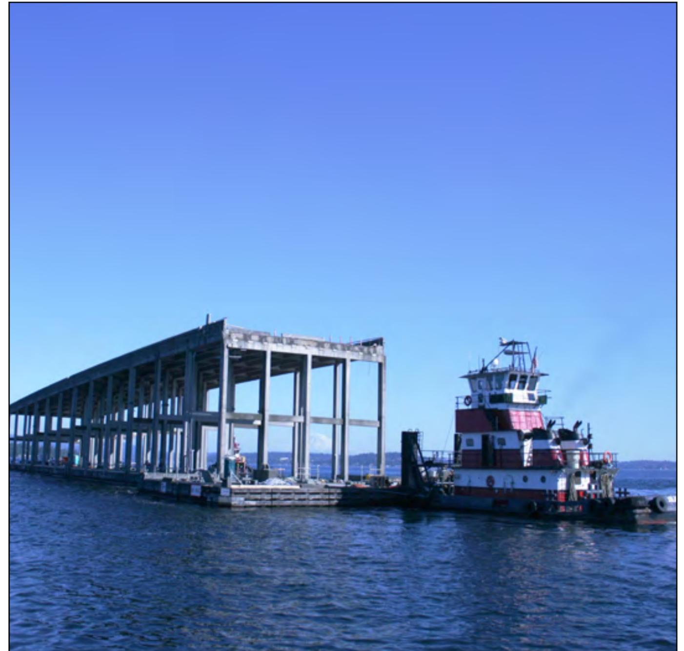
A tugboat pushes pontoons A and B toward the east navigation channel of SR 520 en route to the west side staging area as part of decommissioning of the old floating bridge. Photo taken: June 28.
