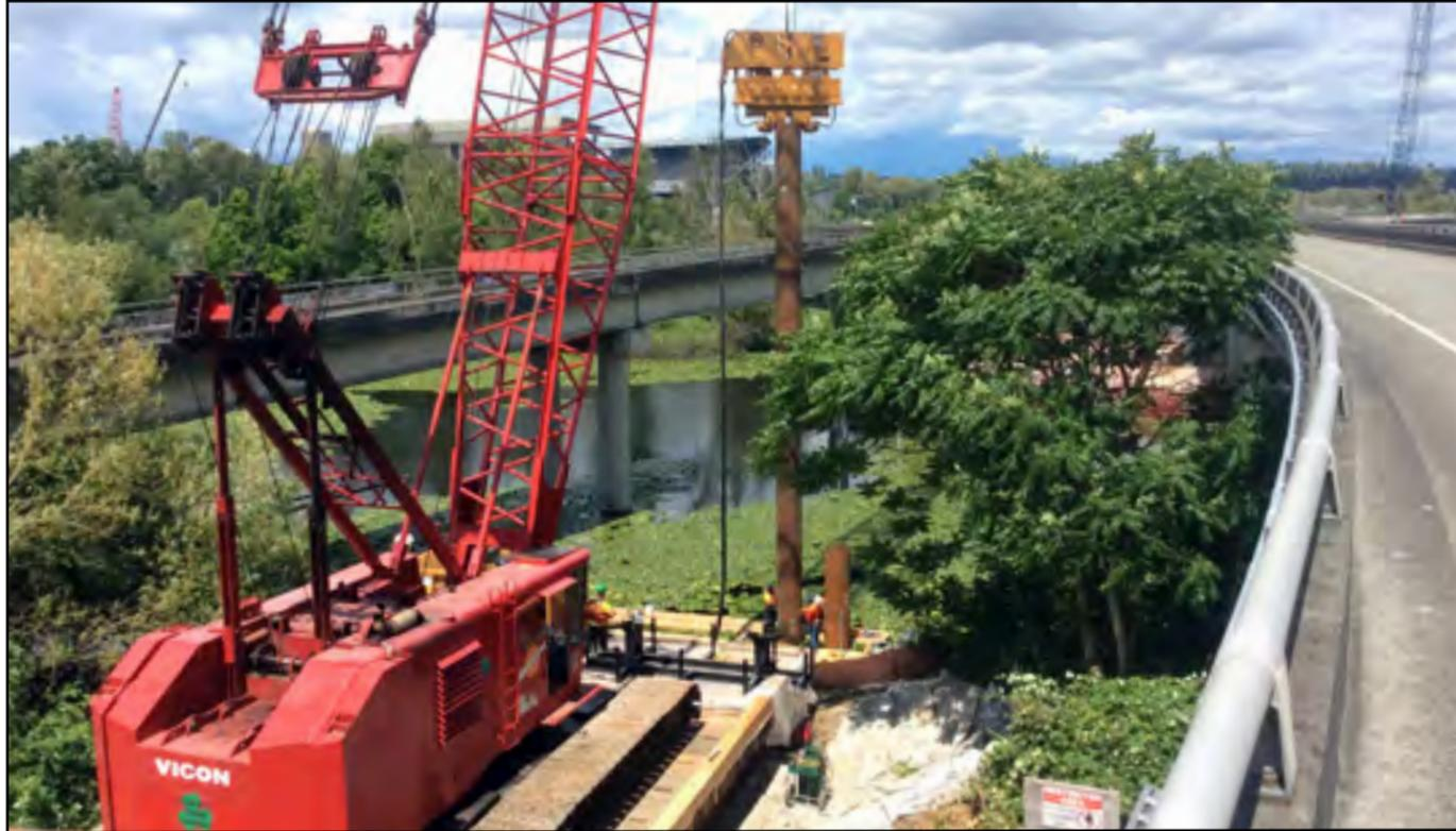
Crews install a pile for the temporary work bridge that will be used to off-load demolition debris of the westbound SR 520 off-ramp to Lake Washington Boulevard East and the R.H. Thomson "Ramps to Nowhere." Photo taken: June 14.
