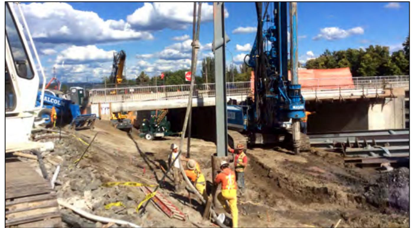
In order to prevent soils from encroaching onto the SR 520 mainline, crews install steel supports for a retaining wall that will extend from the 24th Avenue East overpass to Montlake Boulevard. Photo taken: June 16.
