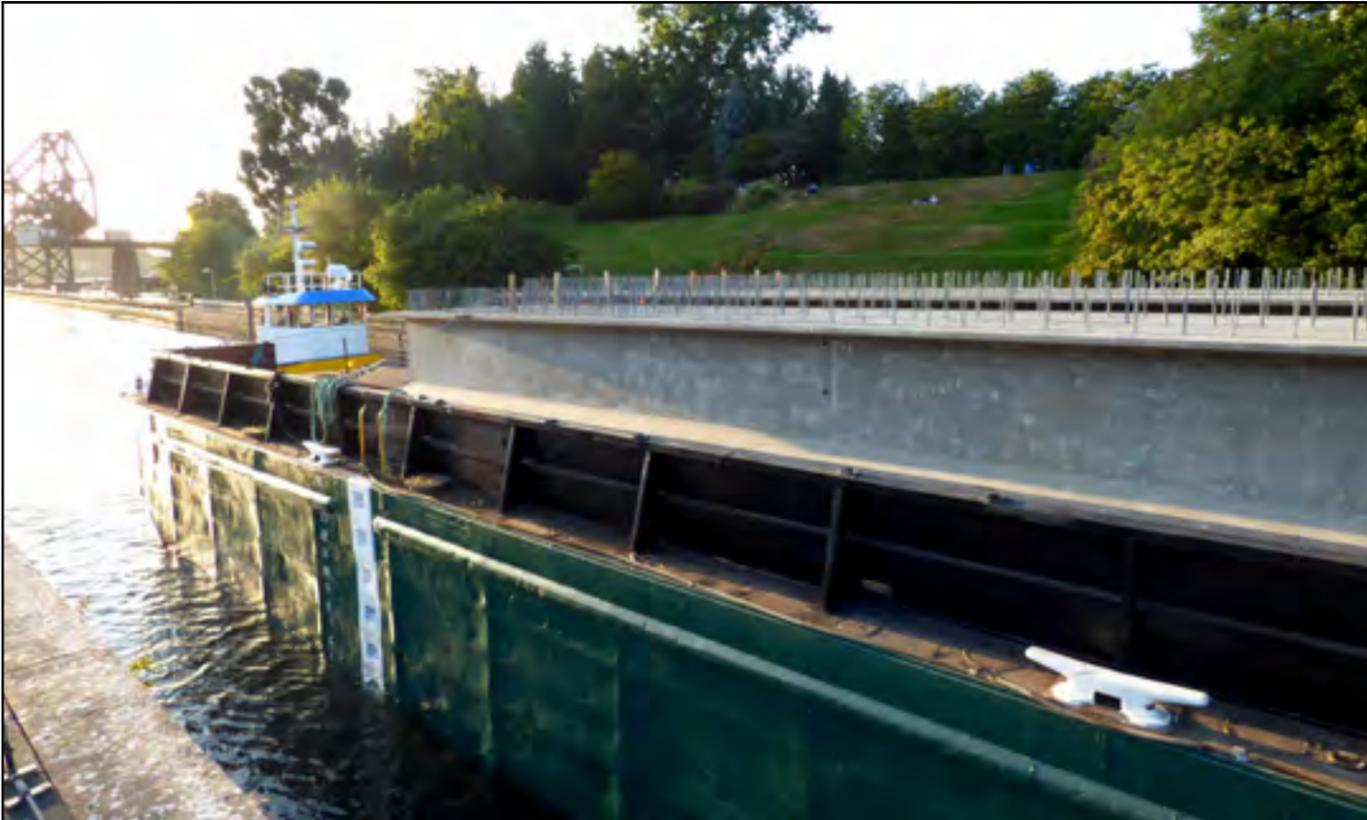
*A barge carrying 150-foot-long girders for the new west approach bridge eases through the Lake Washington ship canal. Each wide-flange girder weighs about 153,000 pounds. Photo taken: July 1*
