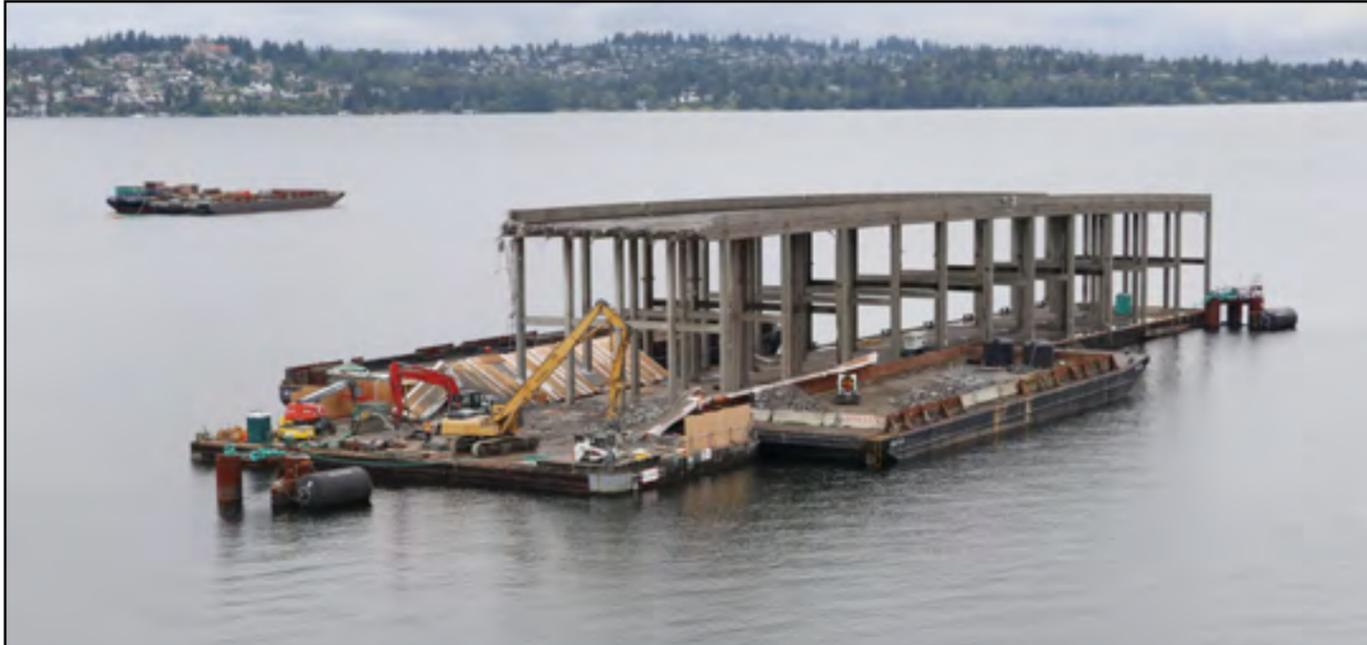
Pontoons A and B from the old floating bridge are anchored at the east side staging area for removal of their concrete columns and roadway deck. Photo taken: July 22
