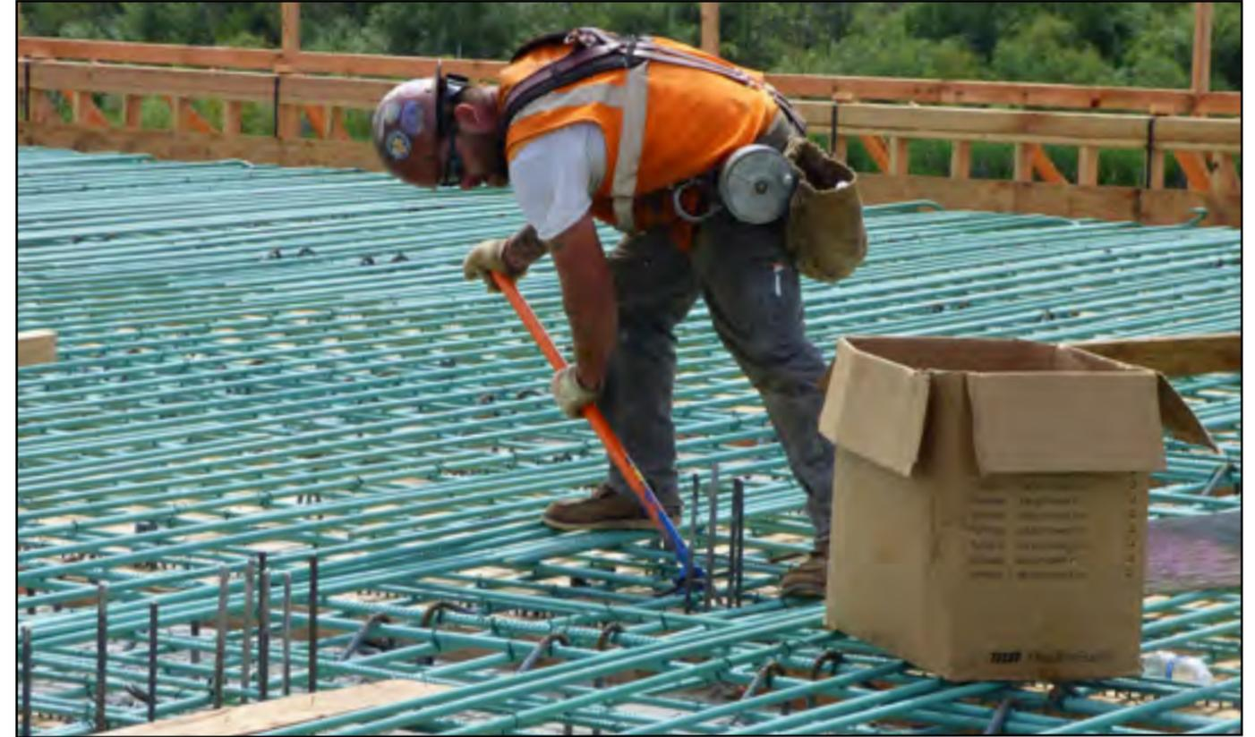
*A crew member fastens rebar together in preparation for pouring concrete for the permanent roadway deck. Photo taken: July 1*
