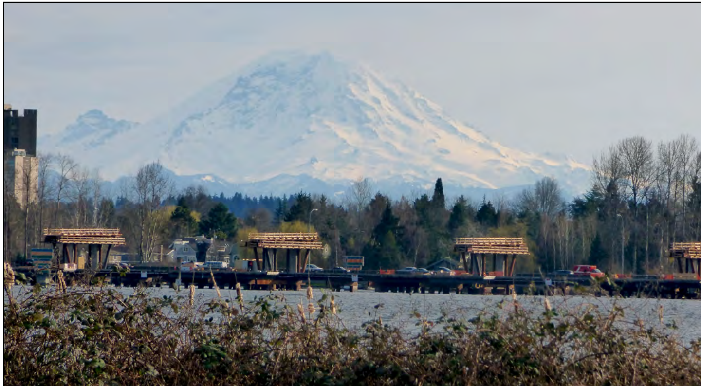
Throughout February, crews on the West Approach Bridge North Project erected falsework on columns to prepare for installation of isolation bearings and girders. Photo taken: Feb. 23
