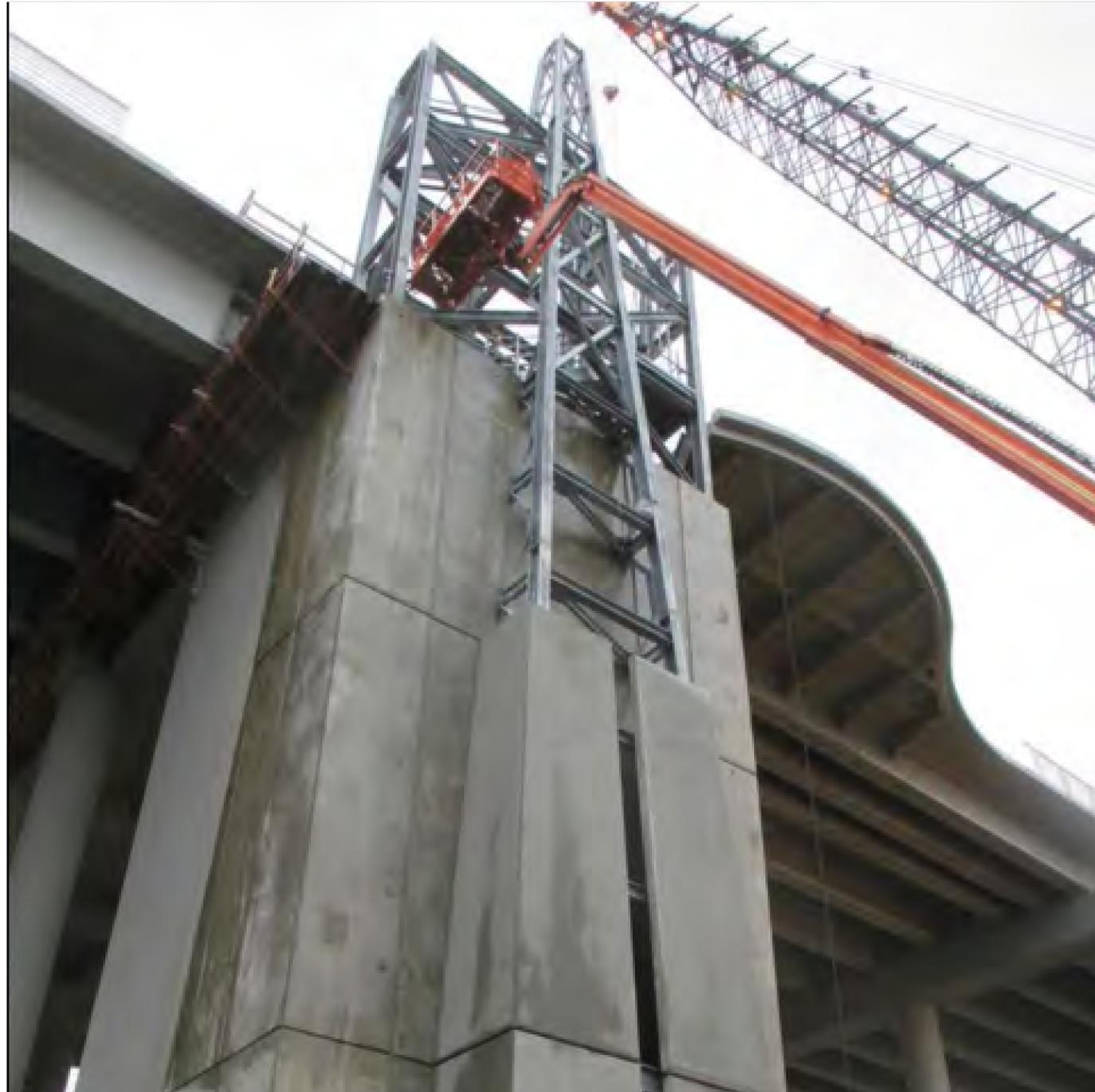
Crew members continue erecting the east high rise north sentinel. These structures will illuminate the navigational channels under the floating bridge. Photo taken: Dec. 28
