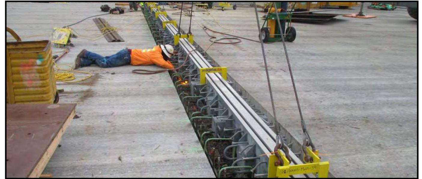
In December, construction crews continued installing the expansion joints that connect the east and west approaches to the floating section of the roadway deck. Photo taken: Dec. 22
