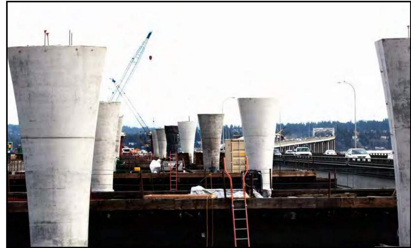
By the end of December, crews had installed 22 of the 95 concrete columns needed for the new West Approach Bridge North. Photo taken: Dec. 15
