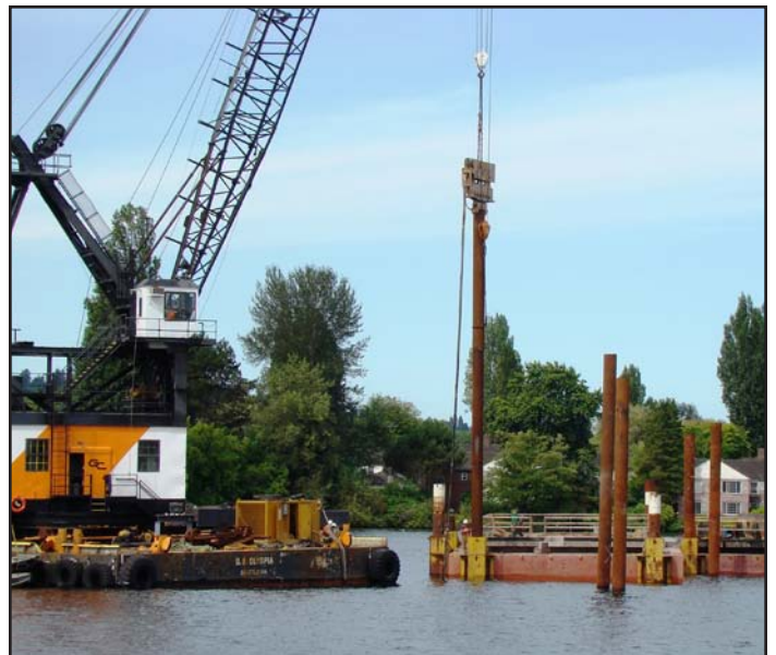
Shaft anchor installation takes place on Lake Washington near Madison Park.
