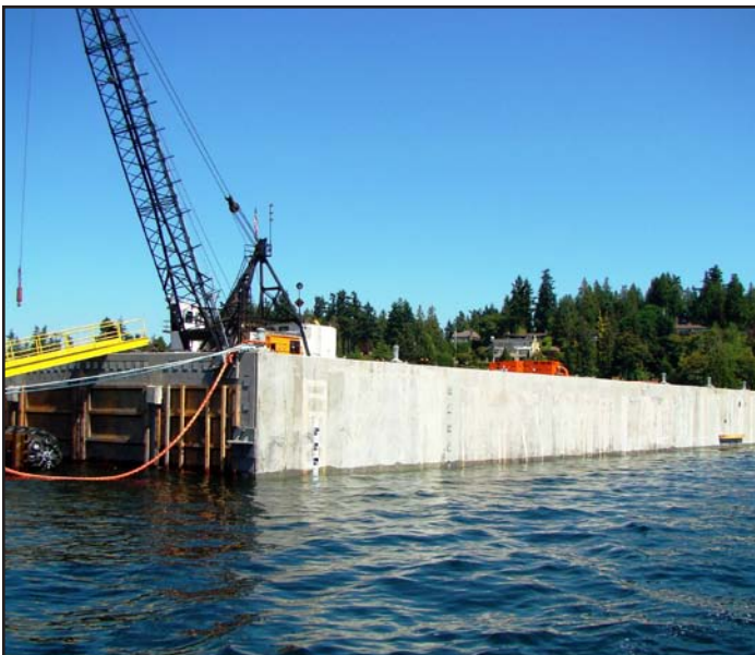
Pontoon V arrived on Lake Washington after a 260-mile journey from its casting basin in Aberdeen.
