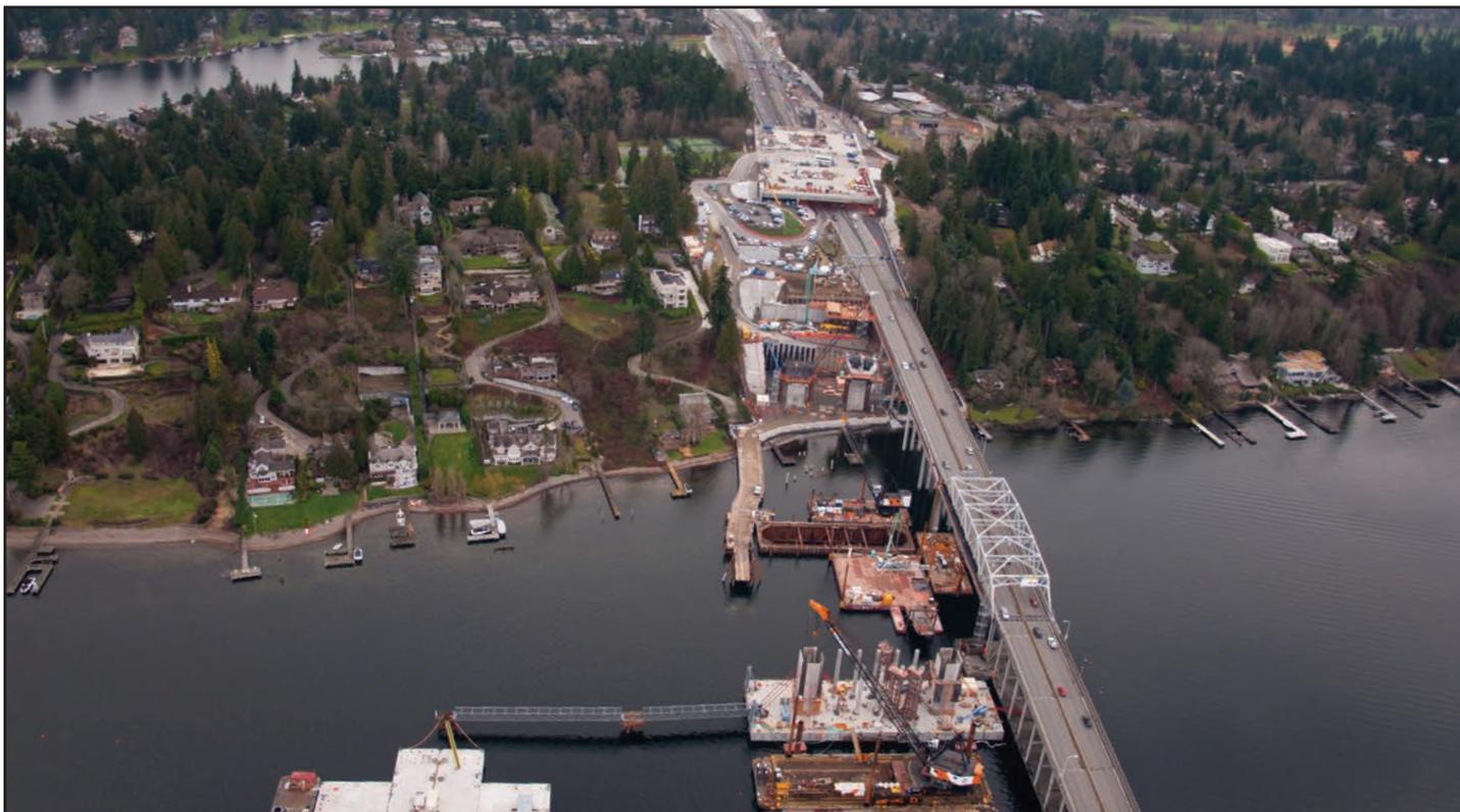
*Aerial view of the new SR 520 floating bridge taking shape on Lake Washington. Also pictured are the new east approach structure and Evergreen Point Road lid that are currently under way.*
