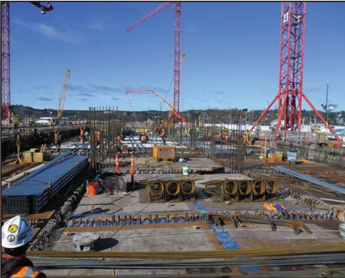
*Crews install new ducts on a longitudinal pontoon in Aberdeen, WA.*
