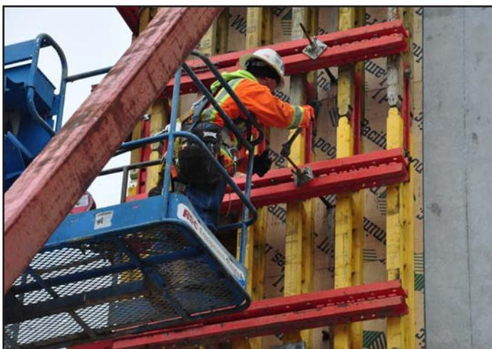
*A worker secures form work on a box column on pontoon W.*
