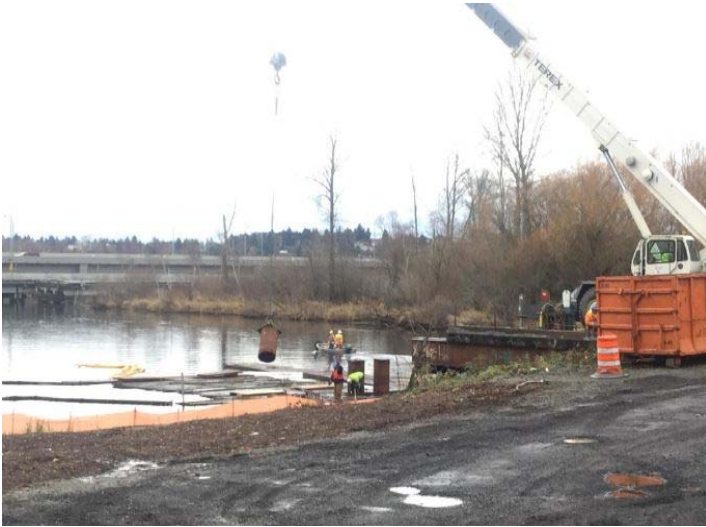
WABN: Removing cut pile from work trestle
