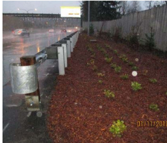
FB&L: Landscape restoration along new guard rail
