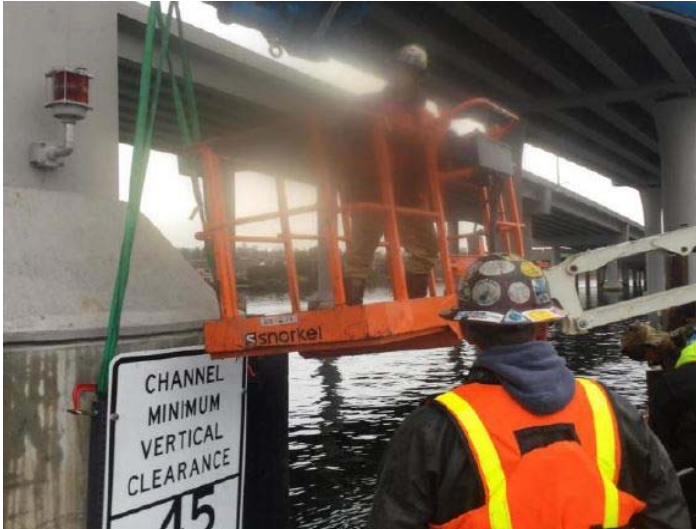
West Approach Bridge North (WABN): Installing clearance sign
