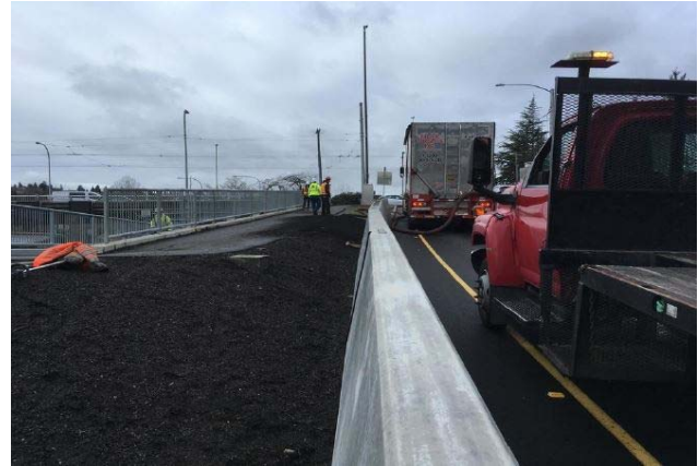
WABN: Preparing seeded lawn soil along alignment for bus path.
