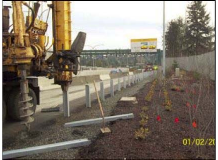
Floating Bridge and Landings (FB&L): Installing flared barrier guardrail
