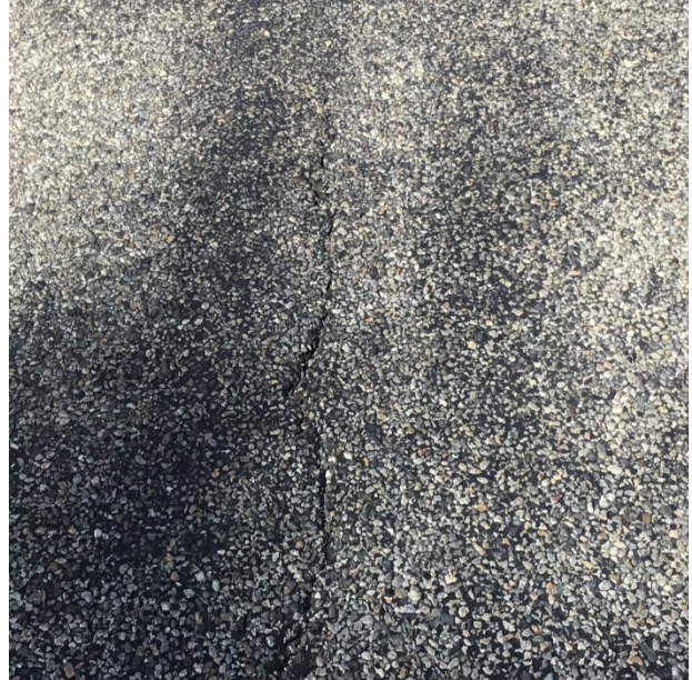
Figure 37. Longitudinal crack reflecting through the HBST at MP 4.00. (August 2017)
