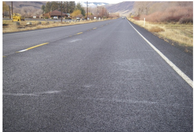
Figure 53. Streaks from underlying crack sealant in HBST at the age of six months. (Dec. 2015)
