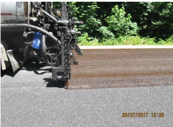
Figure 143. Fog sealing HBST. (July 2017)
