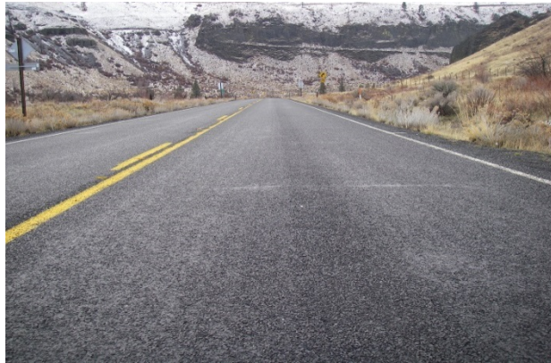
Figure 57. Streaking at the age of six months. (Dec. 2015)
