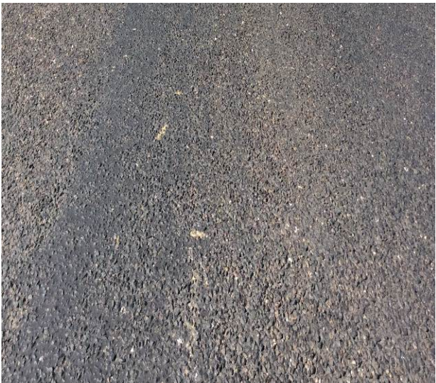
Figure 151. HBST at MP 4.41 with 70-80% embedment (100% in the wheel paths). (August 2017)
