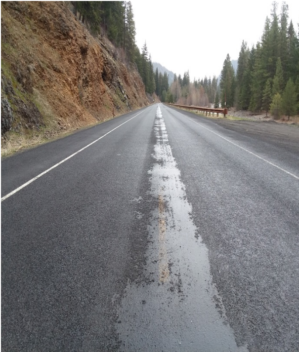
Figure 200. Centerline patch on SR-410. (April 2018)
