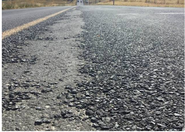
Figure 72. Snowplow damage at MP 5.39. (August 2017)
