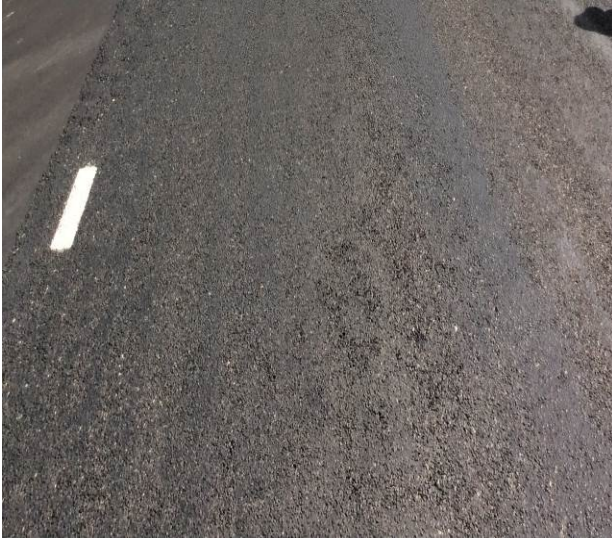
Figure 149. View at MP 4.41 with 70-80% embedment (100% in the wheel paths). (August 2017)
