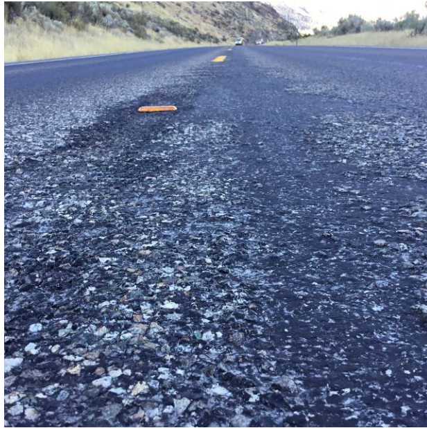
Figure 101. Snowplow damage at the centerline at MP 234.00. (August 2017)
