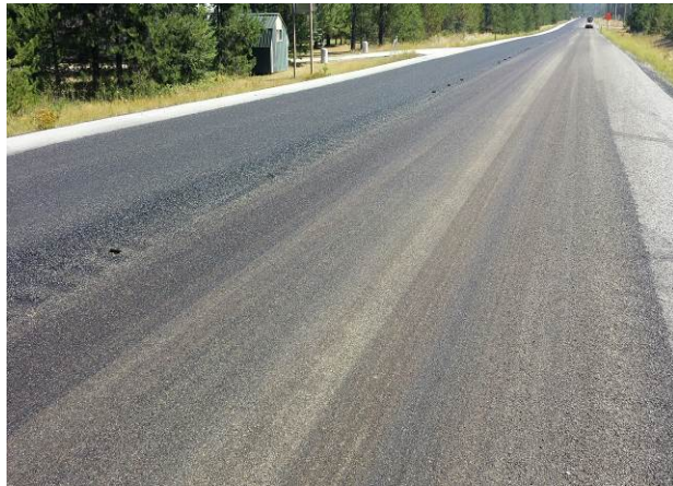
Figure 91. Choke stone on the HBST. (August 2016)
