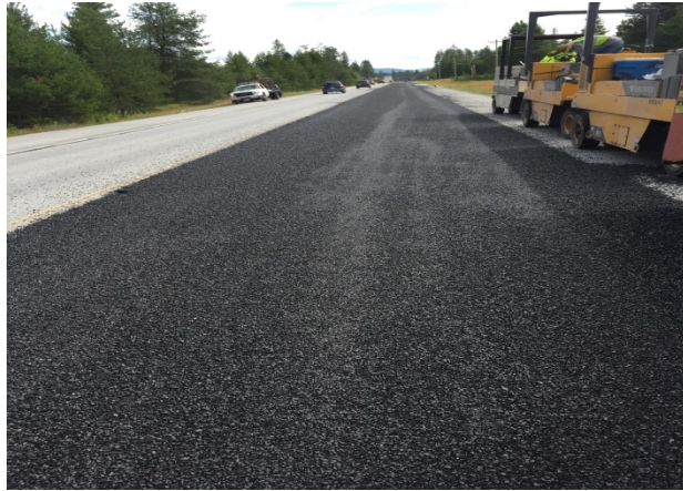
Figure 89. Chips prior to rolling. (August 2016)
