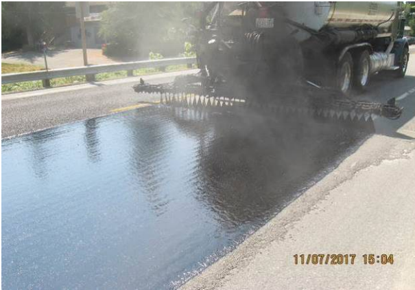
Figure 133. Distributor applying AC-15P. (July 2017)
