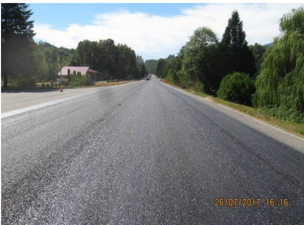
Figure 147. Completed HBST with choke. (July 2017)
