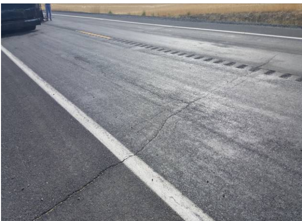
Figure 106. Transverse crack in US-2. (August 2016)
