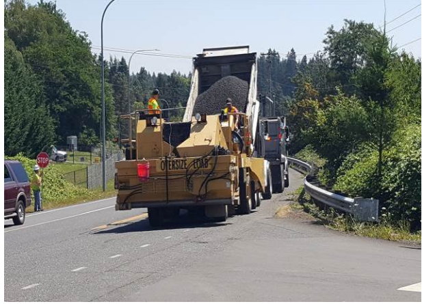
Figure 119. Chip spreader. (July 2016)
