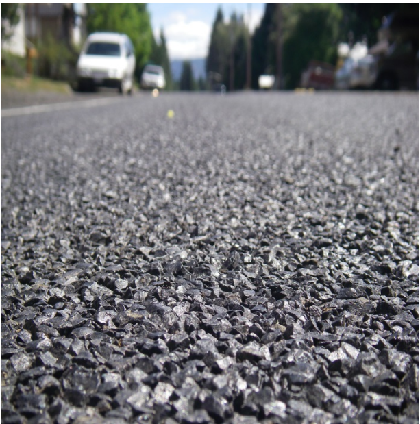
Figure 173. Close-up view at MP 7.30 showing 50% embedment. (Aug. 2017)
