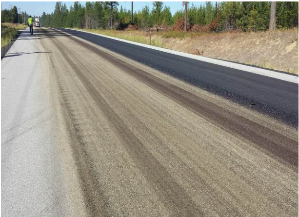
Figure 90. Choke stone on the HBST. (August 2016)
