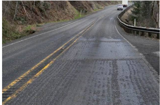
Figure 82. HBST showing aggregate loss. (Jan. 2016)
