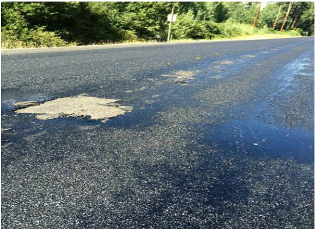
Figure 30. Delamination and flushing of the HBST. (July 2015)
