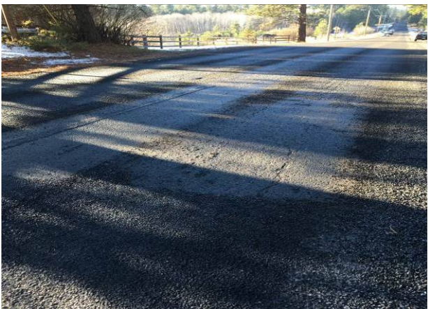
Figure 176. Raveling on the section between Roslyn and Ronald.
