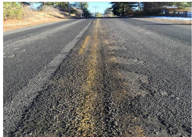
Figure 177. Raveling at MP 6.10 on the section between Roslyn and Ronald.
