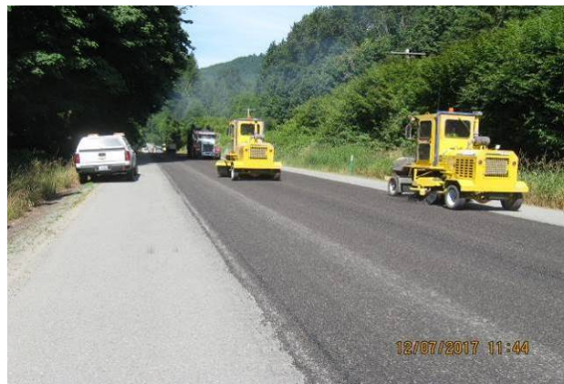
Figure 138. Sweepers removing excess aggregate from the HBST. (July 2017)
