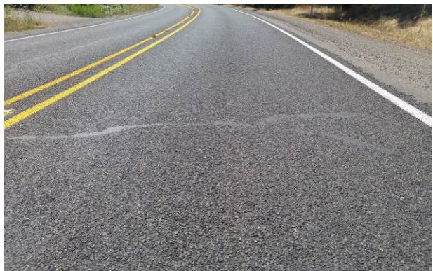
Figure 129. Shadows of crack sealant one month after paving. (August 2016)
