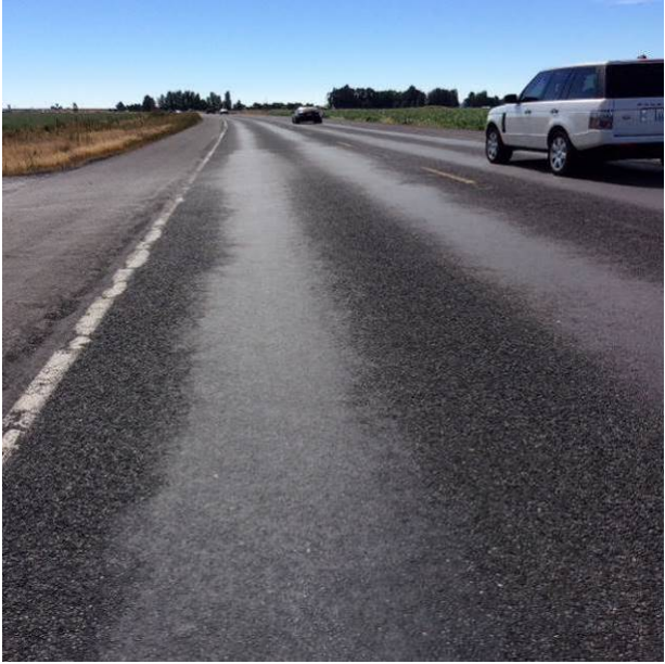
Figure 24. Looking north from MP 3.35 showing 100% embedment in the wheel paths. (August 2017)
