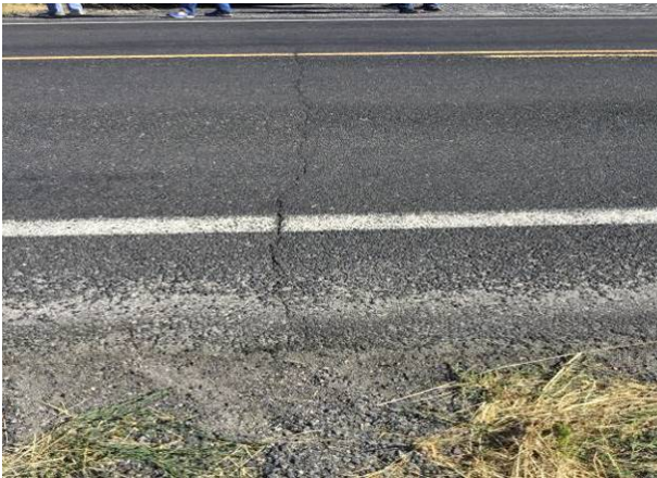
Figure 69. Transverse crack at MP 5.39. (August 2017)
