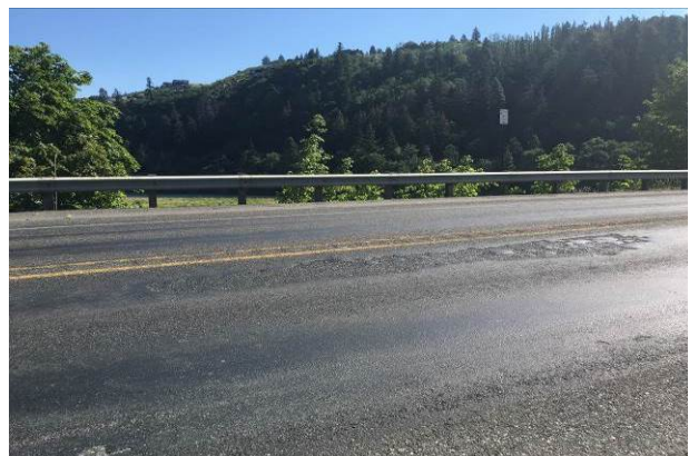
Figure 84. Delamination of HBST. (June 2016)
