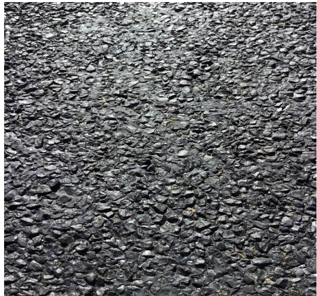
Figure 184. Close-up at MP 69.44 showing spots where the embedment is 60-70%. (August 2017)
