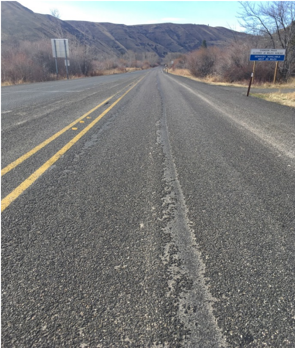
Figure 192. Raveling at MP 116.36. (February 2018)
