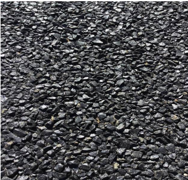
Figure 183. Close-up at MP 69.44 showing 30% embedment. (Aug. 2017)
