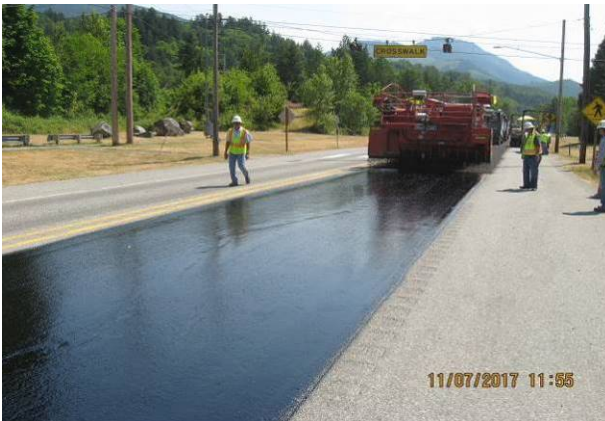
Figure 135. Chip spreader dropping 3/8" to No. 8 aggregate onto the AC-15P. (July 2017)
