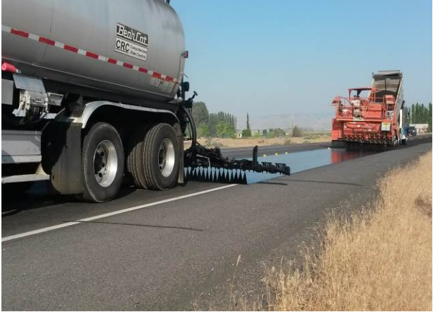
Figure 13. Distributor and chip spreader. (July 2015)
