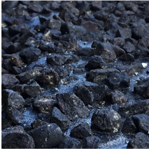
Figure 166. Close-up view of the 50% chip embedment at MP 91.38. (August 2017)
