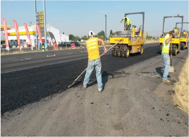
Figure 15. Pneumatic roller. (July 2015)
