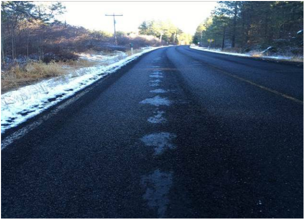
Figure 178. Raveling at MP 8.00 on the section between Ronald and National Forest Boundary.
