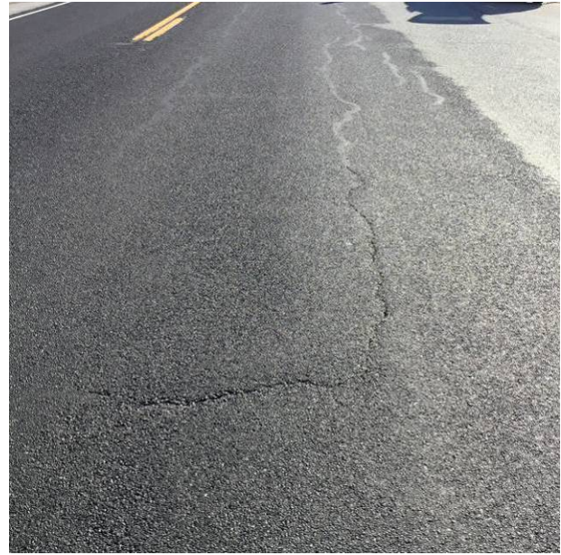
Figure 4. Longitudinal crack extending from crack that was sealed prior to the HBST at MP 223.76. (August 2017)
