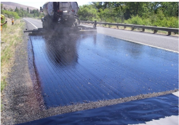
Figure 38. AC-15P binder applied to roadway. (June 2015)
