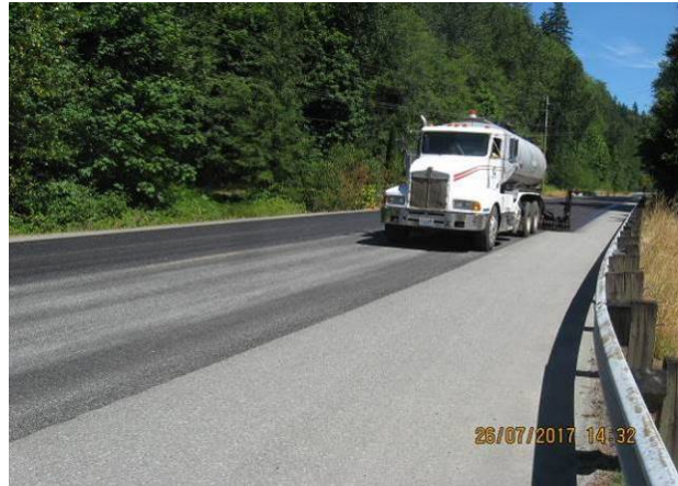
Figure 146. Fog sealed choke. (July 2017)
