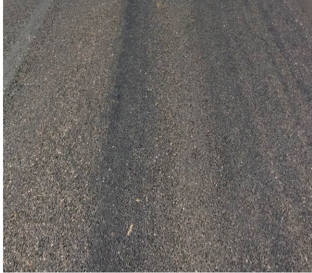
Figure 150. Another view at MP 4.41 with 70-80% embedment (100% in the wheel paths). (August 2017)
