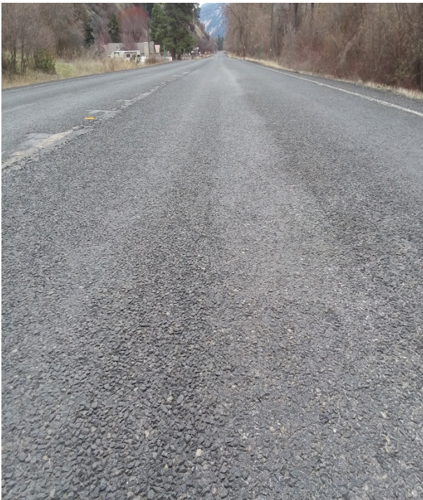
Figure 202. Typical good embedment on SR-410. (April 2018)
