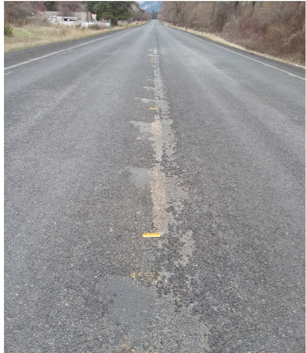
Figure 201. Typical distress on SR-410 (streaks or show plow damage). (April 2018)
