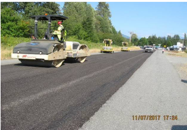
Figure 137. Steel wheel roller which followed the three pneumatic rollers setting the chips. (July 2017)
