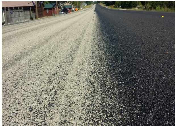
Figure 93. Choke stone on the HBST. (August 2016)
