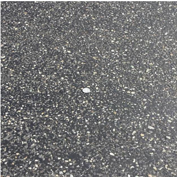
Figure 65. HBST at MP 319.70 with 100% embedment. (August 2017)
