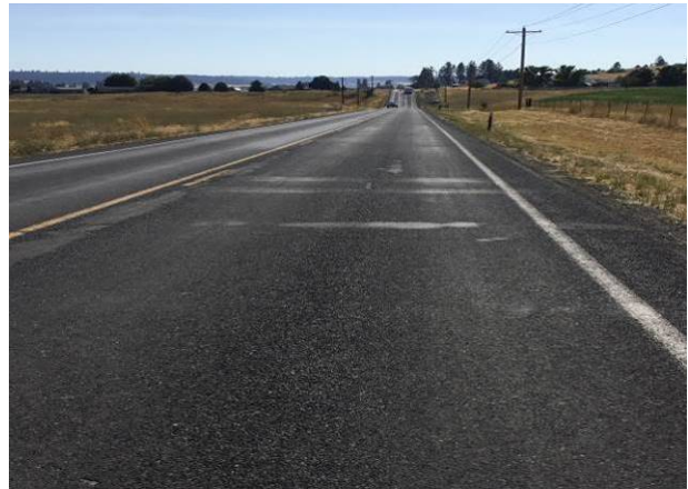
Figure 70. Transverse streaking at MP 5.39. (August 2017)
