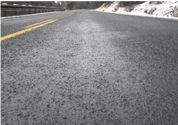
Figure 52. HBST with 100% embedment at the age of six months. (Dec. 2015)
