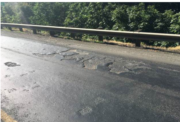
Figure 83. Delamination of HBST. (June 2016)
