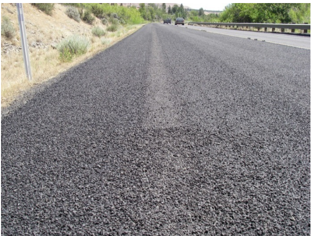
Figure 44. HBST prior to sweeping. (June 2015)
