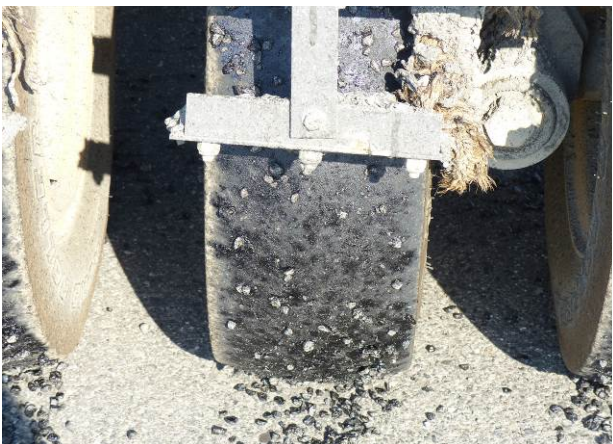
Figure 17. Aggregate and binder sticking to pneumatic roller tire. (July 2015)
