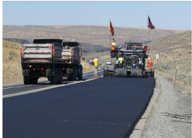
Figure 111. Pre-level paving over the cushion course. (August 2016)
