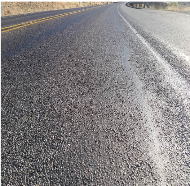
Figure 96. Closer view of HBST at MP 321.85 showing 100% embedment in the wheel paths and 60% between wheel paths. (August 2017)
