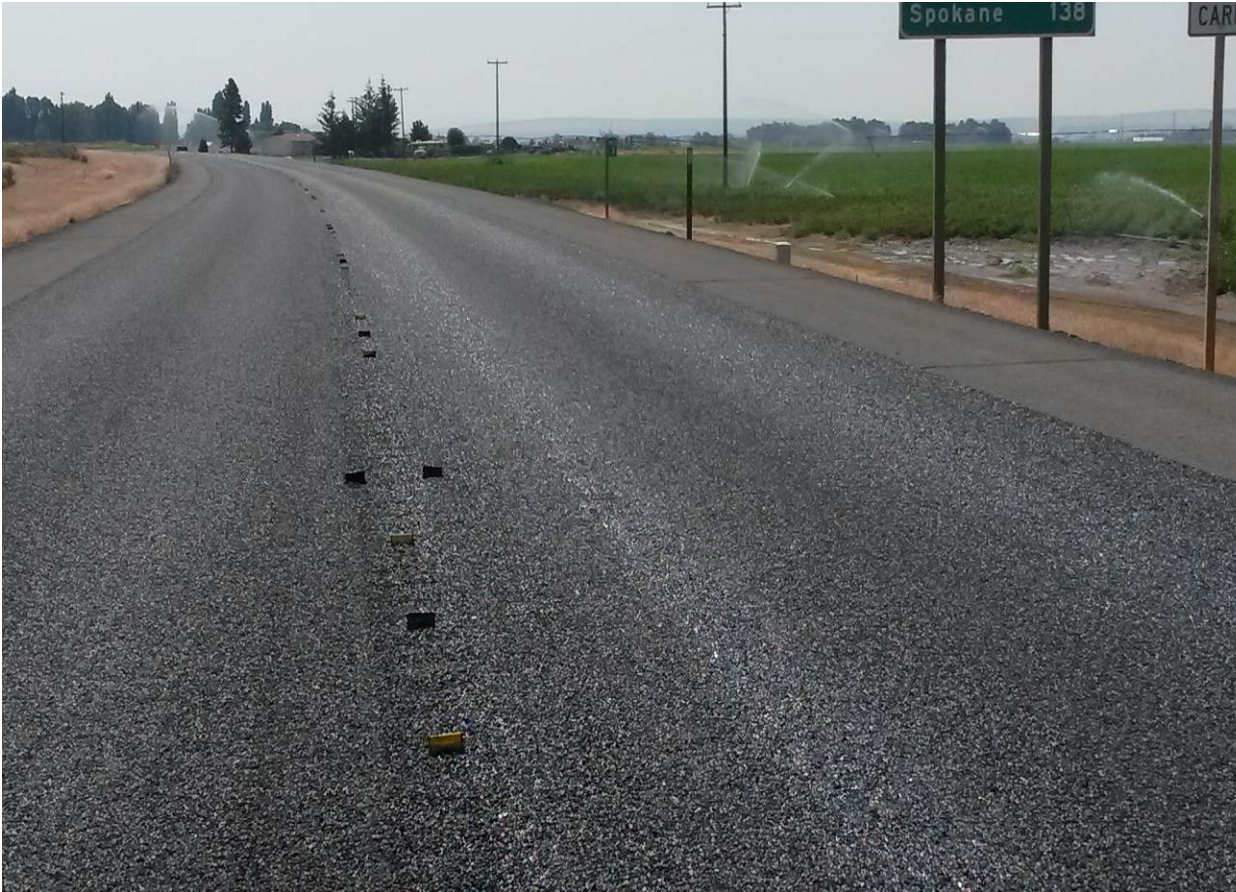
Figure 23. Both lanes of the completed HBST on SR 281 Spur showing 100% embedment in the wheel paths. (July 2015)
