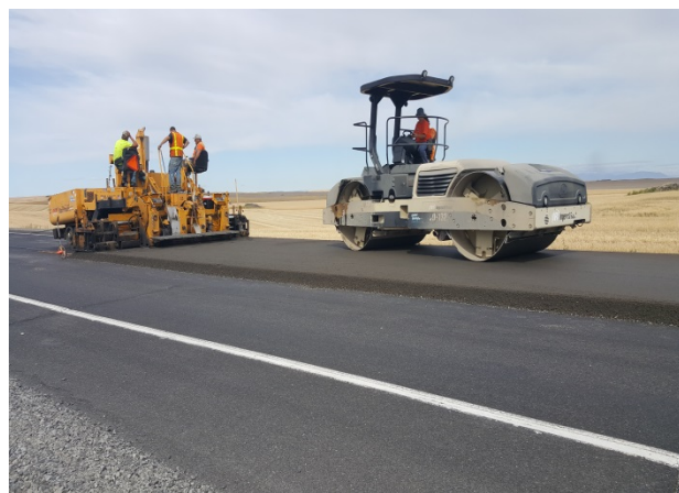
Figure 107. Spreading and compacting cushion course on US-2. (August 2016)
