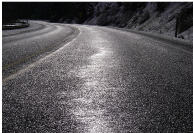
Figure 59. Rich appearing wheel paths at the age of six months. (Dec. 2015)
