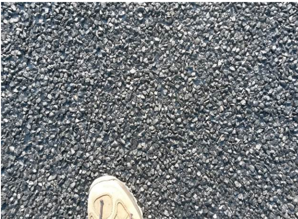
Figure 21. Closer view of HBST. (July 2015)
