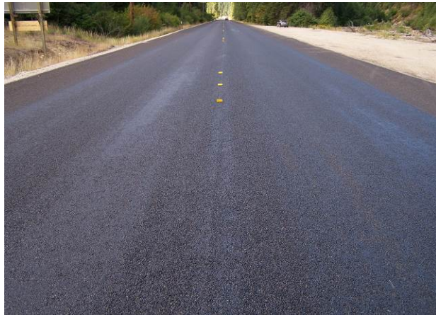
Figure 31. Fog seal applied to HBST after repairs were made. (July 2015)
