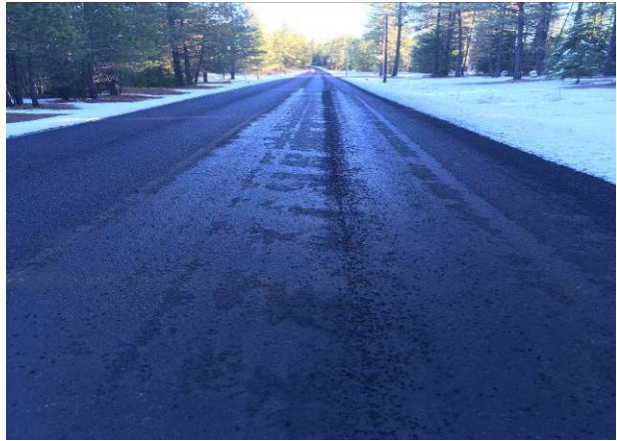
Figure 179. Raveling at MP 9.00 on the section between Ronald and National Forest Boundary.
