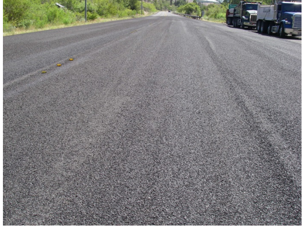
Figure 47. Finished HBST. (June 2015)
