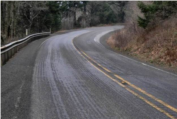
Figure 81. HBST showing aggregate loss. (Jan. 2016)
