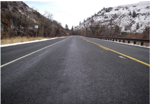
Figure 58. Rich appearing wheel paths at the age of six months. (Dec. 2015)
