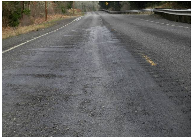
Figure 78. HBST showing aggregate loss. (Jan. 2016)
