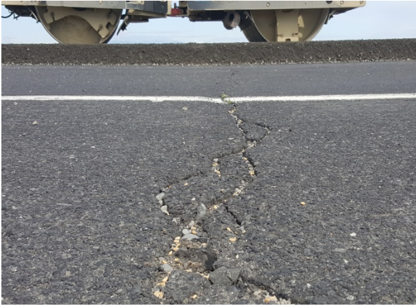
Figure 108. Rolling of cushion course on US-2 over transverse crack. (August 2016)
