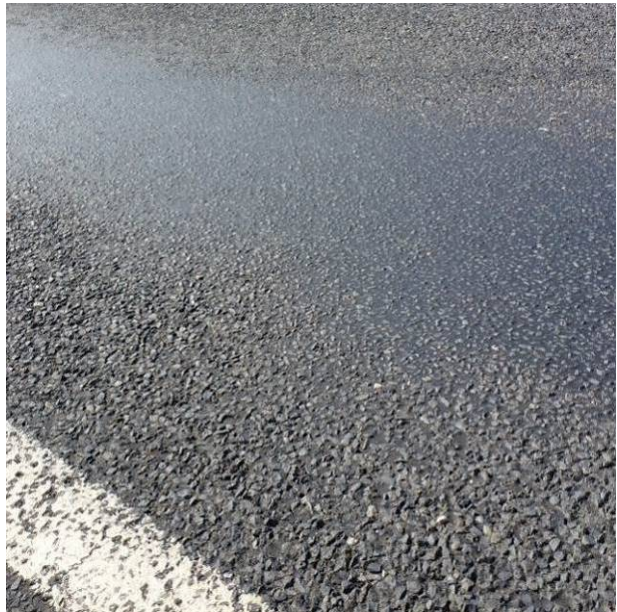
Figure 27. Close-up of the wheel path with 100% embedment at MP 3.35. (August 2017)
