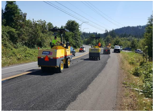
Figure 121. Pneumatic rollers. (July 2016)
