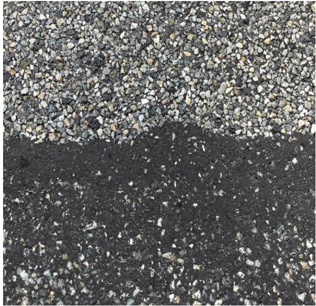
Figure 33. HBST and slurry seal contact at MP 4.00. (August 2017)
