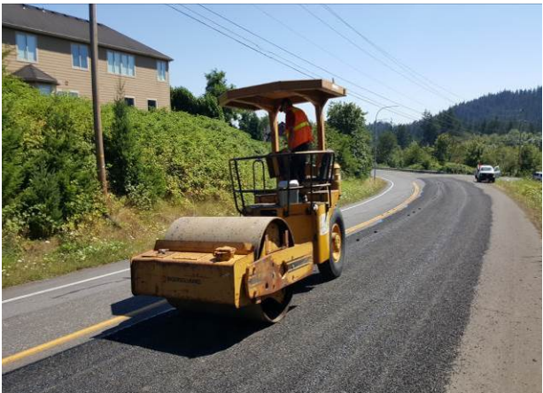
Figure 122. Steel wheel roller. (July 2016)
