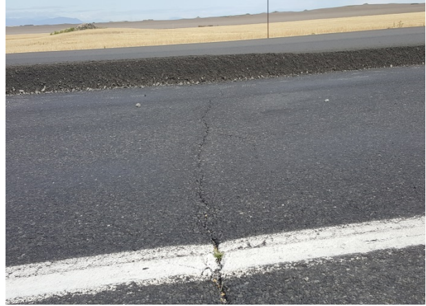
Figure 109. Rolling of cushion course on US-2 over transverse crack. (August 2016)
