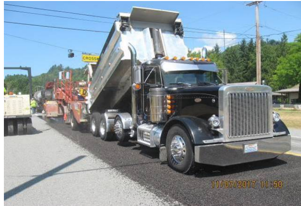
Figure 134. Truck delivering aggregate to spreader. (July 2017)
