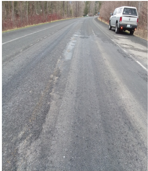
Figure 203. Isolated area of complete aggregate shedding. (April 2018).
