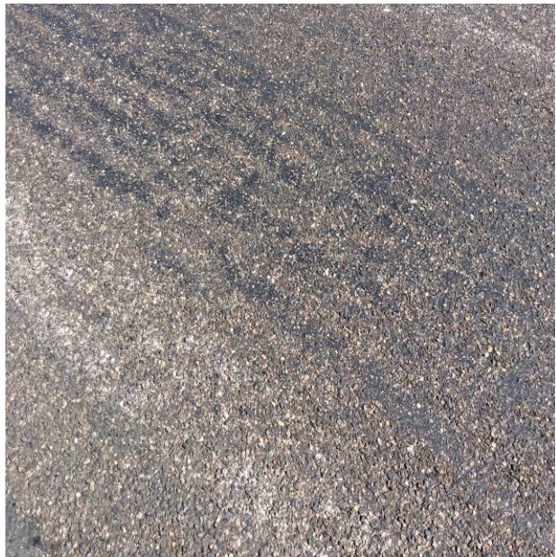
Figure 170. Close-up of the cornrows at MP 18.30. (August 2017)
