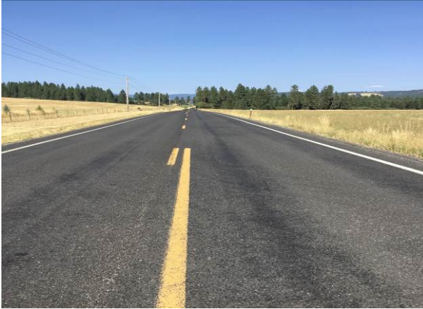
Figure 67. HBST at MP 5.39 on with 100% embedment in the wheel paths. (August 2017).
