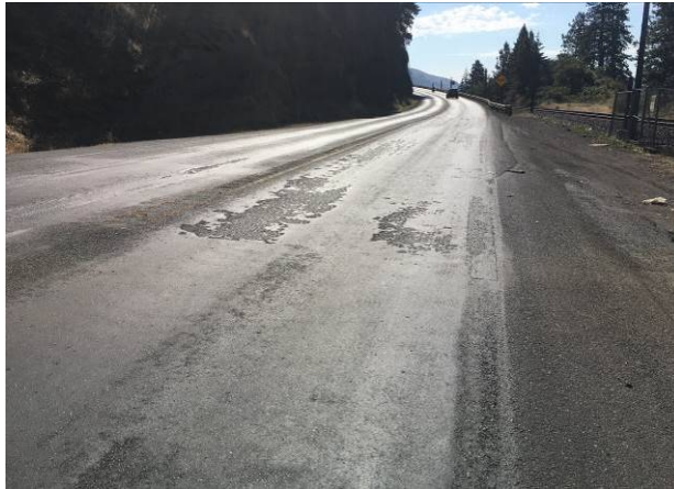
Figure 85. Delamination of HBST. (June 2016)
