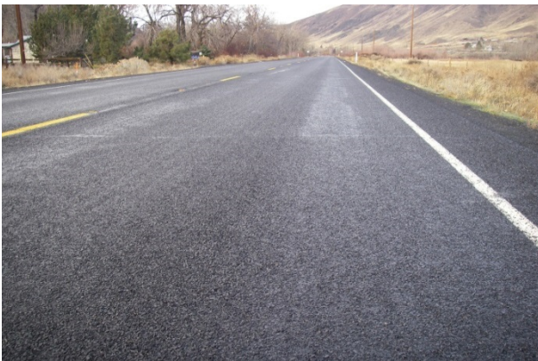
Figure 54. Rich areas in the wheel paths at the age of six months. (Dec. 2015)
