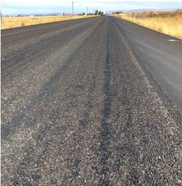
Figure 161. Looking south from MP 3.55 showing streaky appearance (cornrows). Embedment is 70-80%. (August 2017)
