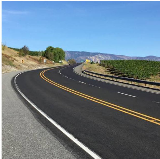
Figure 10. HBST with 100% embedment in the wheel paths at MP 230.20. (August 2017)
