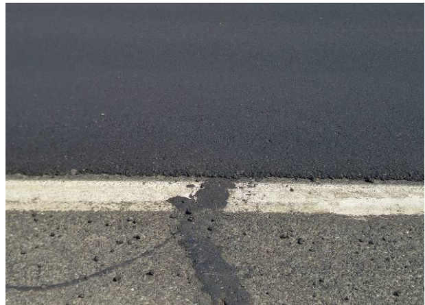
Figure 113. Pre-level on US-2 with over sealed transverse crack. (August 2016)
