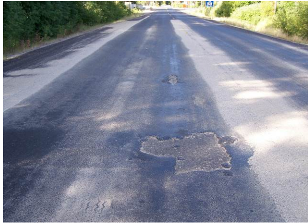
Figure 29. Delamination of HBST. (July 2015)
