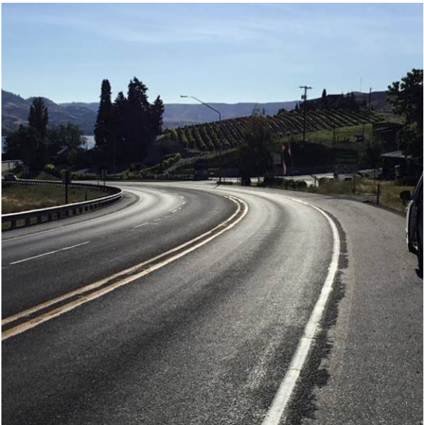
Figure 9. HBST with 100% embedment in the wheel paths at MP 230.20. (August 2017)
