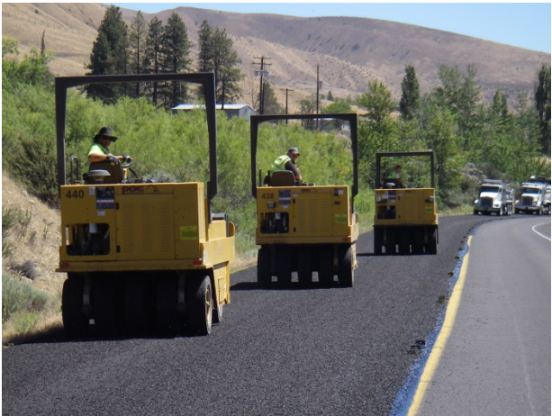
Figure 42. Three pneumatic rollers seating chips. (June 2015)
