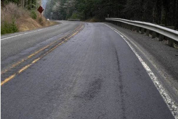
Figure 79. HBST showing aggregate loss. (Jan. 2016)
