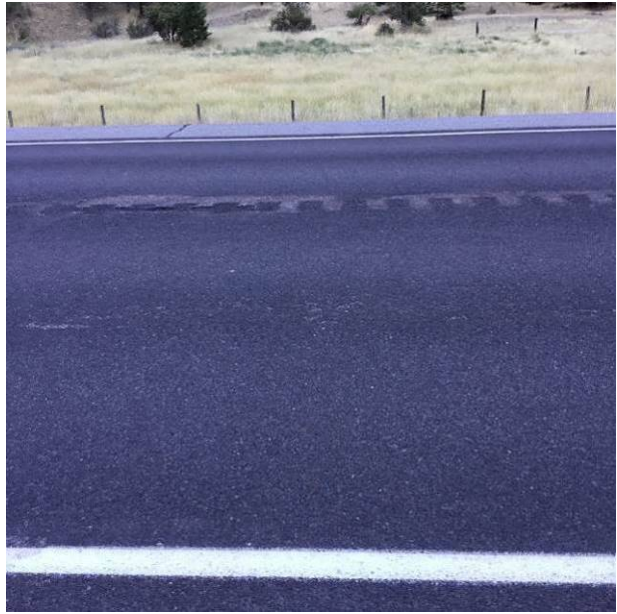
Figure 8. Snowplow damage at MP 227.50. (August 2017)
