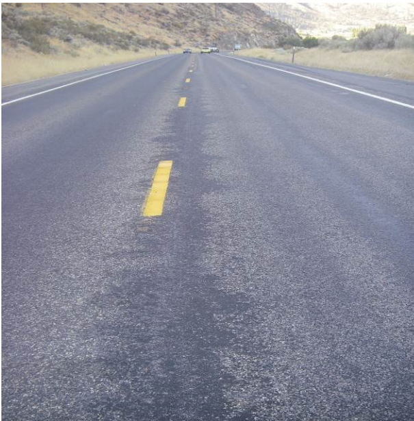
Figure 98. Looking north from MP 234.00 showing snowplow damage at the centerline and 100% embedment in the wheel paths. (August 2017)
