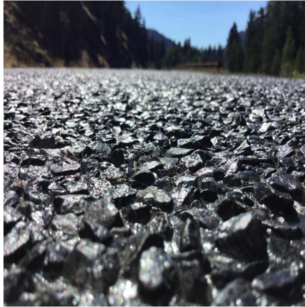
Figure 191. Road level view at MP 94.30 showing 30% embedment. (Aug. 2017)
