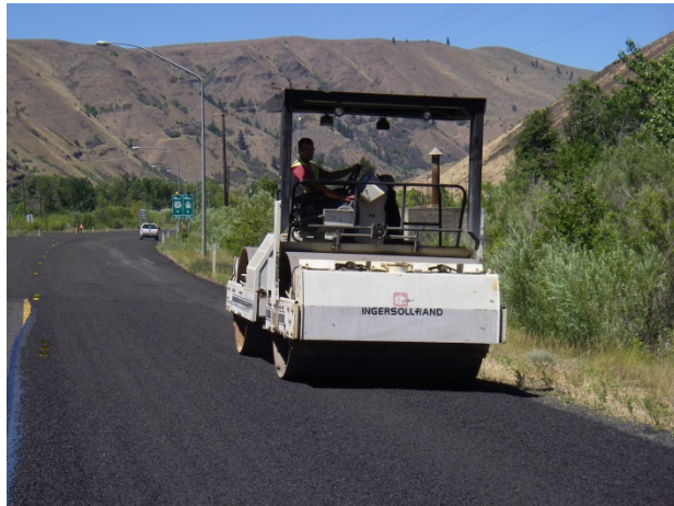
Figure 43. Steel wheel roller doing final rolling. (June 2015)
