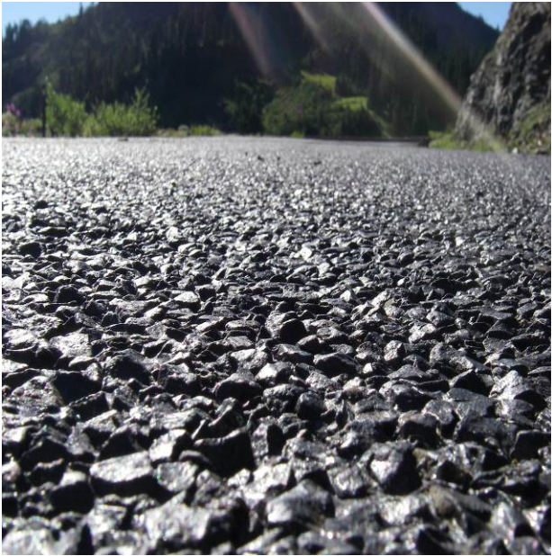
Figure 185. Road level view at MP 69.44 showing lack of embedment. (August 2017)
