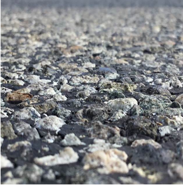
Figure 36. Low level view at MP 4.00 showing 60% embedment. (August 2017)
