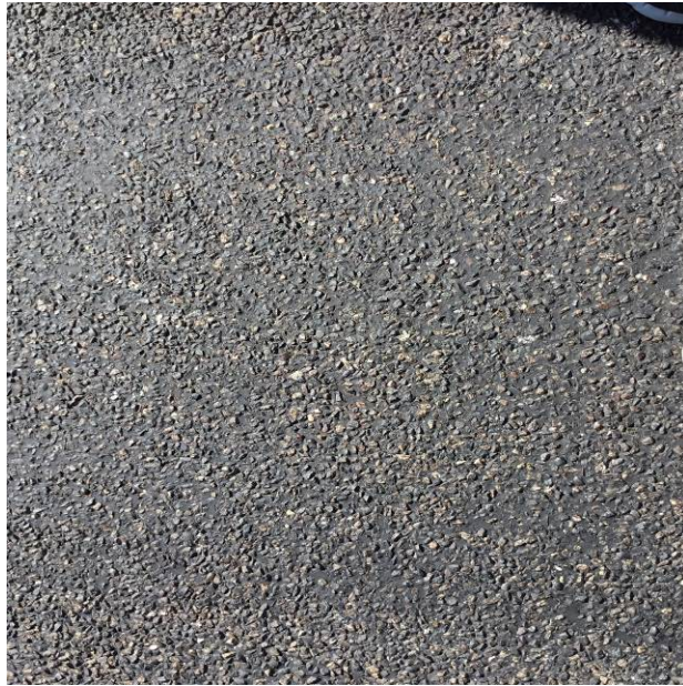
Figure 158. Close-up view at MP 8.00 with 60-90% embedment. (Aug. 2017)
