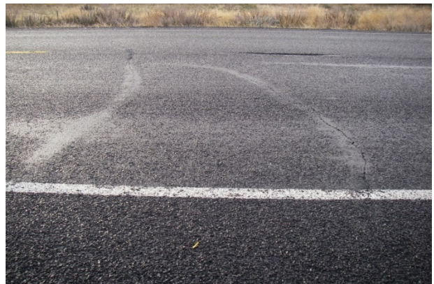
Figure 55. Transverse cracking at the age of six months. (Dec. 2015)
