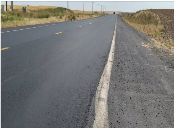
Figure 112. Pre-level on US-2. (August 2016)
