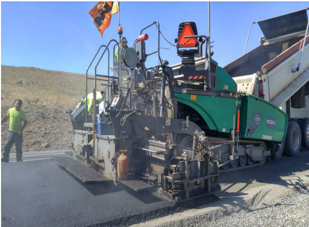
Figure 110. Pre-level paving over the cushion course. (August 2016)
