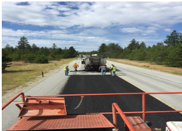
Figure 87. Another view from chip spreader of the distributor. (August 2016)
