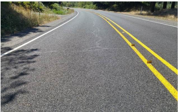
Figure 128. Shadows of crack sealant one month after paving. (August 2016)
