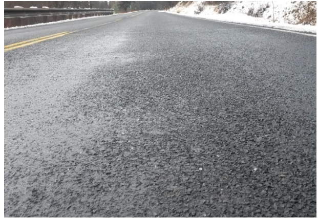
Figure 51. HBST with 100% embedment at the age of six months. (Dec. 2015)
