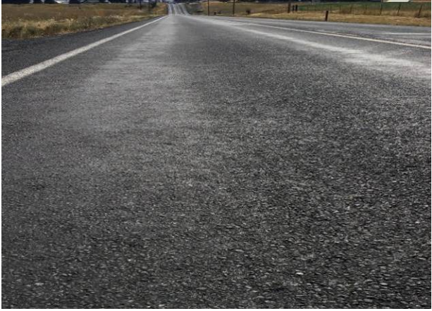
Figure 71. Rich appearance of HBST at MP 5.39 with 100% embedment in the wheel paths. (August 2017)
