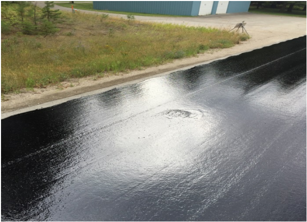
Figure 88. AC-15P binder on the roadway. (August 2016)
