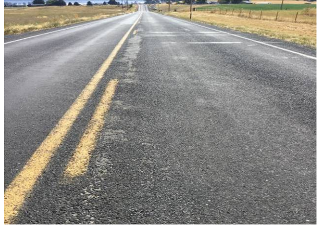
Figure 68. Centerline snowplow damage on HBST at MP 5.39. (August 2017).
