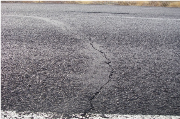
Figure 56. Transverse cracking at the age of six months. (Dec. 2015)
