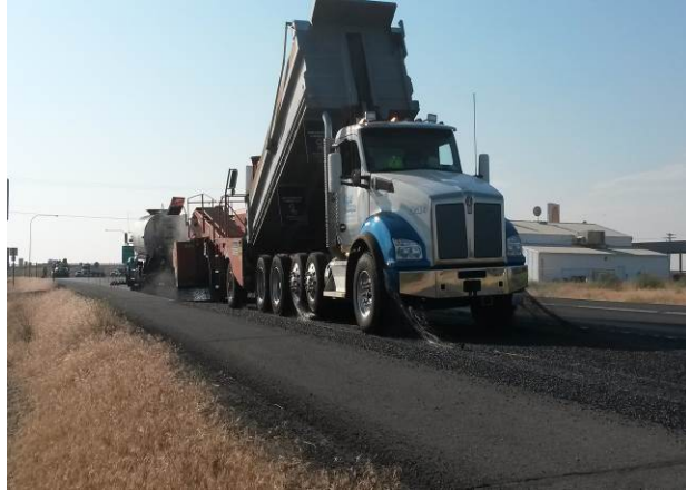
Figure 14. Truck dumping pre-coated chips into the spreader. (July 2015)
