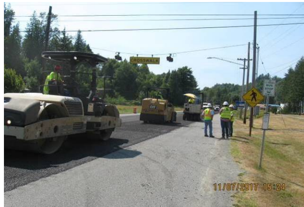
Figure 136. Three pneumatic rollers setting the chips. (July 2017)
