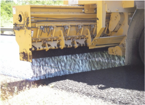
Figure 40. Curtain of chips falling onto binder. (June 2015)
