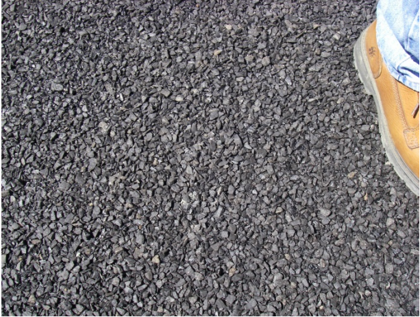
Figure 46. Finished HBST. (June 2015)
