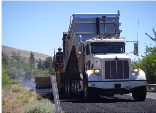
Figure 41. Truck delivering pre-coated chips. (June 2015)
