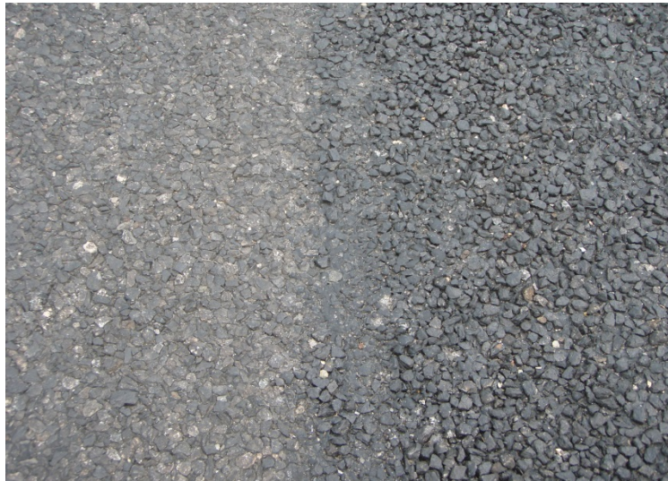
Figure 60. Choked (left) and un-choked (right) HBST. (Sept. 2015)
