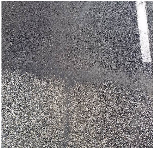
Figure 97. HBST at the top and conventional BST at the bottom at MP 321.85. (August 2017)
