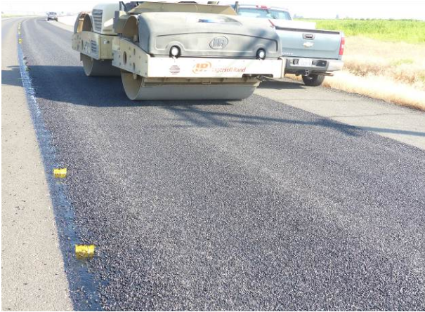
Figure 19. Steel wheel roller. (July 2015)
