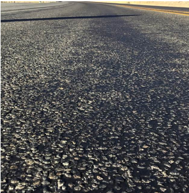
Figure 104. HBST at MP 205.09 showing 100% embedment in the wheel paths. (August 2017)
