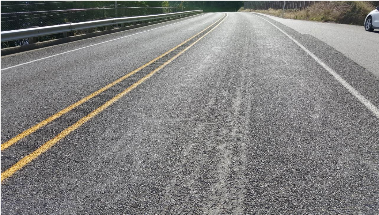
Figure 53. OR1a, SR101, three years after installation. Very slight flushing and shadowing of the sealed cracks.
