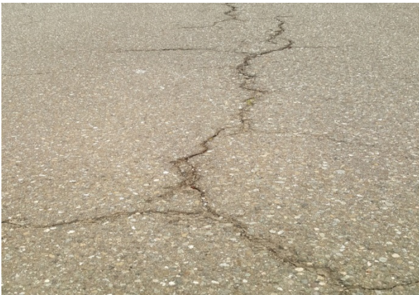
Figure 125. OR3a, SR101, Poor category, age 62 months. No maintenance as of the 2017 inspection.
