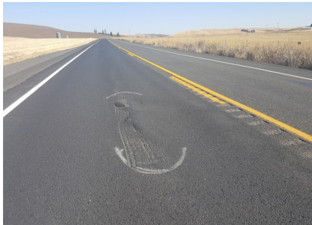
Figure 115. ER26, SR127, Good, age 26 months. Pot hole formed in 2016. Flushing in wheel paths noted in 2017.
