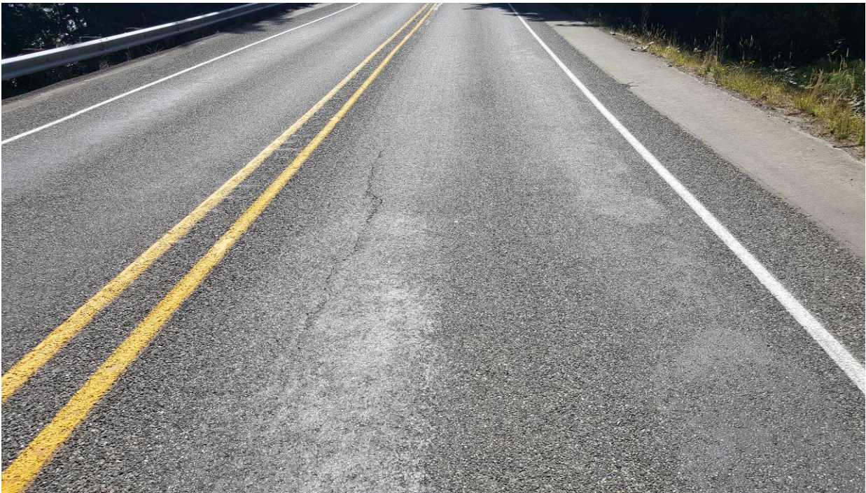
Figure 29. OR1b, SR101, five years after installation. Longitudinal crack condition is about the same, slight rutting and flushing in the wheel paths.
