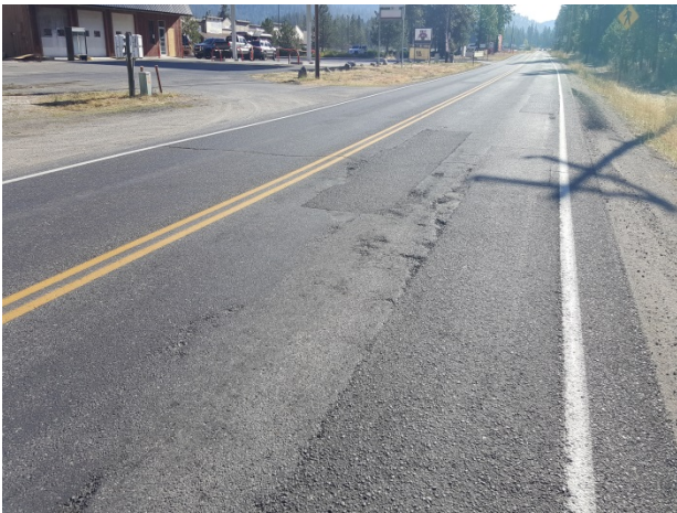
Figure 58. ER3, SR291, Fair, age 62 months. Additional dig outs added in 2015. Transverse reflection crack noted at 10 months after treatment. More dig outs are scheduled for installation in 2017 and a HMA grind/inlay in 2018, C9223.
