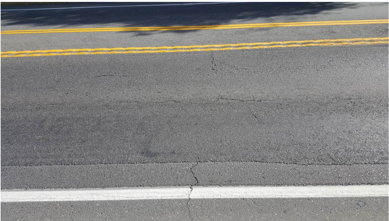
Figure 37. OR12, SR20, four years after installation. Some loss of aggregate and lots of reflection cracking through the wheel path chip seal.
