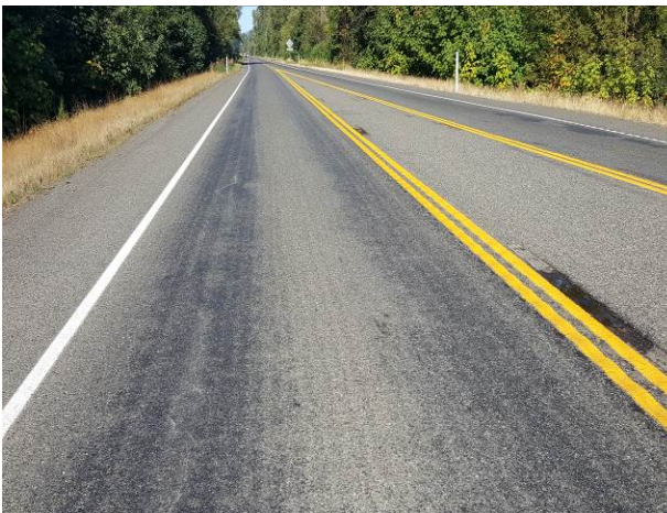
Figure 22. OR16, SR16, Good, age 49 months. Longitudinal cracking and pumping of fines noted at 14 months. Alligator cracking noted at 49 months.
