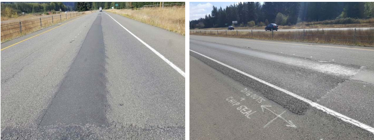
Figure 136. OR2 and OR2a on SR8. OR2 received dig outs and OR2a received dig outs and a chip seal. Photos are from 2016, both sections were milled and filled with HMA in 2017
