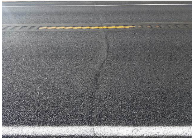
Figure 49. NC1, SR155, Good, age 38 months. Transverse crack locations are depressed and very thin cracks are present.
