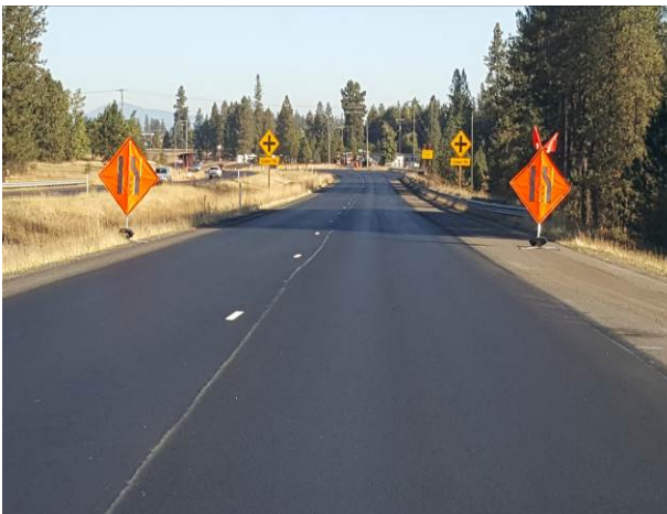
Figure 90. ER1, US2, Poor, 62 months. Additional dig outs and crack sealing done in 2015. HMA grind/inlay in 2017, C9124.
