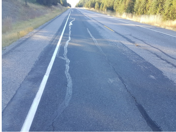
Figure 113. ER9a, SR395, Good, age 37 months. Transverse and longitudinal cracking reflecting through the patch at 13 months.
