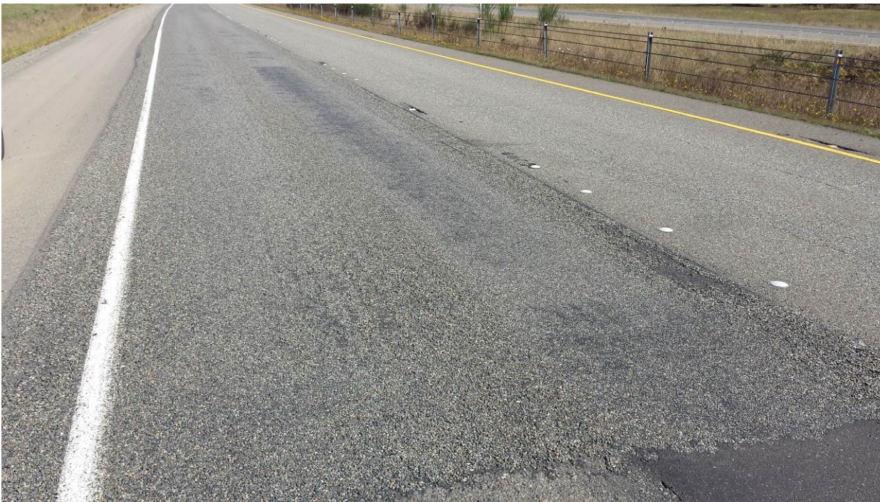
Figure 108. OR2a, SR8, two years after installation. Increased flushing in the wheel paths over the dig out patches.
