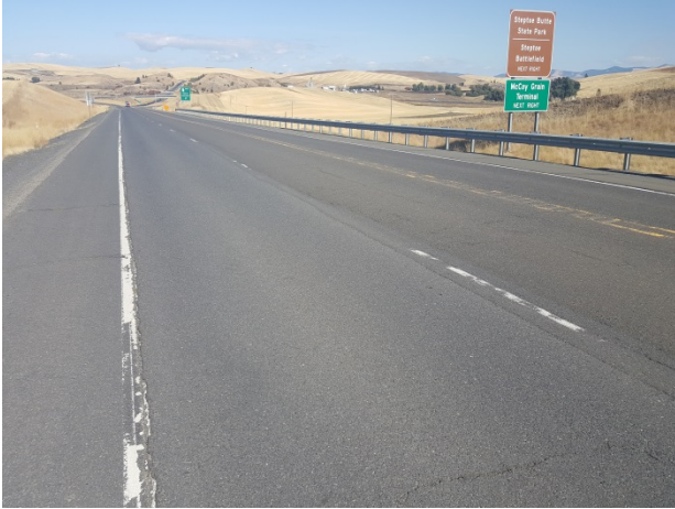
Figure 112. ER8, SR195, Good, are 39 months. Blade patch used to fill wheel path ruts. Additional patches placed in 2017.
