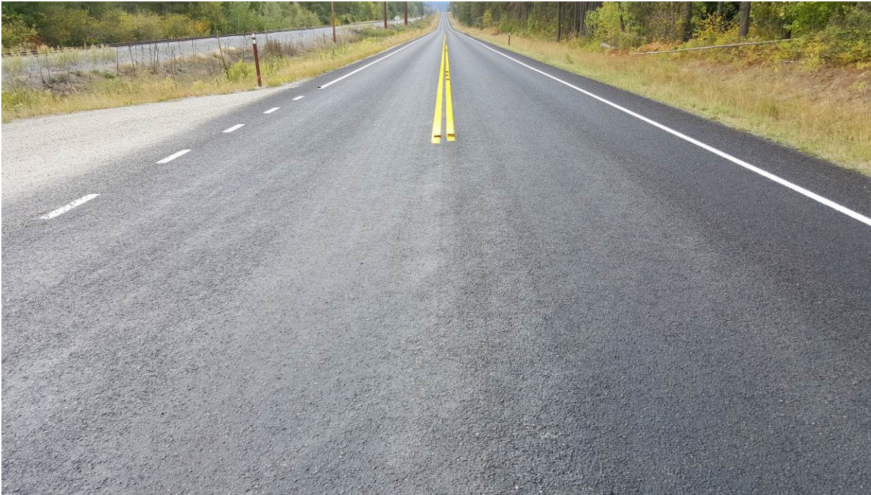
Figure 47. ER7, SR20, three years after installation. Full lane chip seal installed under Contract 8728, US 2 ET AL 2015 Eastern Region Chip Seal.
