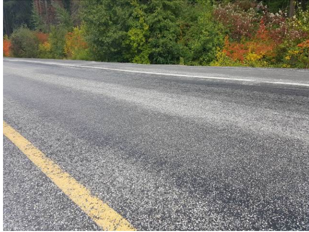
Figure 105. NC3, SR207, Good, age 38 months. Dig out patches flushing through the chip seal after 12 months. This is actually a HBST with 100% embedment in the wheel paths.
