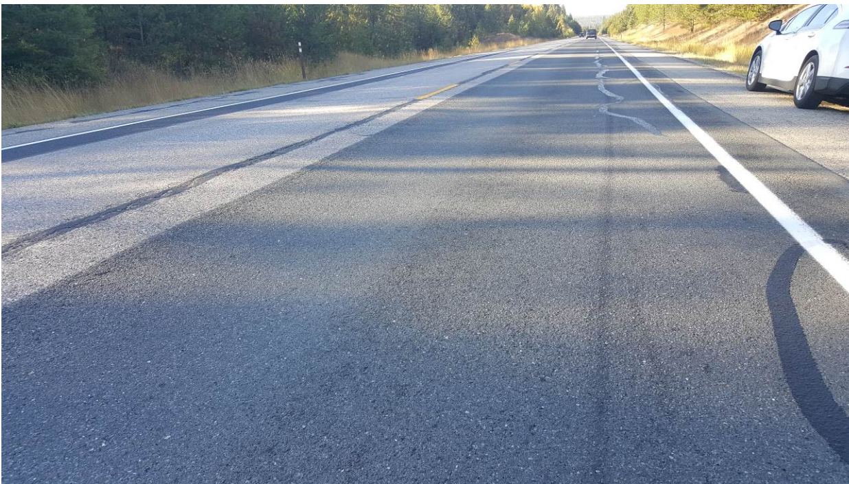
Figure 123. ER9a, SR395, two years after installation. Longitudinal reflection cracking has been sealed. Note slight flushing in the left wheel path.
