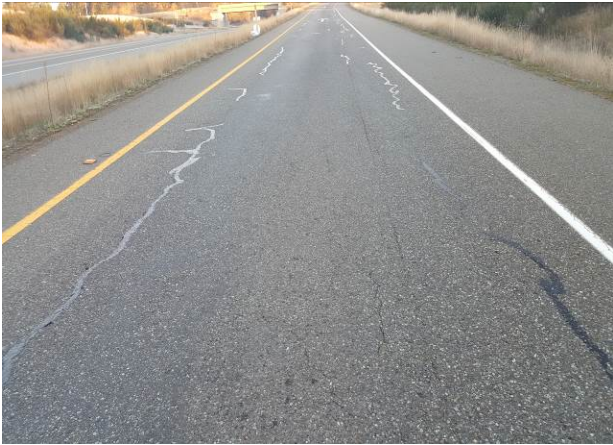
Figure 4. OR8, SR8, Ramp, Poor, age 51 months.
