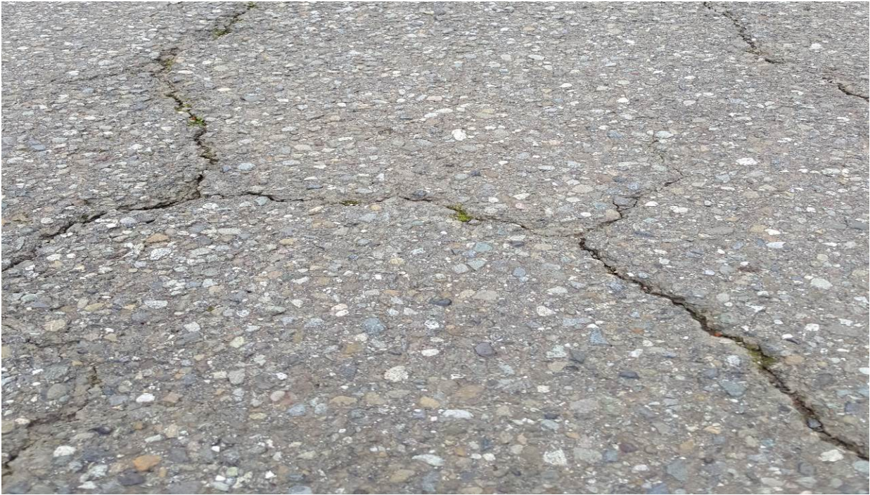
Figure 132. OR3a, SR101, three years after the other section were treated. Cracks are wide but not spalling.
