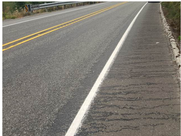
Figure 23. OR22, SR101, Good, age 26 months. Loss of aggregate at bottom of super elevation.
