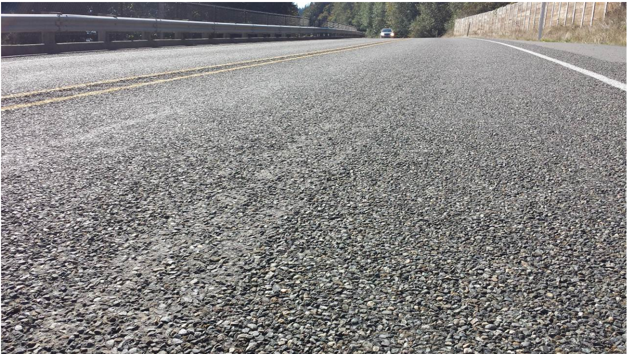
Figure 52. OR1a, SR101, two years after installation. Shadowing of the sealed cracks visible.
