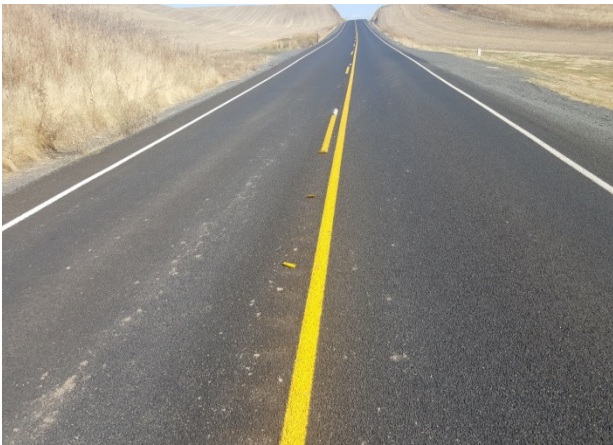
Figure 114. ER20, SR272, Good, age 24 months. Transverse crack reflecting through the patch. HMA grind/inlay in 2017, 9031.
