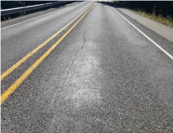
Figure 20. OR1b, SR101, Poor, age 62 months. Longitudinal cracking noted at 21 months. Slight flushing in the wheel paths.
