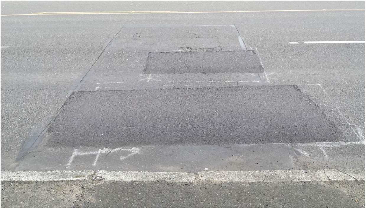
Figure 86. OR5, SR7, one year after installation. No change in the dig out patches.
