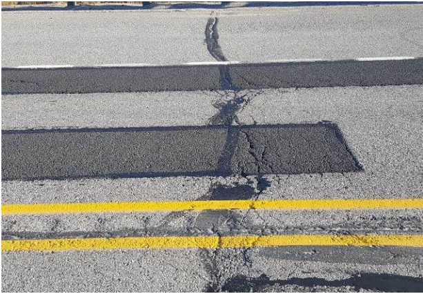
Figure 66. ER9, SR395, Good, age 37 months. Additional dig outs installed in 2015. Transverse reflection cracking noted in 2017.
