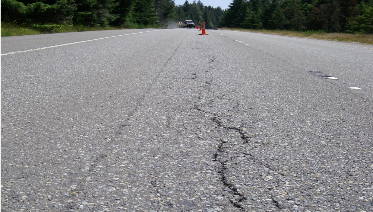
Figure 78. OR2, SR8, prior to treatment. Alligator cracking in the left wheel path. This is not the same location as the following photos which had alligator cracking in both wheel paths.
