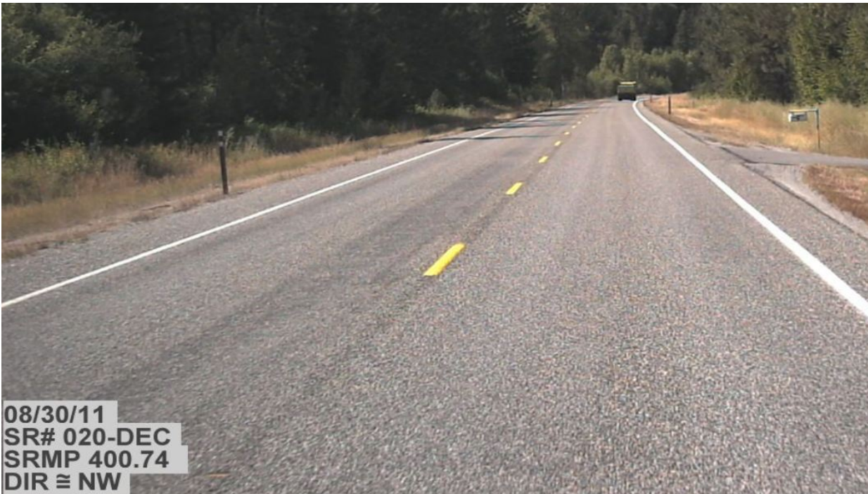
Figure 43. ER7, SR20, prior to treatment. Rutting is visible in the wheel paths.
