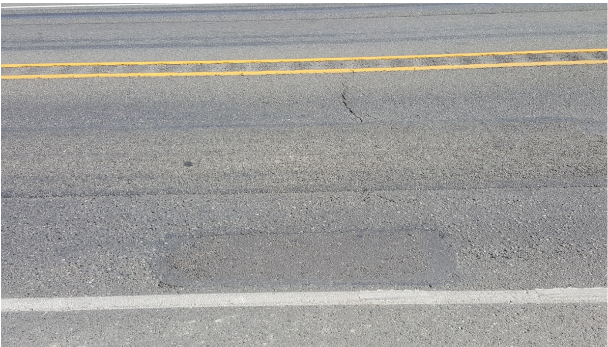
Figure 35. OR12, SR20, two years after installation. Some loss of aggregate but no reflection cracking.
