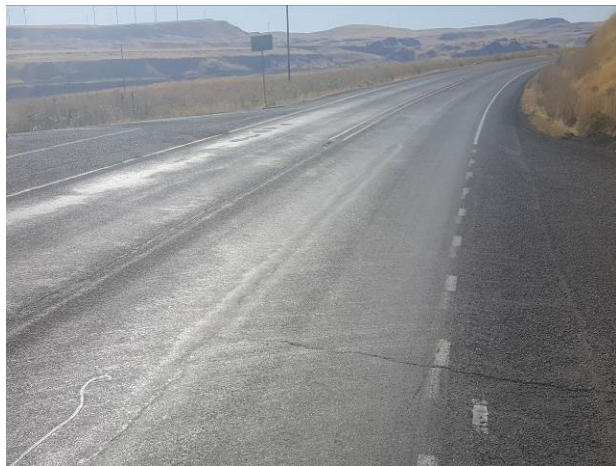
Figure 103. SW1a, SR14, Poor, age 62 months. Transverse and longitudinal reflection cracking and flushing noted at 12 months after installation. Potholes developed at 50 months.
