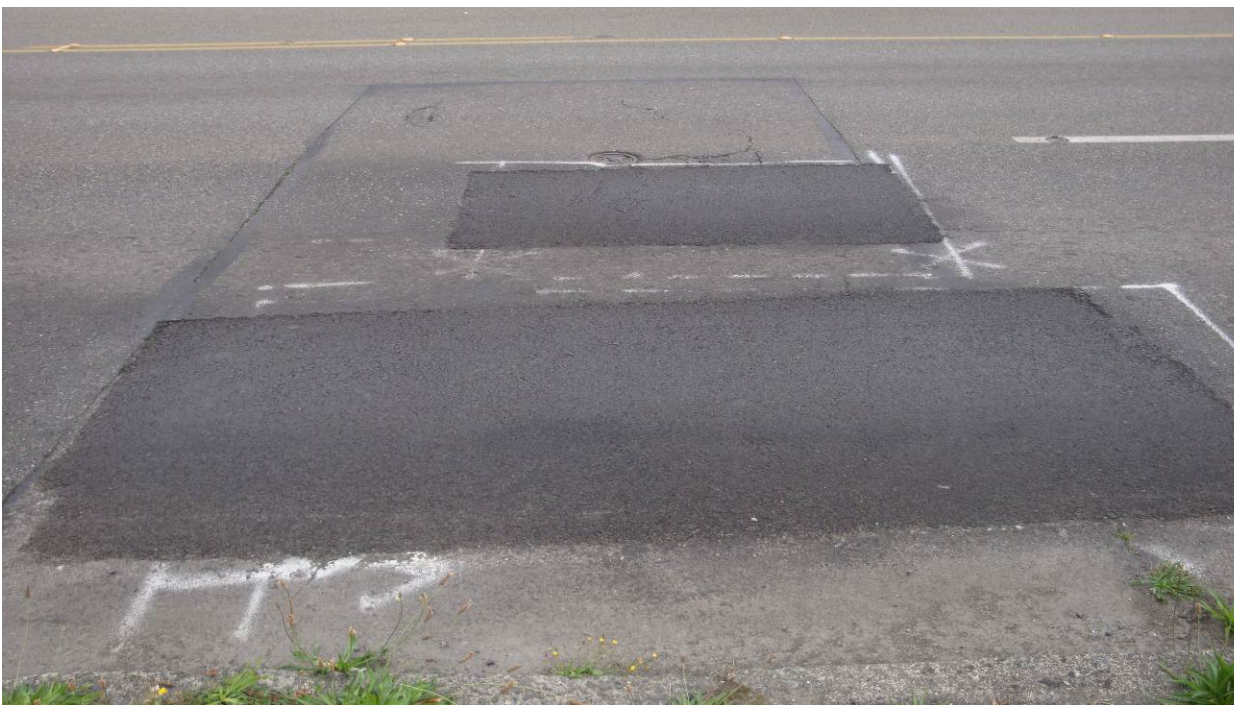
Figure 85. OR5, SR7, immediately after installation in 2013. Dig out patches look good. They appear to be related to utility cuts in original pavement.
