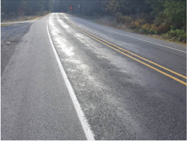
Figure 104. OR14, SR7, Good, age 51 months. Dig out patches flushing through the chip seal at 27 months.
