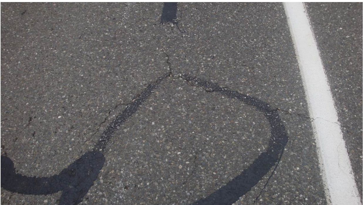
Figure 15. OR1, SR101, one year after installation. Slight wear of sealant over banding.
