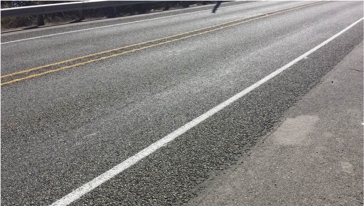
Figure 26. OR1b, SR101, two years after installation. Longitudinal crack appears to have “healed”. Slight flushing in the wheel paths.
