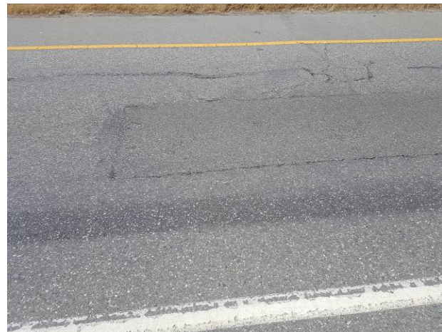
Figure 91. OR4, SR3, Good, age 50 months. Dig out patches and crack sealing in excellent condition.
