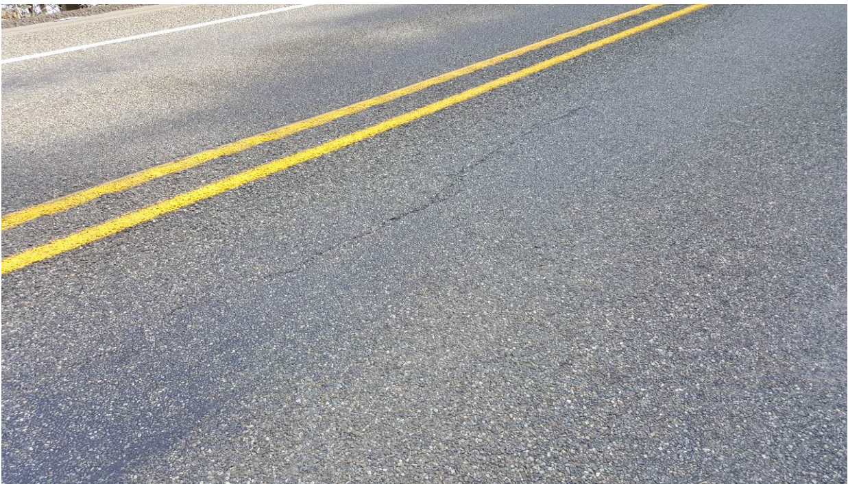
Figure 27. OR1b, SR101, three years after installation. Longitudinal crack is getting longer and wider. Flushing in the wheel paths is about the same.
