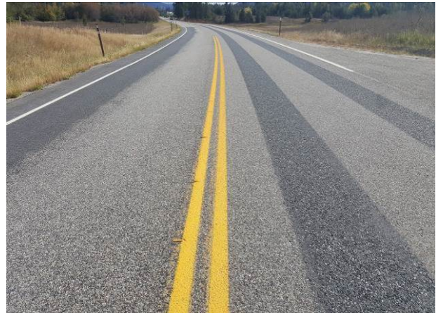
Figure 41. ER18, SR31, Good, age 26 months. BST in 2017, C9031. Photo is from 2016.
