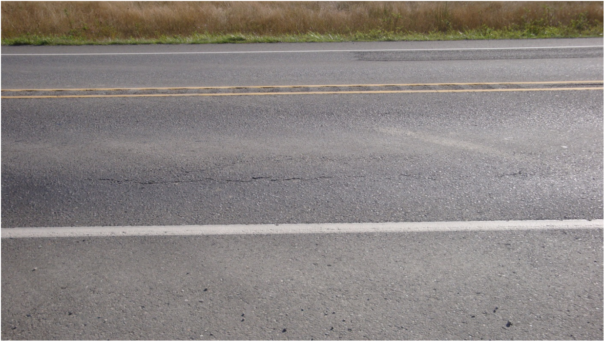
Figure 32. OR12, SR20, prior to treatment. Longitudinal and alligator cracking present in the wheel paths.
