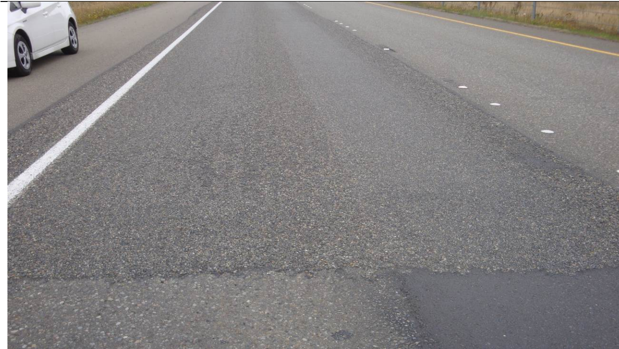
Figure 107. OR2a, SR8, one year after installation. Slight flushing in the wheel paths over the dig out patches.
