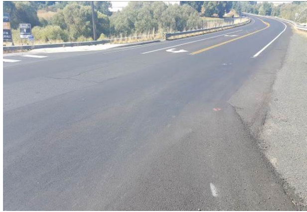
Figure 67. ER11, SR270, Fair, age 37 months. HMA grind/inlay in 2017, C9062.
