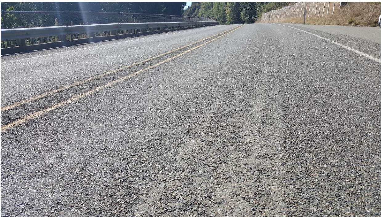
Figure 54. OR1a, SR101, four years after installation. Slight amount of rutting beginning to appear. Flushing does not seem to be a big issue.
