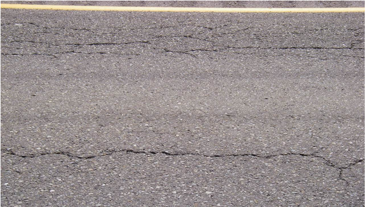
Figure 14. OR1, SR101, prior to treatment. Cracks exceed 1/4 inch in width in places.
