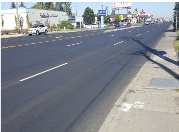
Figure 127. ER2a, US2, Poor category, age 62 months. Dig outs, crack sealing and patching were necessary to preserve the roadway. HMA grind/inlay in 2017, C9063.
