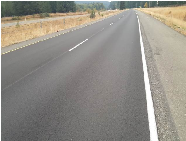
Figure 56. OR2, SR8, Fair, age 62 months. HMA grind/inlay in 2017, C9001.
