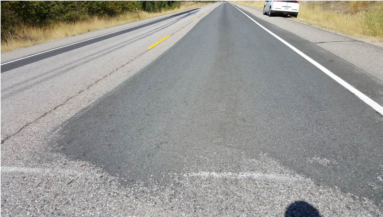
Figure 122. ER9a, SR395, one year after installation in 2014. Some wear of the blade patch at each end. Transverse cracks reflected through the blade patch after only one year.
