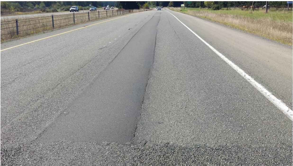
Figure 80. OR2, SR8, two years after installation. No change in condition of patch.
