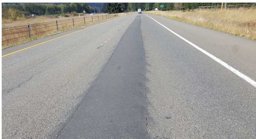
Figure 144. OR2 dig outs on SR 8. (September 2016)
