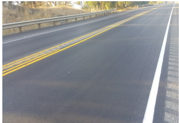
Figure 119. ER37, SR395, Fair, age 25 months. Excellent performance. HMA grind/inlay in 2017, C9105.
