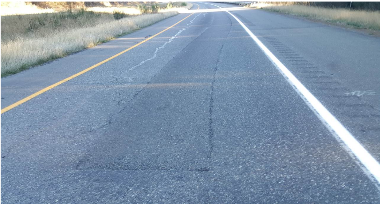
Figure 98. OR4, SR3, three years after installation. No change in dig out patch or crack sealing.
