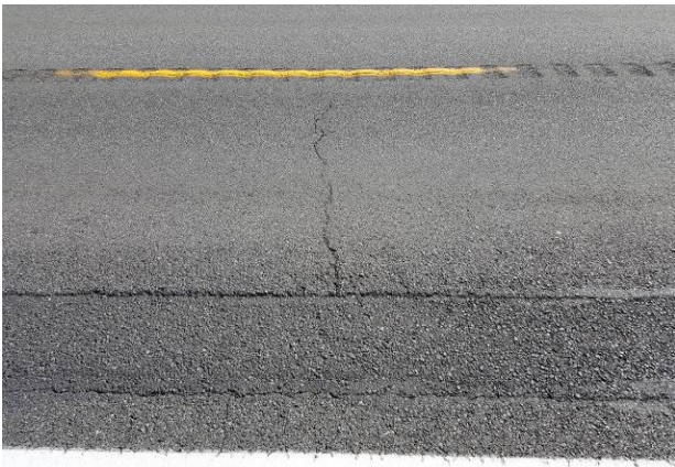
Figure 64. OR11, SR20, Good, age 49 months. Raveling of patch edges noted at 25 months.
