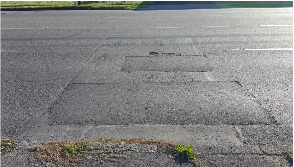
Figure 87. OR5, SR7, two years after installation. No change in the dig out patches.
