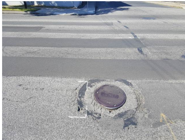
Figure 59. ER4, US2, Fair, age 62 months. Additional dig outs installed in 2013 and 2015. Note different colors of dig out patches done in different years. HMA grind/inlay scheduled in 2018, C9187
