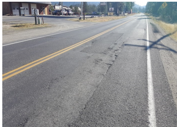
Figure 128. ER3a, SR291, Fair category, 62 months. Dig outs, crack sealing and patching were necessary to preserve the roadway. HMA grind/inlay scheduled in 2018, C9223
