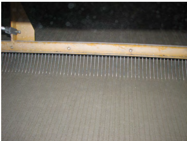
Figure 15. I-5 formation of longitudinal tined texture.
