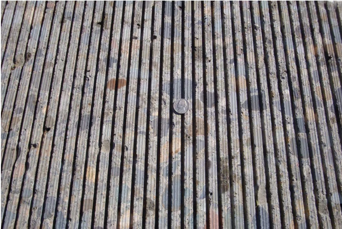
Figure 21. I-82 NGCS October 2010 after construction.
