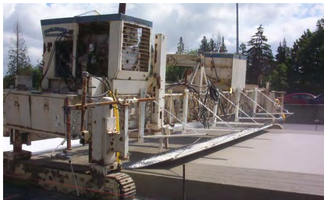
Figure 11. Installation of carpet drag texture on I-5.
