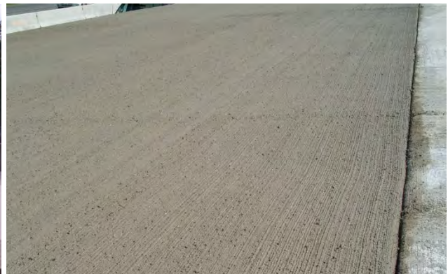
Figure 12. I-5 fresh carpet drag texture.
