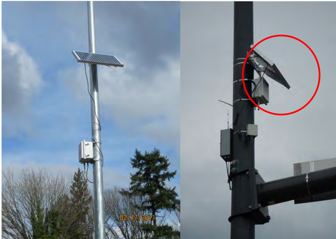
Figure 3-9. BlueTOAD sensor design and components
