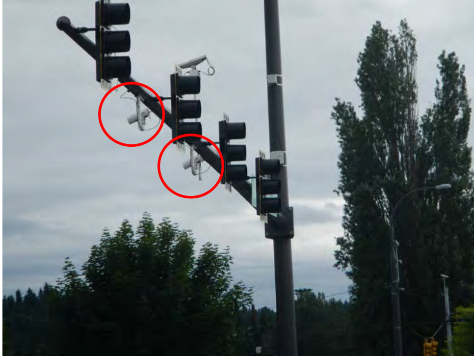
Figure 3-8. Pips P327 Spike ANPR sensor
