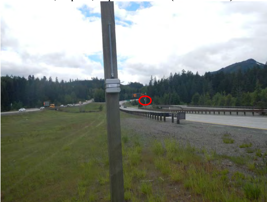
Site C, Milepost 70, Easton, Washington
