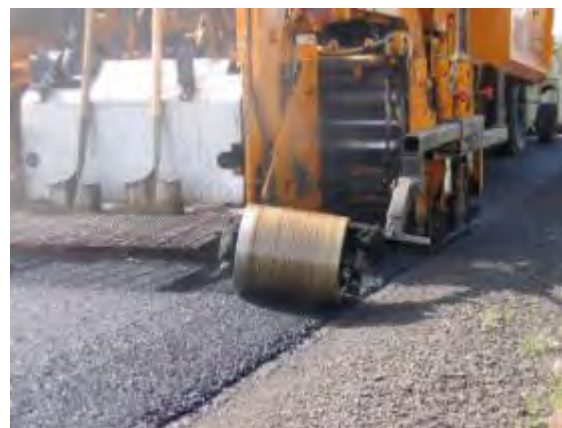
Figure 17. Paver forming and compacting pavement edge treatment.
