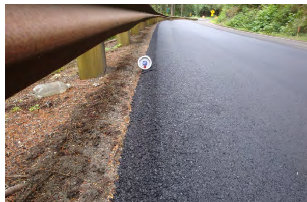
Figure 60. Pavement edge treatment next to guardrail.
