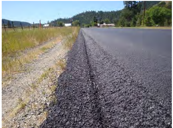
Figure 47. Another view of the edge treatment.
