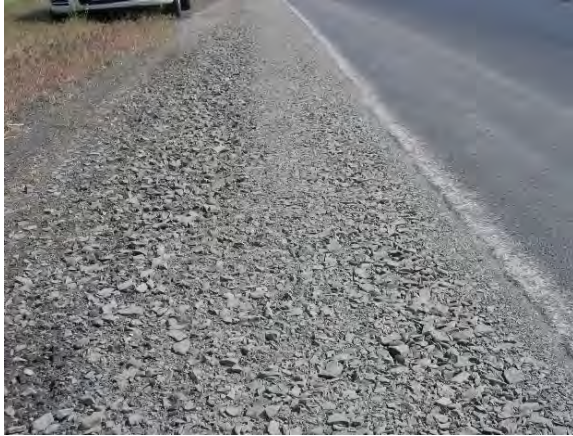
Figure 24. Finished pavement with shoulder material in place.
