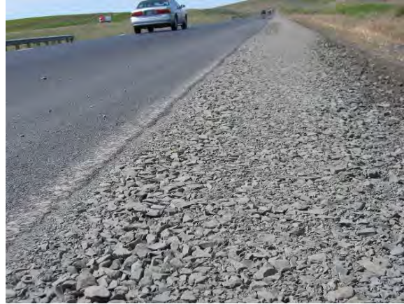
Figure 25. Finished pavement with shoulder material in place.
