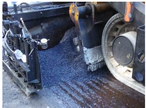
Figure 54. Mix passing through the end gate.
