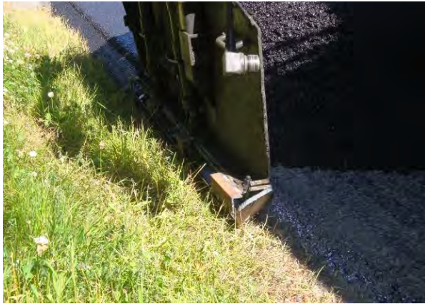
Figure 29. End view of TransTech pavement edge hardware without the roller.
