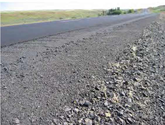
Figure 16. SR 395 before overlay. Note wide stable shoulder.
