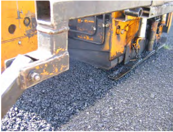
Figure 18. Close-up of paver screed.
