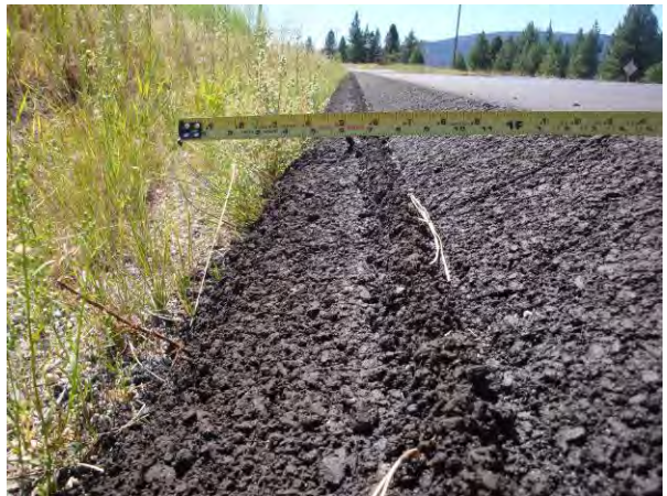
Figure 45. Close-up of edge treatment slope.
