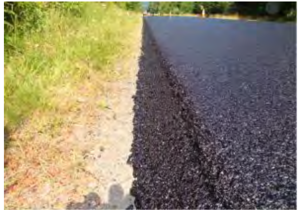
Figure 30. Pavement edge formed by the TransTech hardware prior to adding the roller. Note open texture of the HMA.
