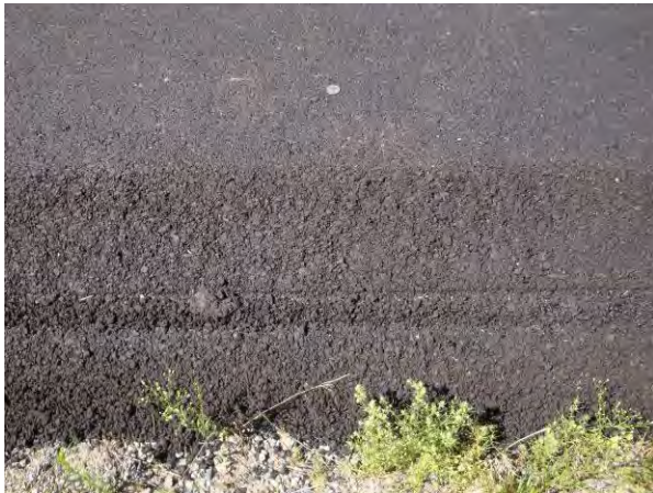
Figure 46. Side view of edge treatment.
