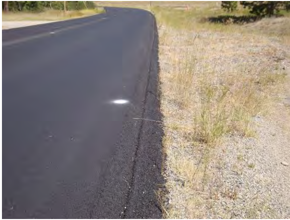
Figure 48. Edge treatment and shoulder area.
