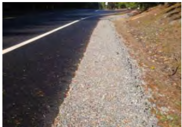
Figure 34. Finished pavement with dressed shoulders.
