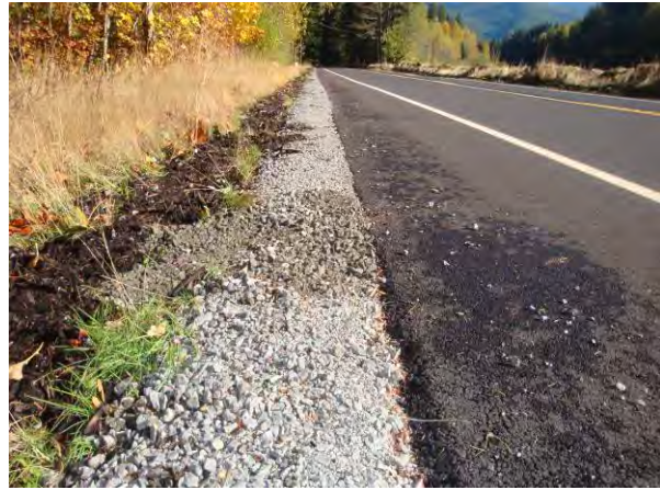
Figure 36. Shoulder material put back in place.
