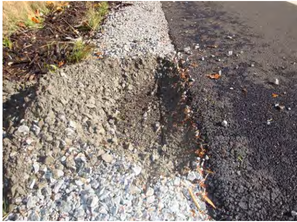
Figure 35. Dig out showing slope of pavement edge.
