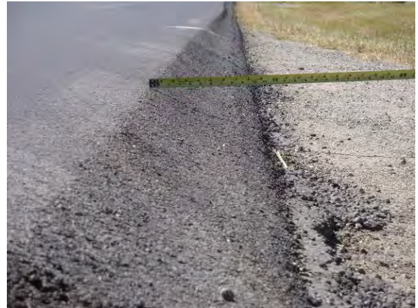
Figure 51. Closer view of slope of edge treatment.
