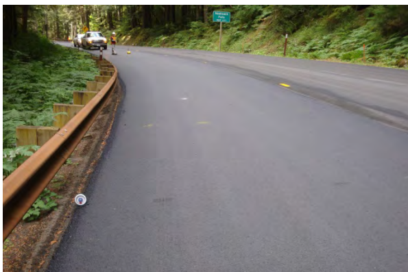
Figure 59. Pavement edge treatment next to guardrail.
