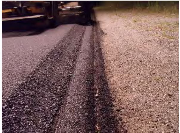
Figure 43. Pavement edge treatment produced by the Advant-Edge™.
