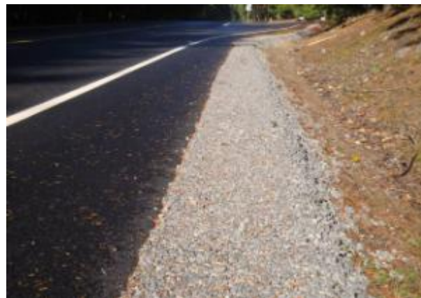
Figure 34. Finished pavement with dressed shoulders.
