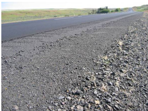
Figure 16. SR 395 before overlay. Note wide stable shoulder.
