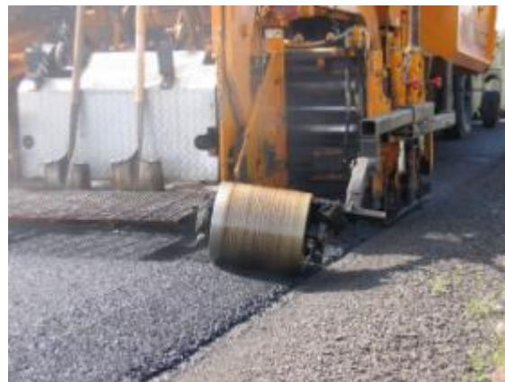
Figure 17. Paver forming and compacting pavement edge treatment.
