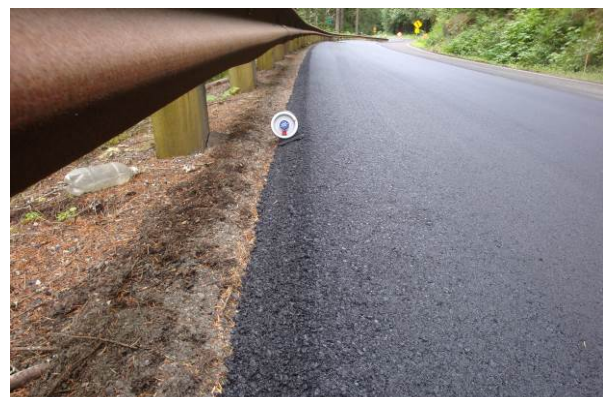
Figure 60. Pavement edge treatment next to guardrail.
