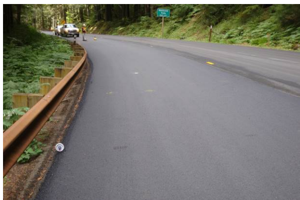
Figure 59. Pavement edge treatment next to guardrail.
