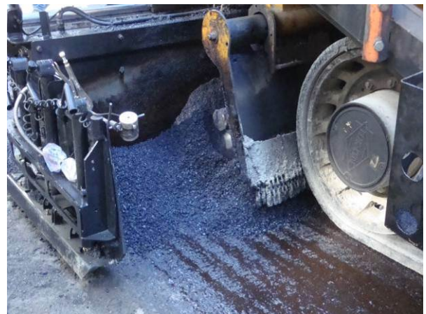
Figure 54. Mix passing through the end gate.
