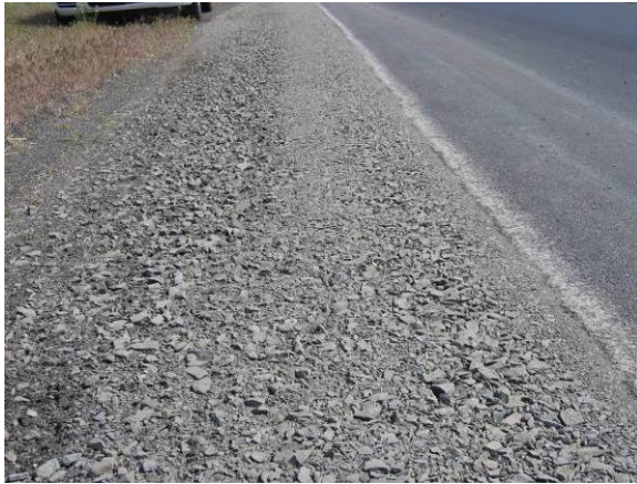
Figure 24. Finished pavement with shoulder material in place.
