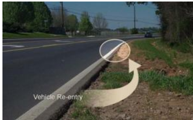
Figure 5. Vertical drop off at pavement edge. (FHWA Safety Edge SM PowerPoint)
