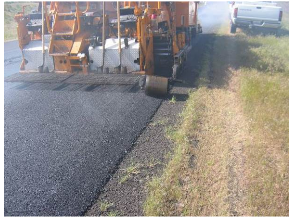
Figure 21. View of rolled pavement edge treatment.
