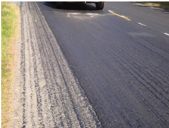
Figure 27. SR 410 prior to construction.
