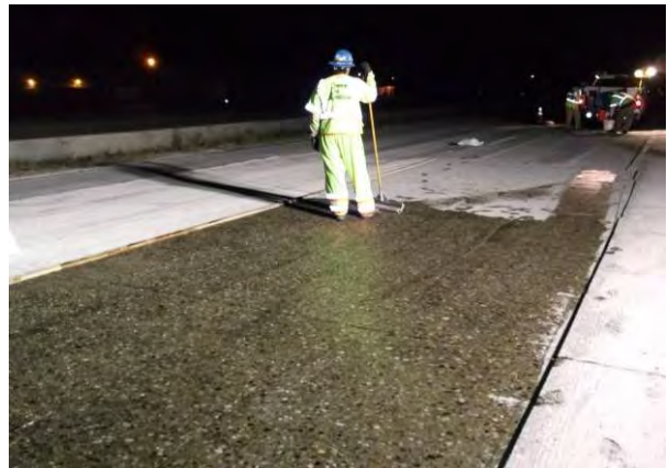
Figure 15. HMWM prime coat being applied. Wheel path inlay section is in the background
