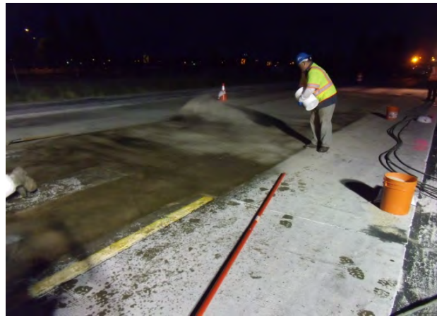
Figure 26. Top dressing wheel path inlay section.
