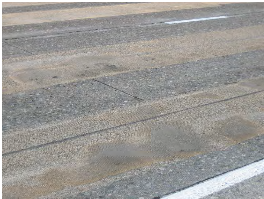
Figure 54. Close-up of wheel path inlay section after diamond grinding.
