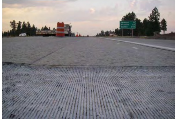
Figure 13. West end of full lane section.
