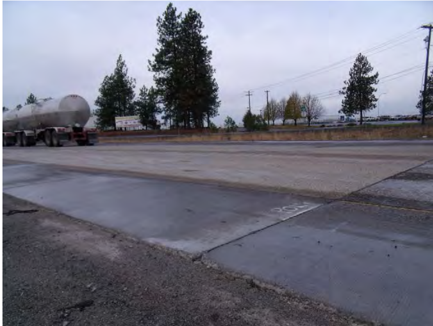
Figure 45. Full lane inlay section after diamond grinding.
