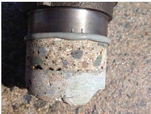
Figure 10. Pull off test 1.
