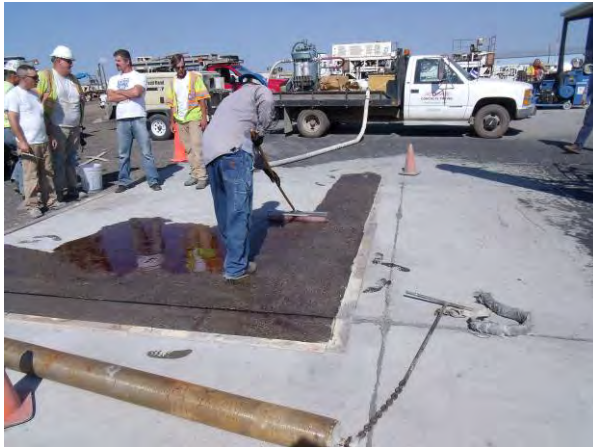
Figure 6. Rolling of high molecular weight methacrylate (HMWM) prime coat.
