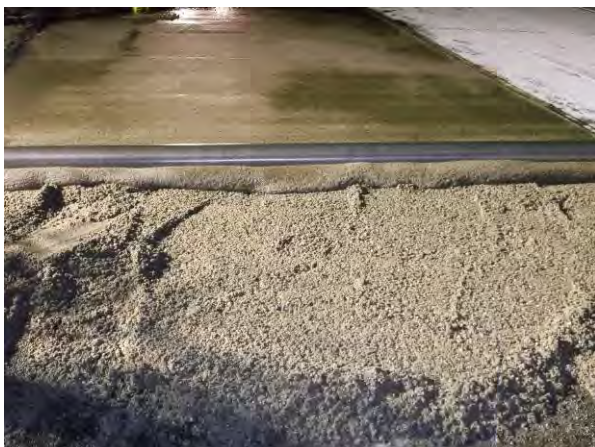
Figure 16. Roller screed finished PPC.
