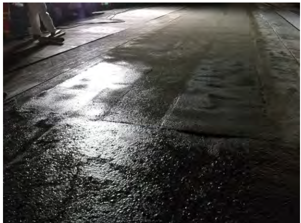
Figure 27. Finished wheel path section.
