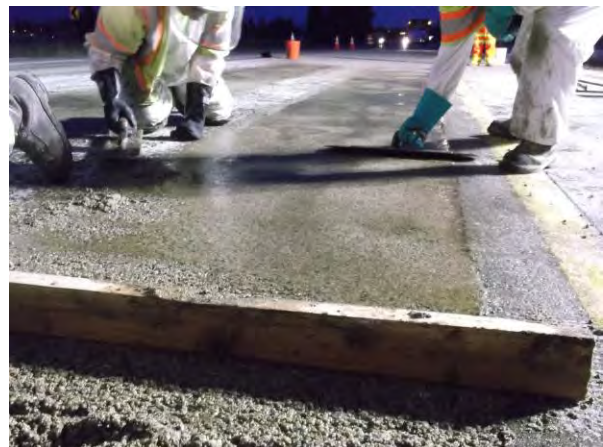
Figure 23. Using 2x4 to screed PPC.
