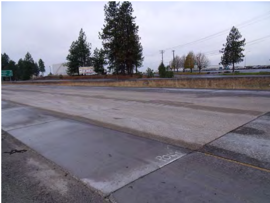
Figure 46. Full lane inlay section after diamond grinding.
