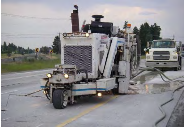
Figure 12. Diamond grinding machine.
