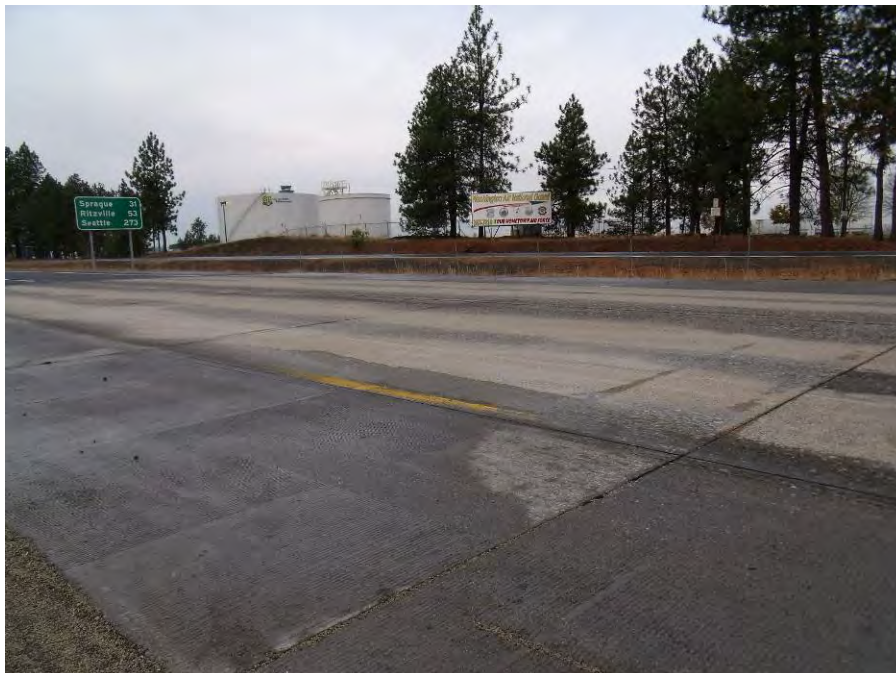
Figure 56. Rut fill section after diamond grinding.
