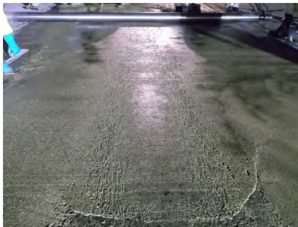
Figure 33. Finished PPC in the rut fill section.
