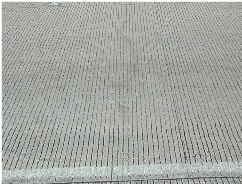
Figure 2. Concrete pavement on Interstate 45 in Houston, Texas after thirteen years of traffic.
