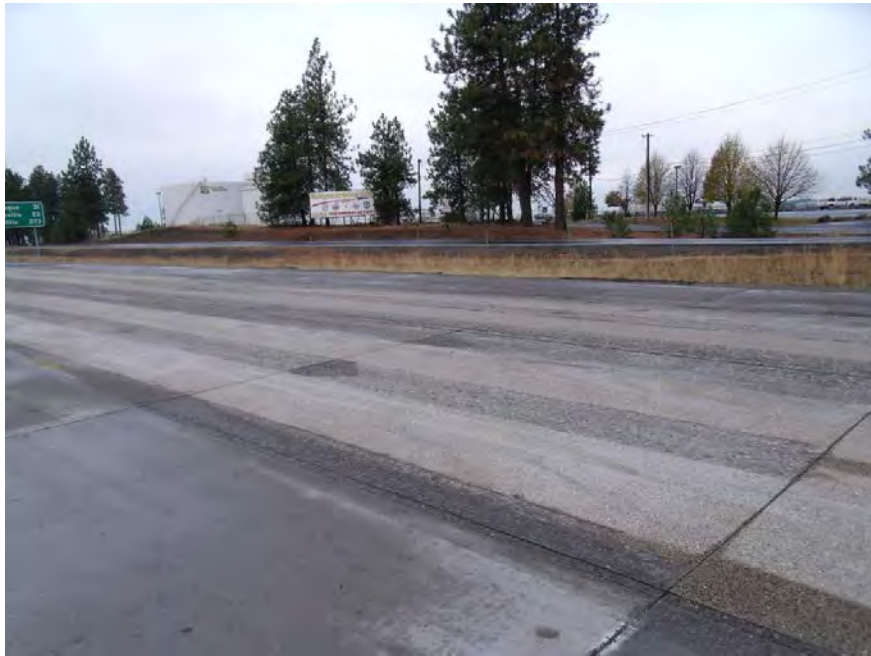
Figure 51. Wheel path inlay section after diamond grinding.
