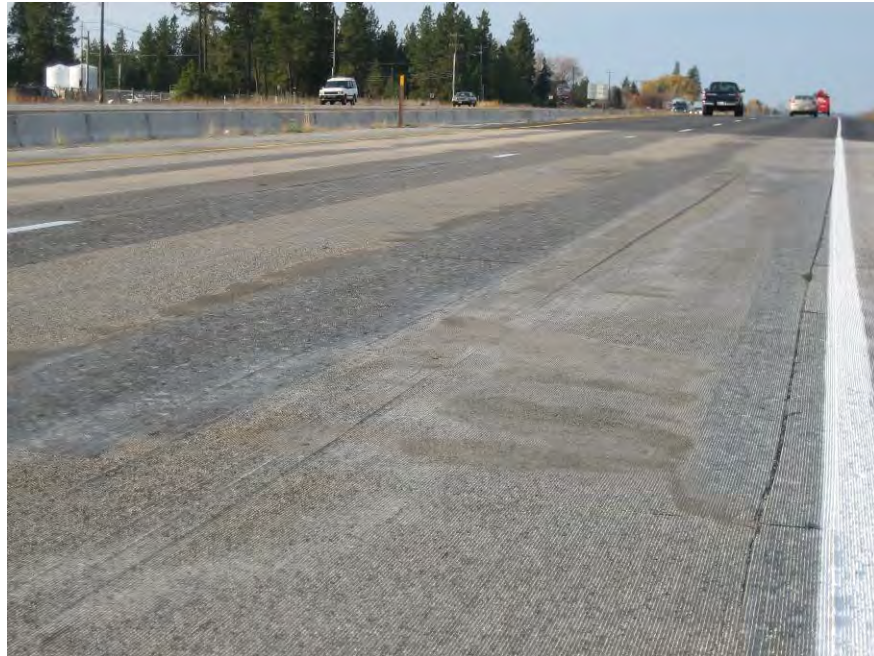
Figure 53. Wheel path inlay section after diamond grinding.
