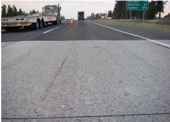
Figure 28. Rut fill section prior to overlay.
