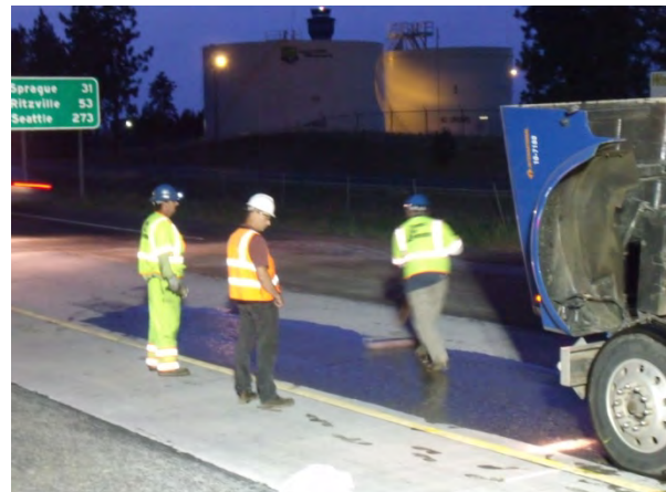
Figure 31. HMWM prime coat application.
