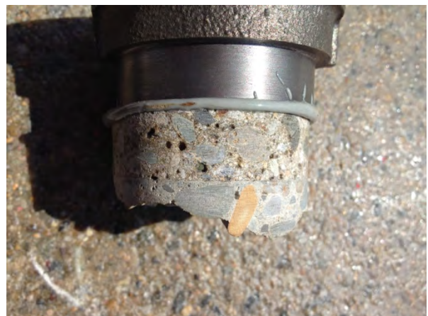
Figure 11. Pull off test 3.
