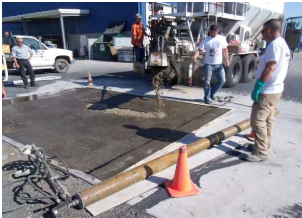
Figure 8. PPC being placed.
