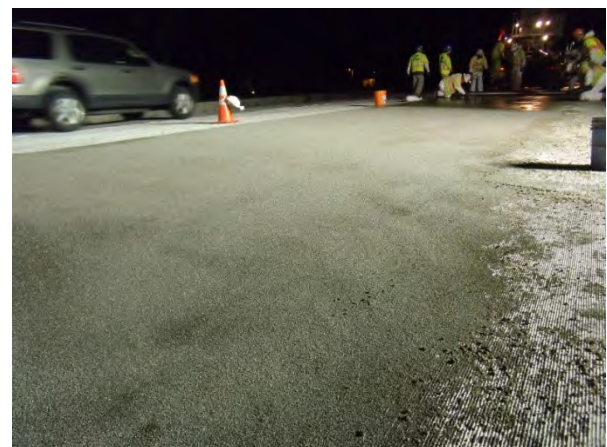
Figure 17. Finished PPC after top dressing with aggregate.
