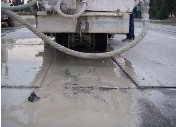
Figure 18. Diamond grinding wheel path inlay section.
