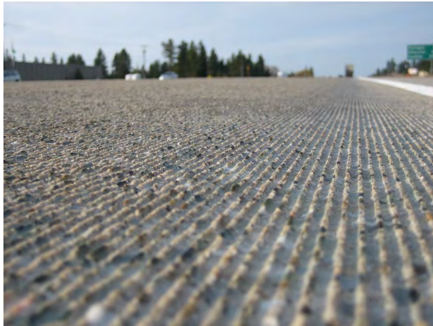
Figure 49. PPC texture of full lane inlay section after diamond grinding.
