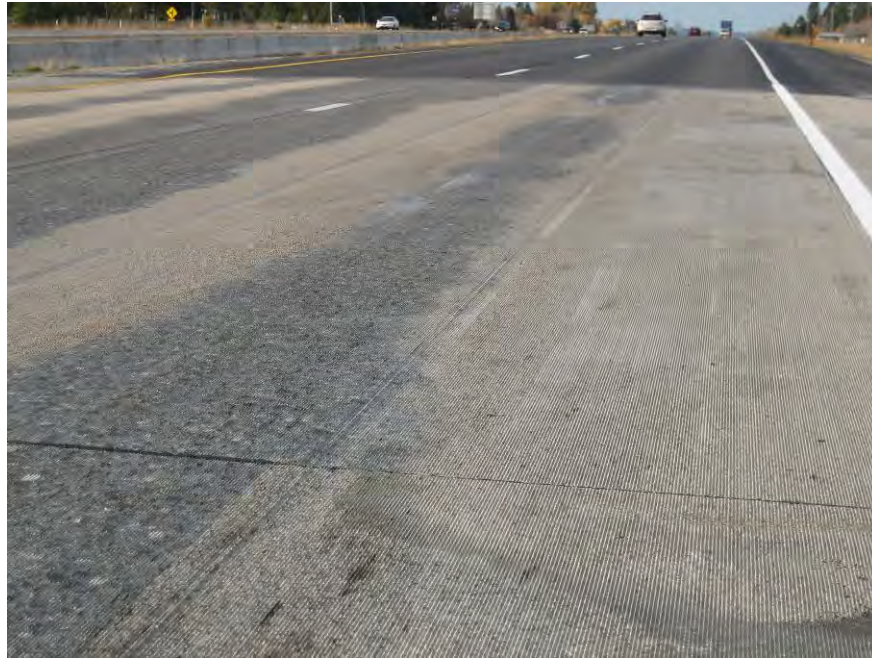
Figure 57. Rut fill section after diamond grinding
