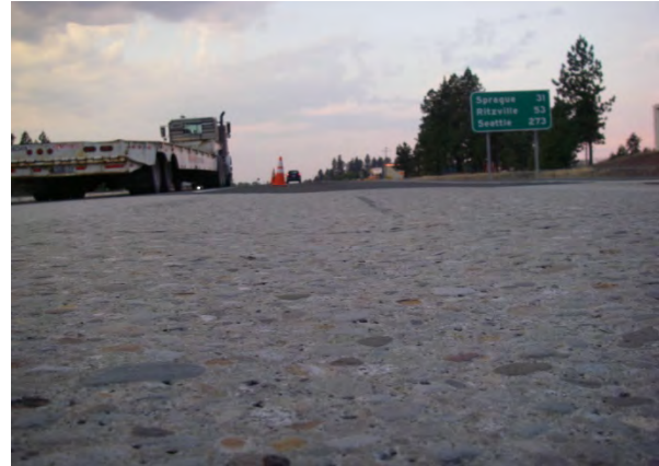
Figure 29. Close-up of rut fill section.
