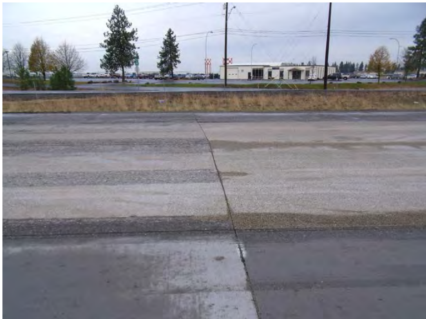
Figure 52. Wheel path inlay section after diamond grinding.
