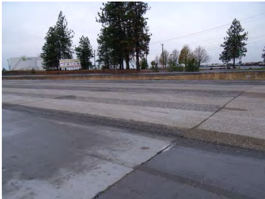
Figure 50. Wheel path inlay section after diamond grinding.
