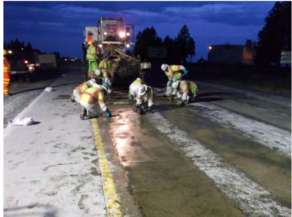
Figure 25. Final hand troweling of the wheel path inlay section.
