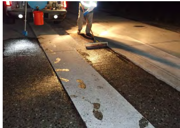
Figure 21. HMWM prime coat applied in wheel paths.
