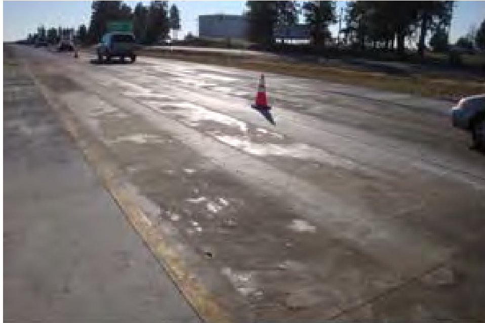
Figure 40. Wheel path inlay section of PPC.
