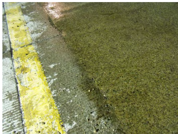
Figure 32. Close-up of finished PPC prior to top dressing with aggregate.
