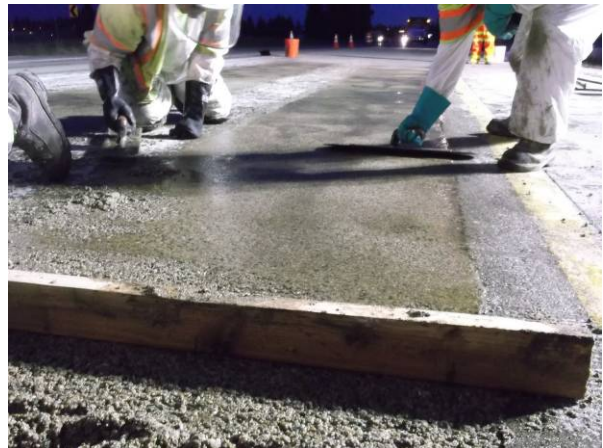
Figure 23. Using 2x4 to screed PPC.
