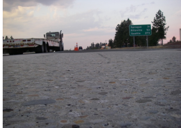
Figure 29. Close-up of rut fill section.
