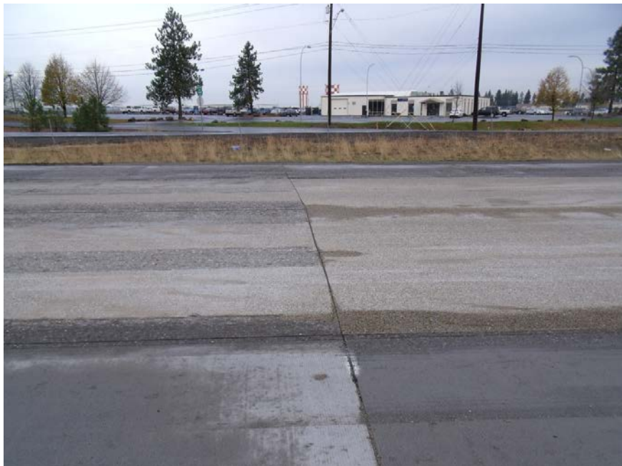
Figure 52. Wheel path inlay section after diamond grinding.
