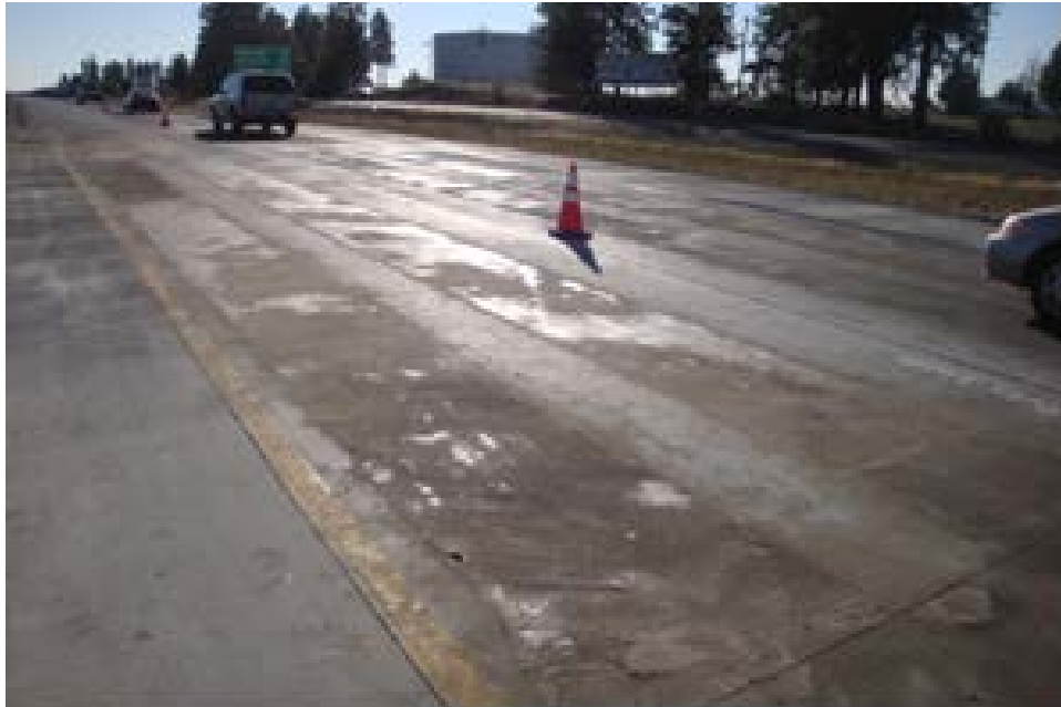
Figure 40. Wheel path inlay section of PPC.
