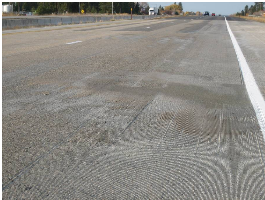
Figure 48. Full lane inlay section after diamond grinding in foreground, other sections in background.
