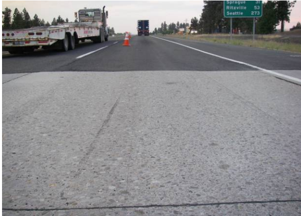
Figure 28. Rut fill section prior to overlay.
