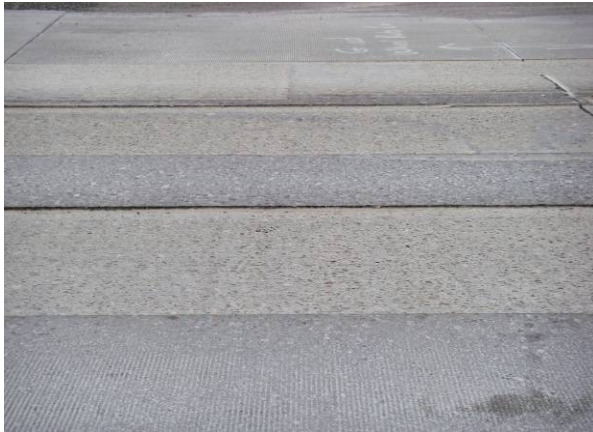
Figure 20. Side view of wheel path inlay section.
