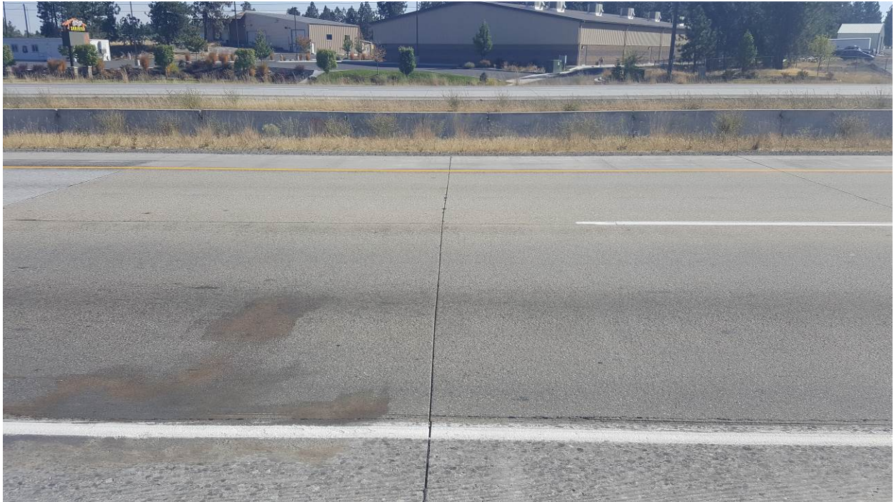
Figure 64. Side view of the full lane mill and fill section. The discoloration has been present from day one. No cracking or delaminations are visible (September 27, 2017).
