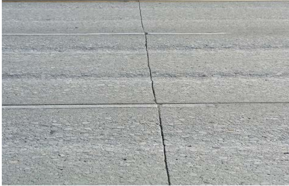
Figure 3. Studded tire wear on a concrete pavement (I-90 Spokane).
