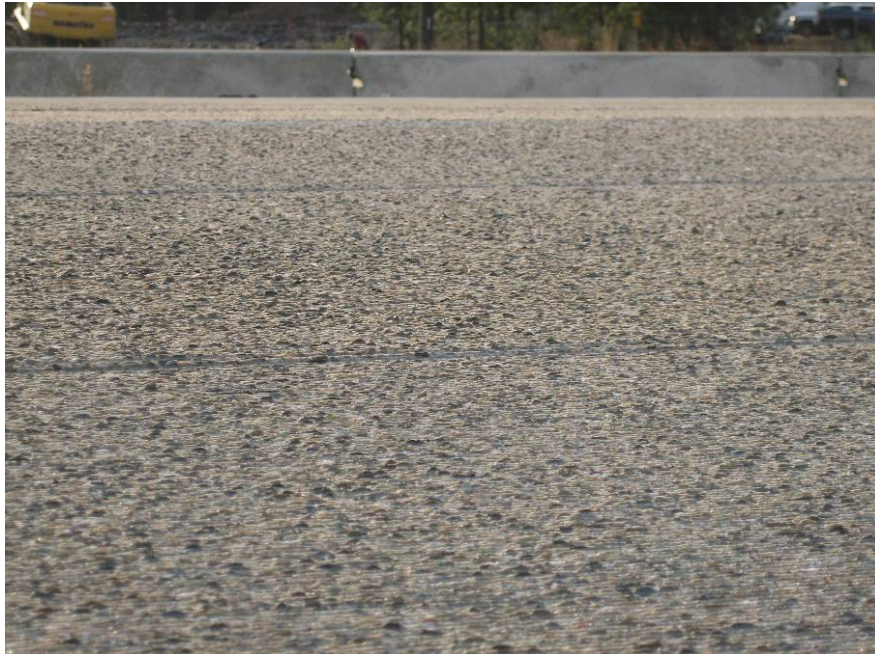
Figure 47. Close-up of full lane inlay section after diamond grinding.
