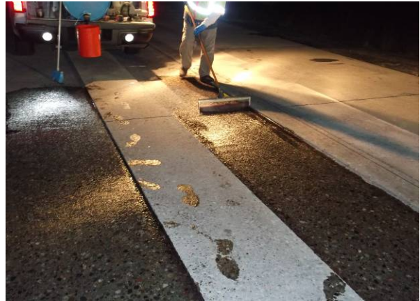
Figure 21. HMWM prime coat applied in wheel paths.
