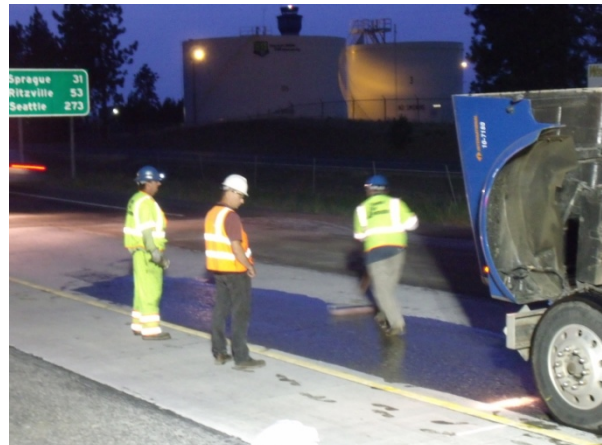
Figure 31. HMWM prime coat application.
