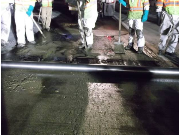
Figure 34. Distributing PPC in front of roller screed in rut fill section.
