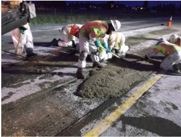
Figure 24. Spreading and striking off PPC in wheel path inlay section.
