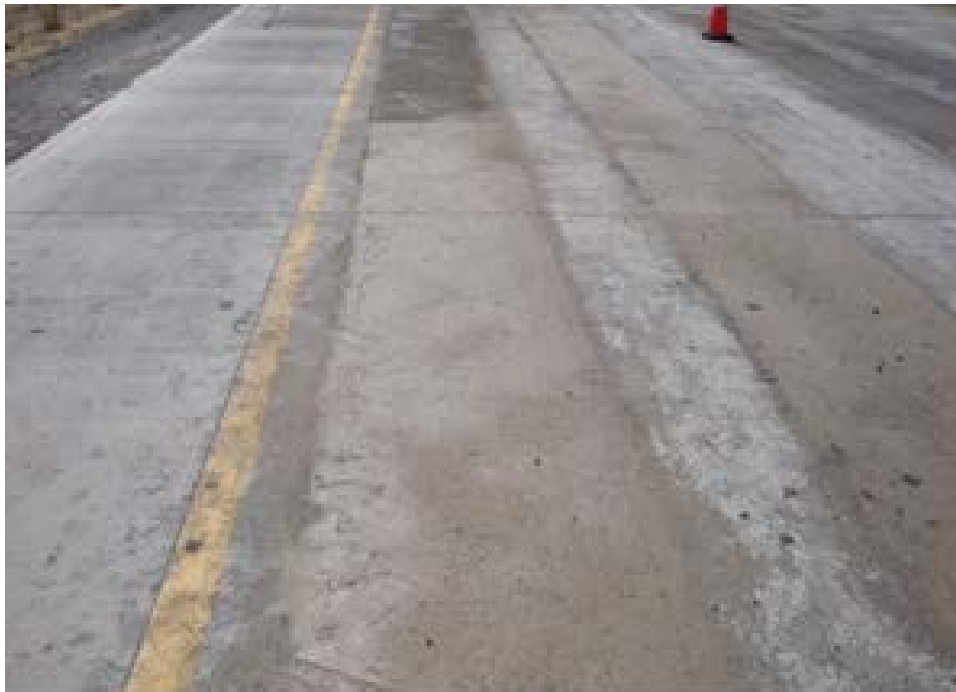
Figure 39. Close-up of wheel path inlay section of PPC.
