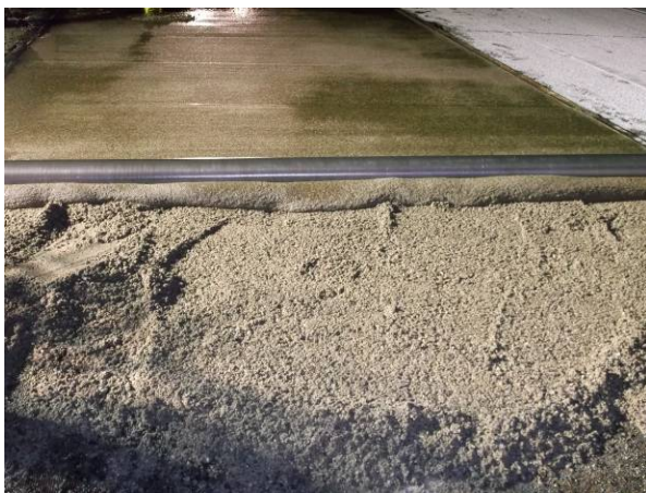
Figure 16. Roller screed finished PPC.
