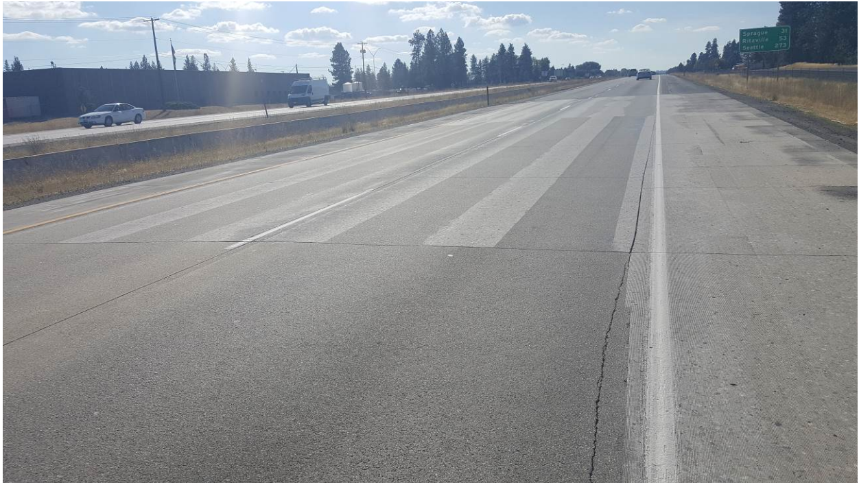
Figure 62. Longitudinal view of the wheel path mill and fill section. Note the sharp edges with no evidence of spalling of the PPC. No cracking or delaminations are visible (Sept. 27, 2017).
