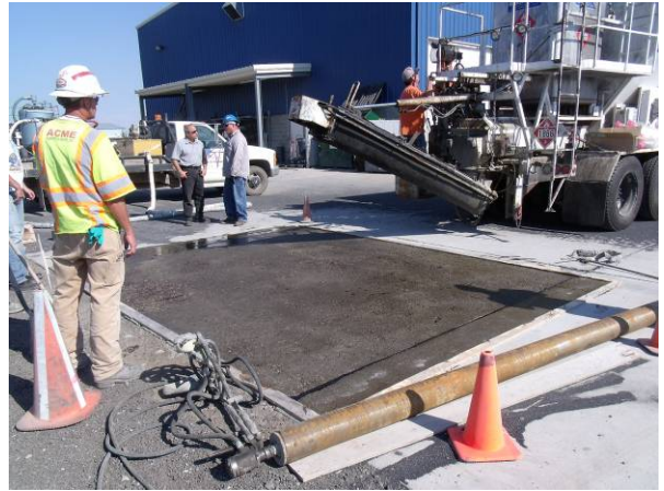
Figure 7. Mobile mixer moving into place to distribute PPC.
