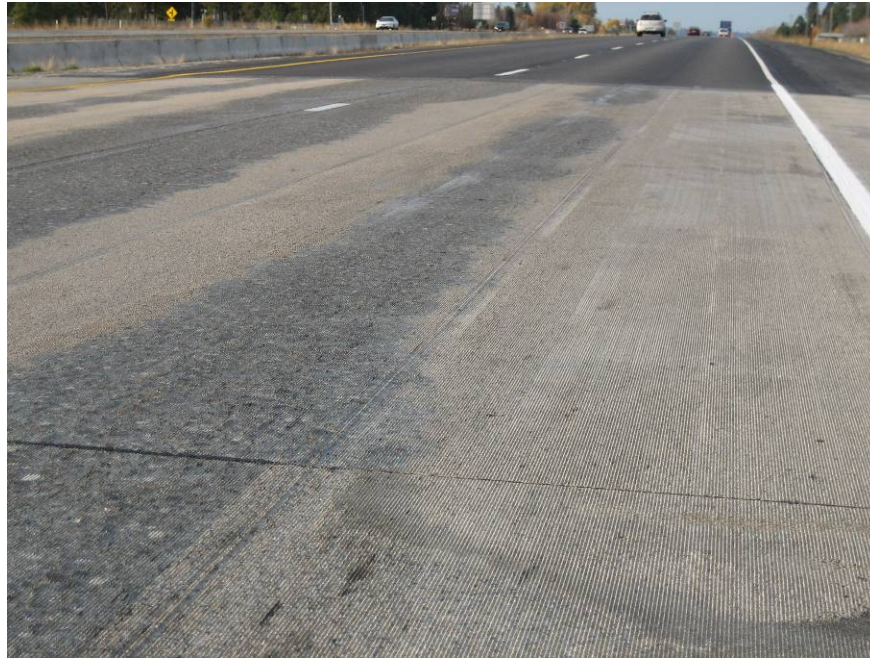
Figure 57. Rut fill section after diamond grinding.
