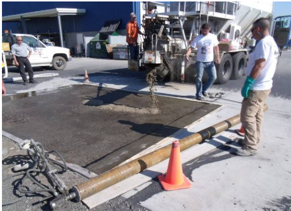
Figure 8. PPC being placed.
