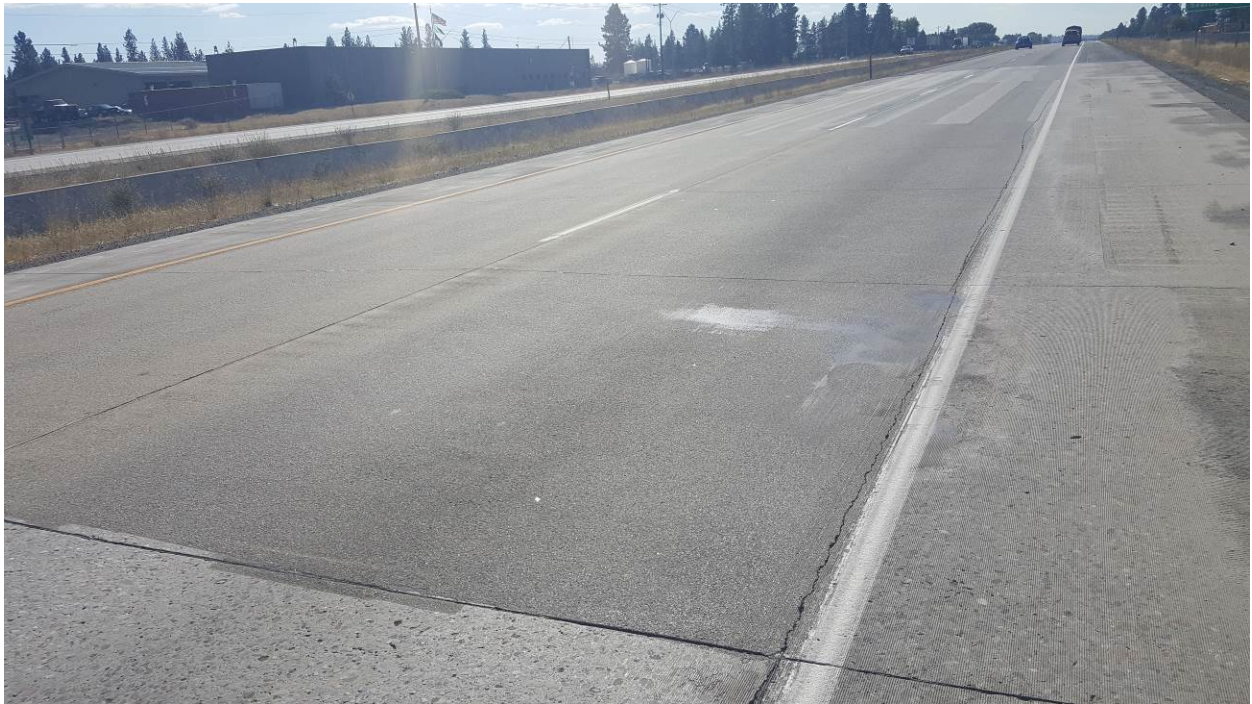
Figure 61. Longitudinal view of the full lane mill and fill section. Note the absence of spalling at the transverse joints or along the longitudinal edges of the slabs. No cracking or delaminations are visible (September 27, 2017).
