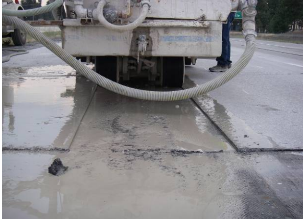
Figure 18. Diamond grinding wheel path inlay section.
