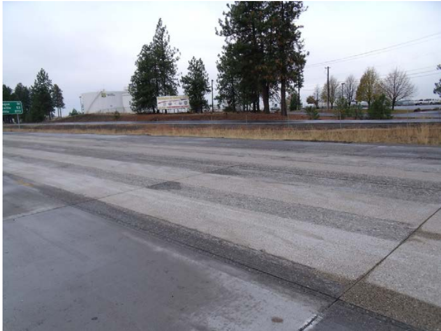
Figure 51. Wheel path inlay section after diamond grinding.
