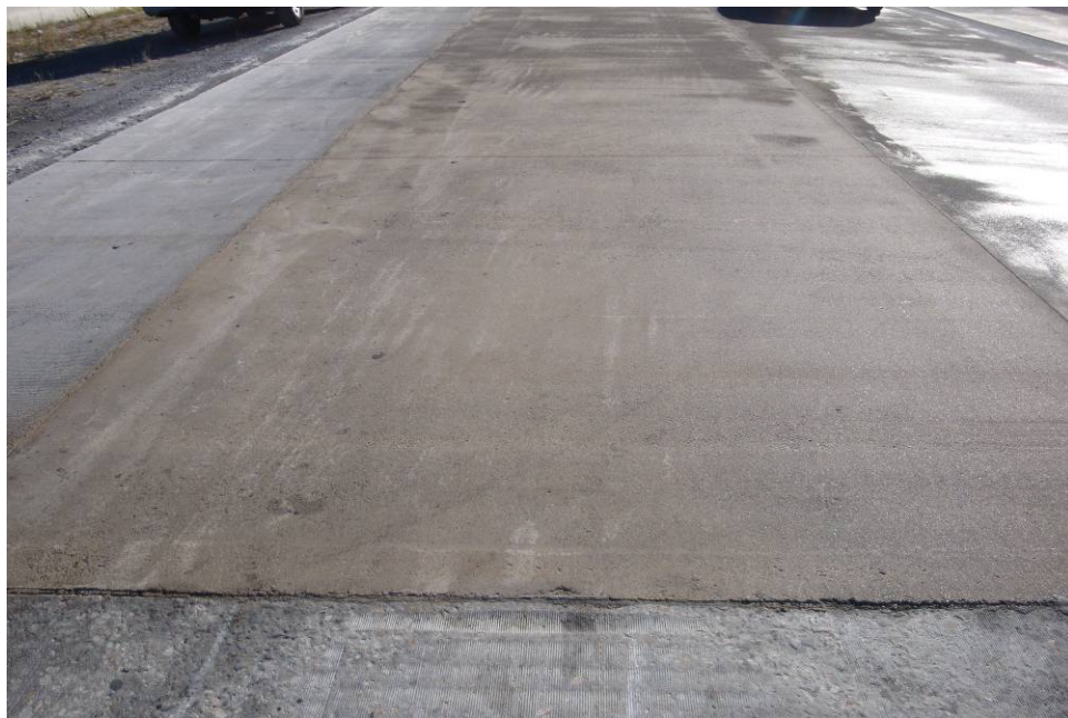
Figure 37. Close-up of the full lane section of PPC.
