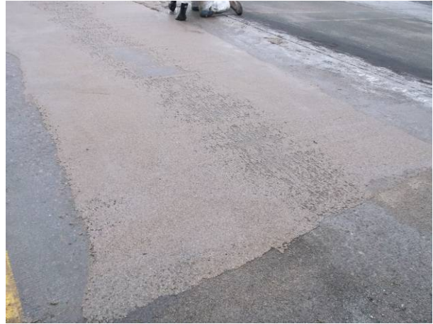
Figure 35. Finished rut fill section prior to application of top dressing.
