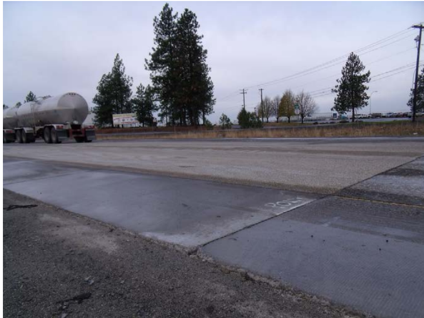
Figure 45. Full lane inlay section after diamond grinding.
