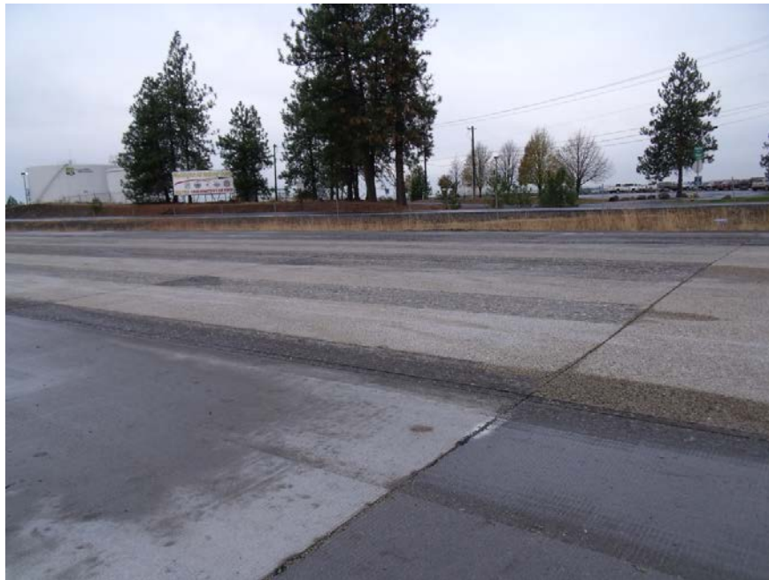
Figure 50. Wheel path inlay section after diamond grinding.
