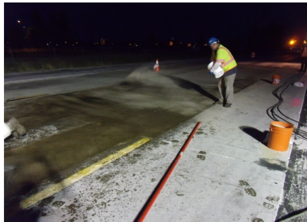
Figure 26. Top dressing wheel path inlay section.
