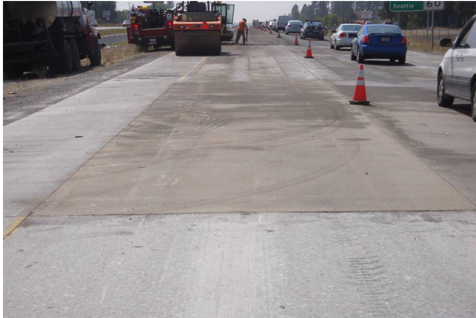
Figure 36. Both lanes of the full lane section of PPC.
