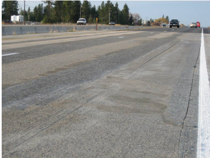
Figure 53. Wheel path inlay section after diamond grinding.
