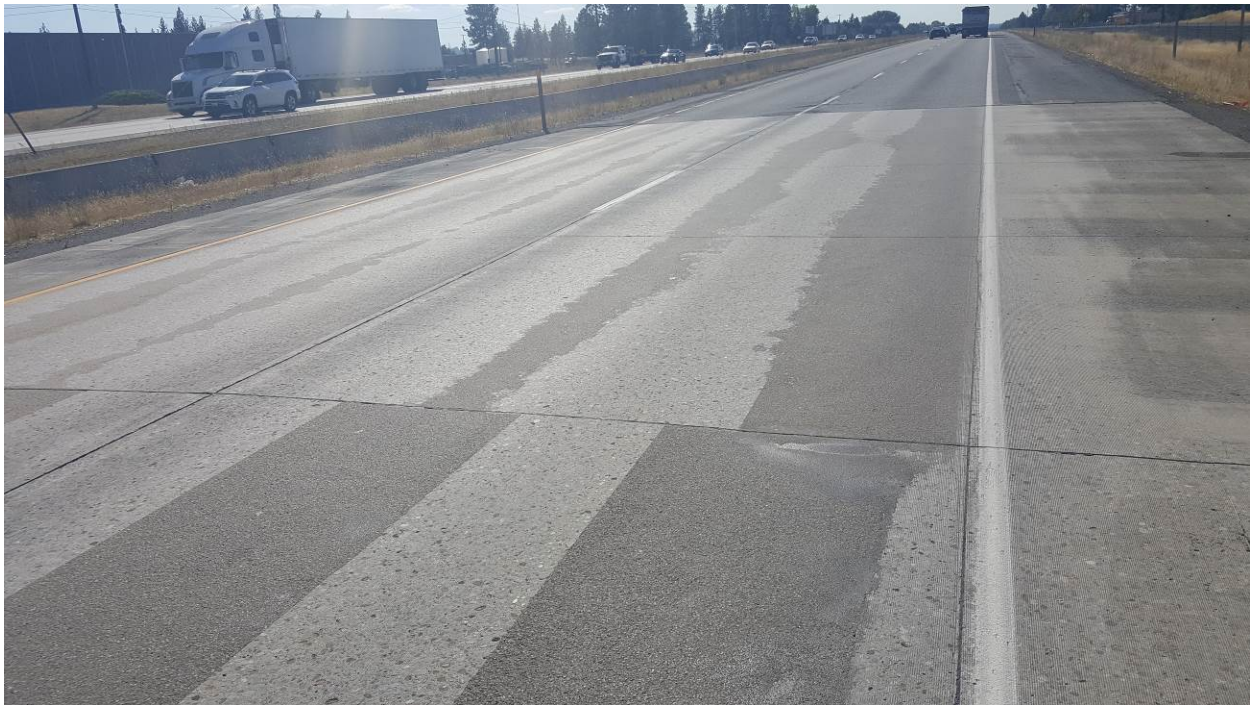
Figure 63. Longitudinal view of the section that was applied with a screed. No cracking or delaminations are visible (September 27, 2017)
