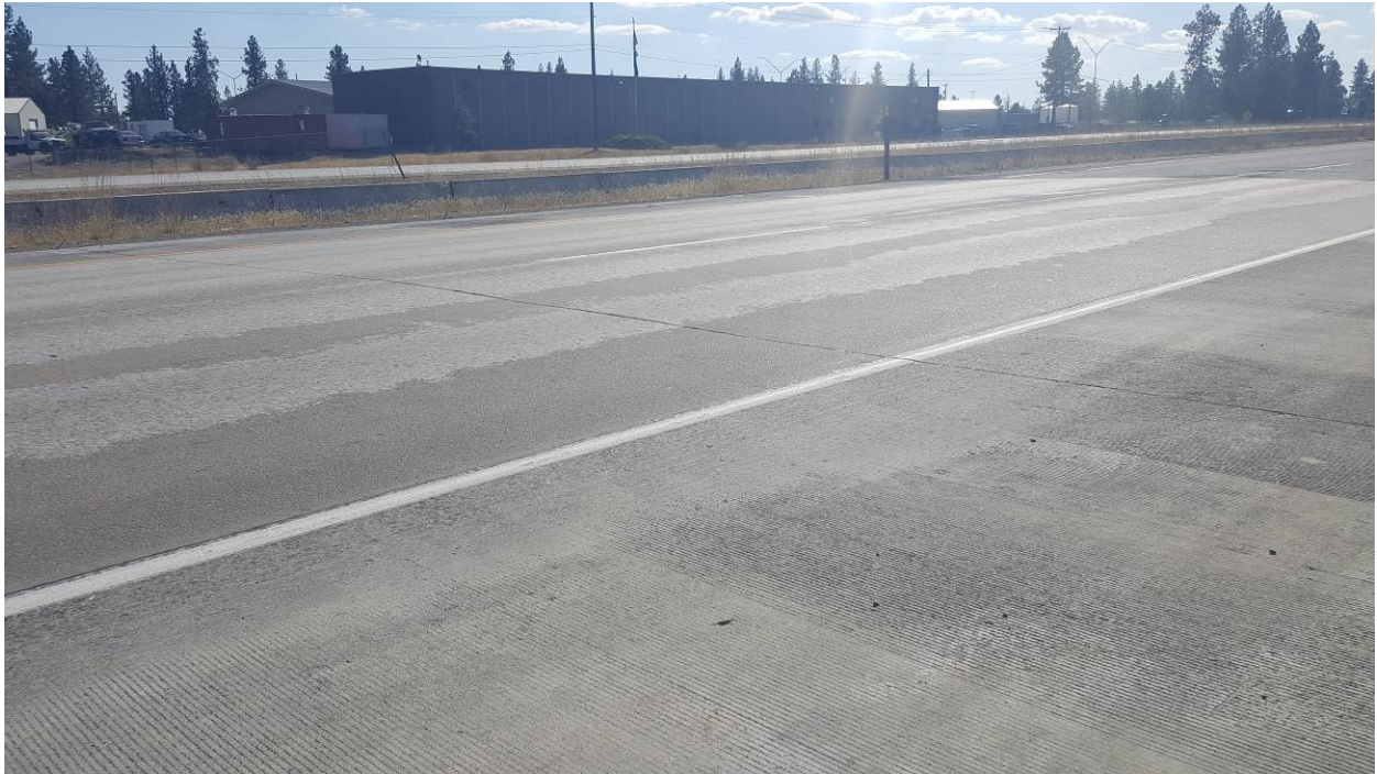
Figure 66. Side view of the section that was applied with a screed. No cracking or delaminations are visible (September 27, 2017).
