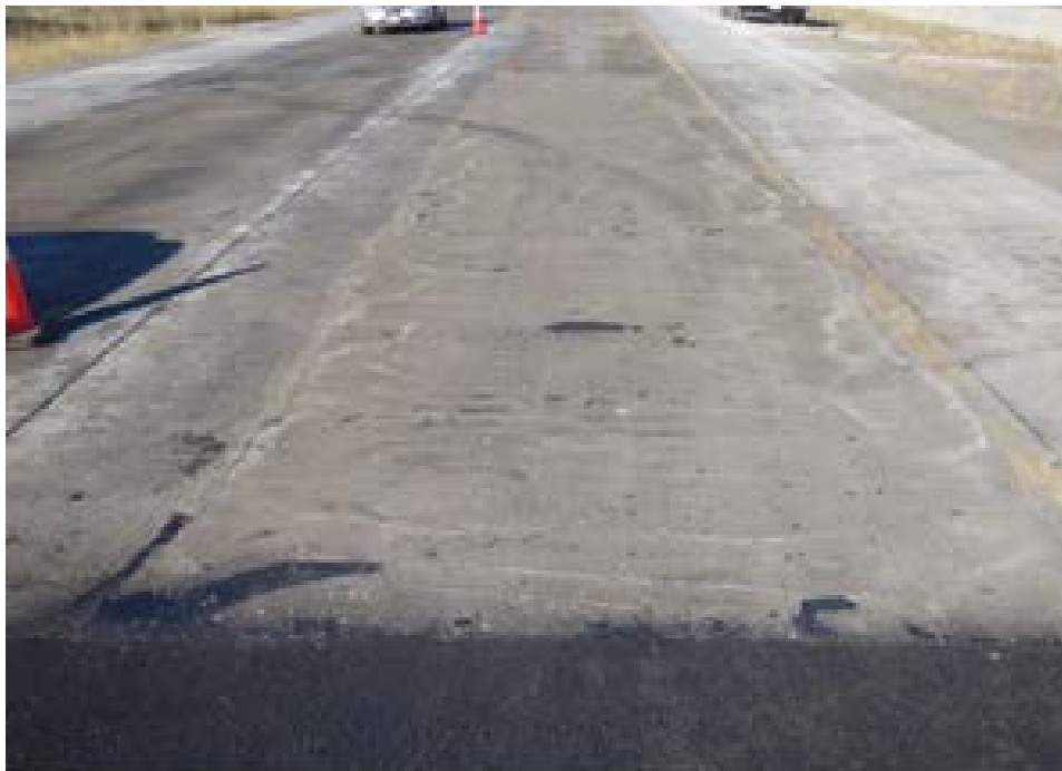
Figure 43. End view of rut fill section of PPC.
