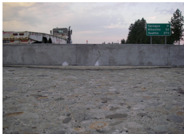
Figure 30. Amount of wear in rut fill section.
