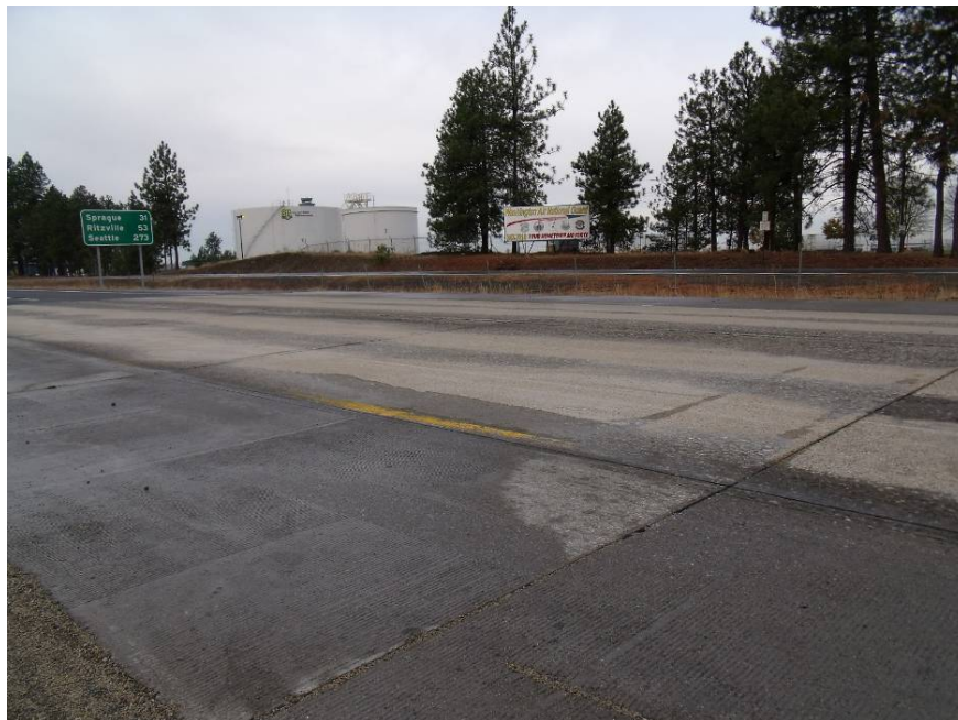
Figure 56. Rut fill section after diamond grinding.
