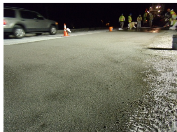
Figure 17. Finished PPC after top dressing with aggregate.
