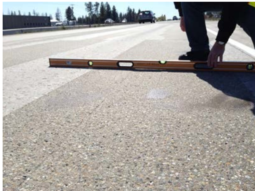
Figure 58. Wheel path inlay section after diamond grinding.
