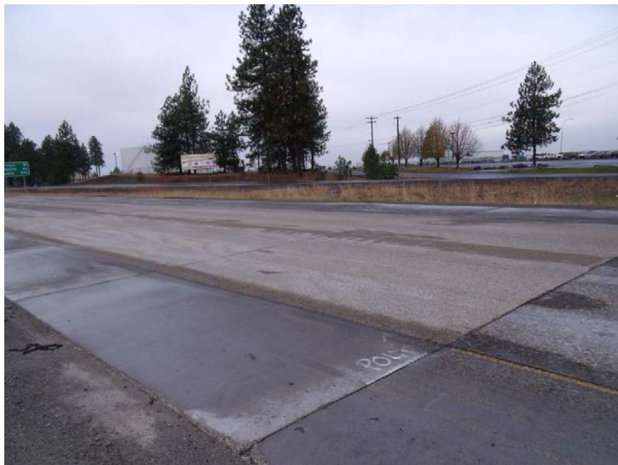
Figure 46. Full lane inlay section after diamond grinding.
