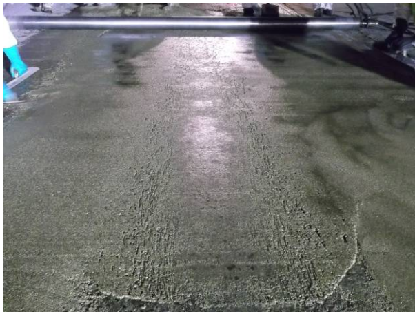
Figure 33. Finished PPC in the rut fill section.
