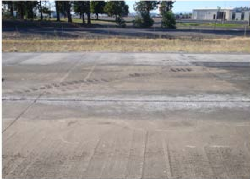
Figure 44. Side view of both lanes of the rut fill section of PPC.
