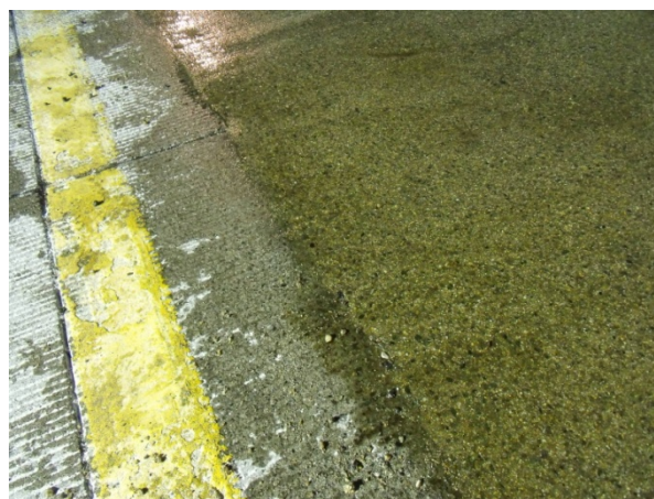
Figure 32. Close-up of finished PPC prior to top dressing with aggregate.
