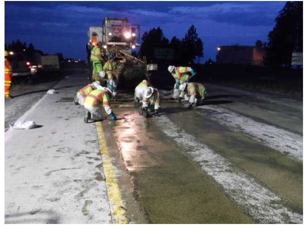
Figure 25. Final hand toweling of the wheel path inlay section.
