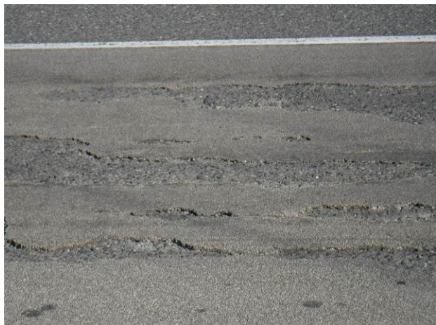
Figure 38. Delamination close-up.
