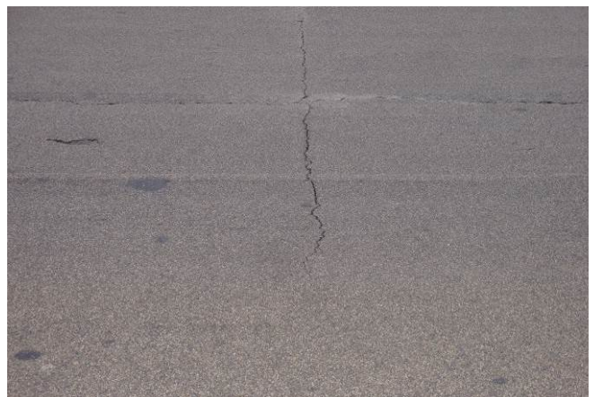
Figure 32. Transverse crack.
