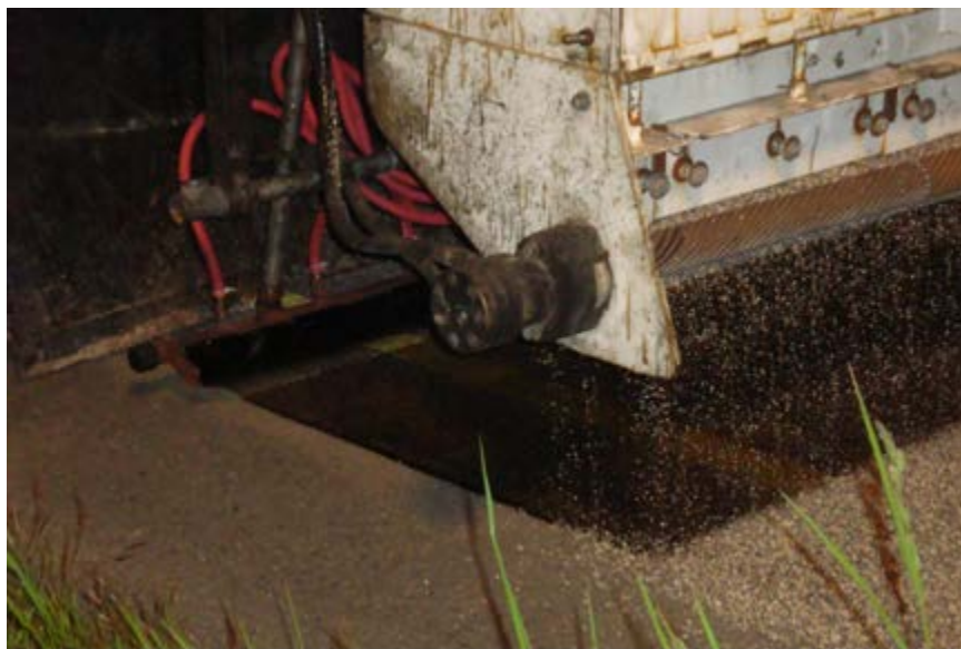
Figure 20. Close-up of spreader bar distributing epoxy binder and aggregate spreader dropping material on top of the epoxy.
