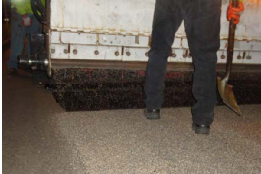
Figure 19. Aggregate being applied to epoxy after being placed on the pavement surface.
