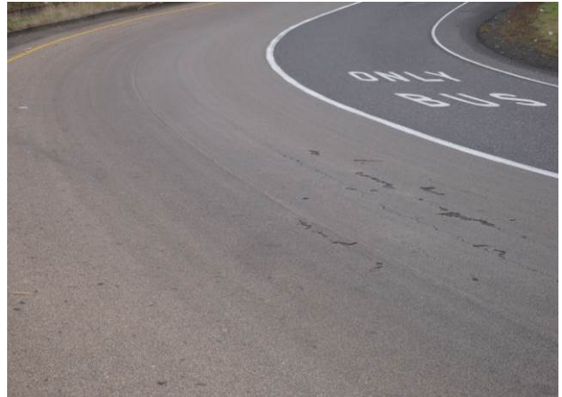
Figure 28. Random delamination.
