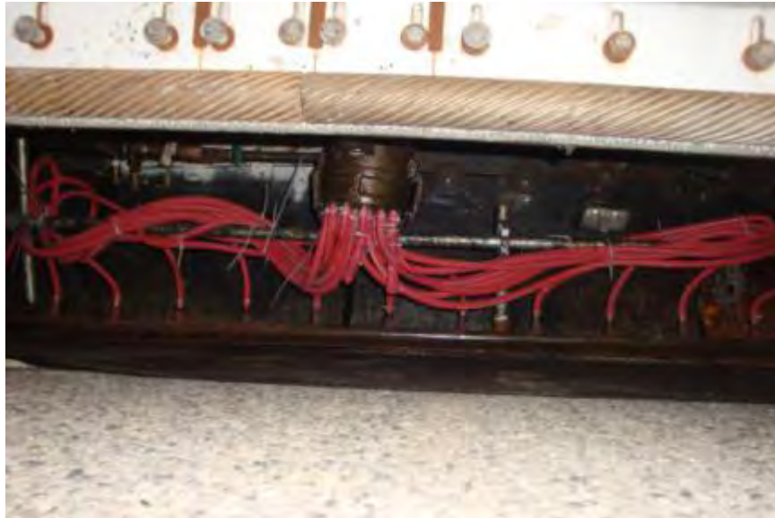
Figure 18. Multiple hoses used to distribute epoxy binder from the mixer to the spreader.
