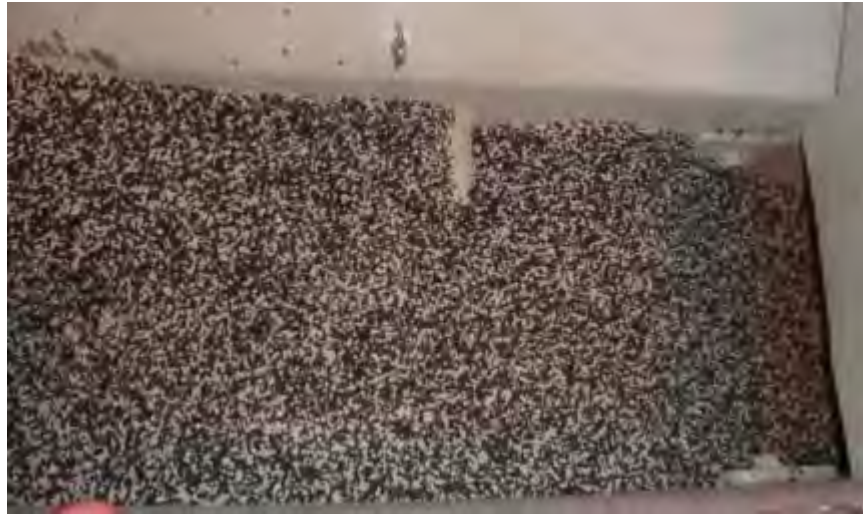
Figure 5. Aggregate in spreader box prior to production.
