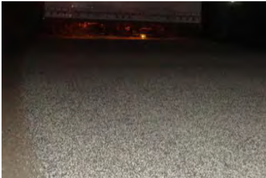
Figure 11. Illustration of uniform aggregate placement.
