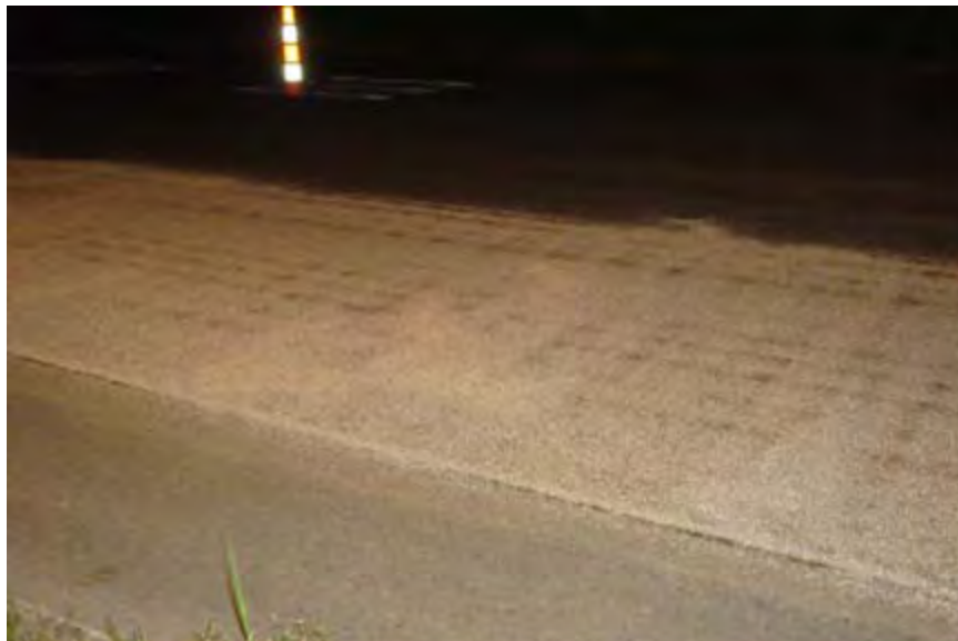
Figure 21. Completed installation prior to the removal of the excess aggregate.
