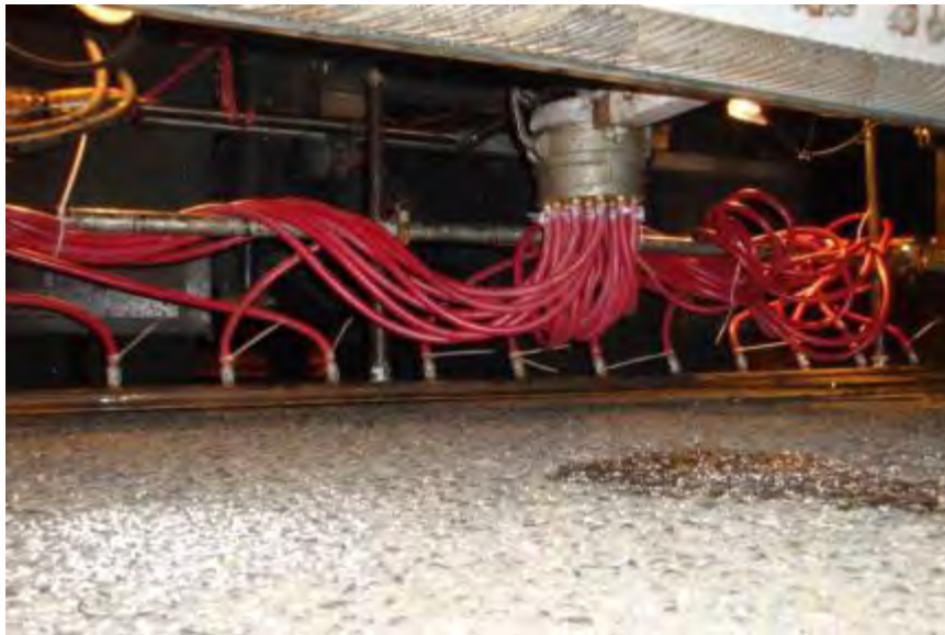
Figure 4. Supply hoses and spreader bar prior to production.
