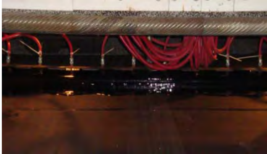
Figure 7. Epoxy resin extruded over spreader plate onto roofing material at startup location.
