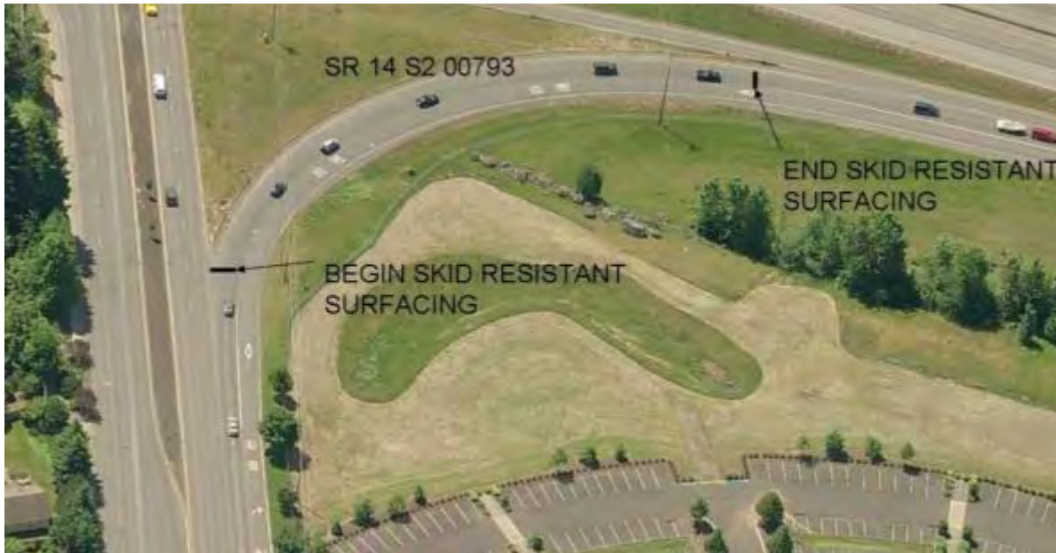
Figure 1. Approximate limits of Tyregrip® installation on SR 14 S2 00793 ramp.
