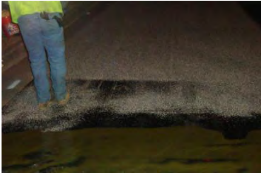
Figure 8. Hand placement of aggregate at beginning of project.
