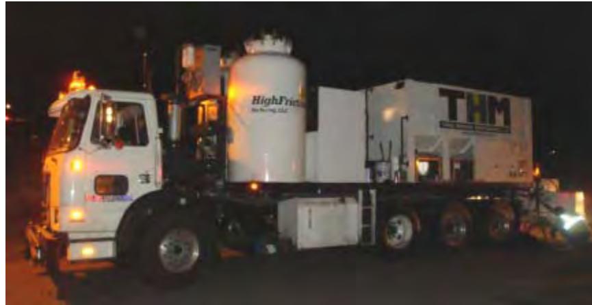
Figure 2. Vehicle used to mix and place epoxy binder and aggregates.
