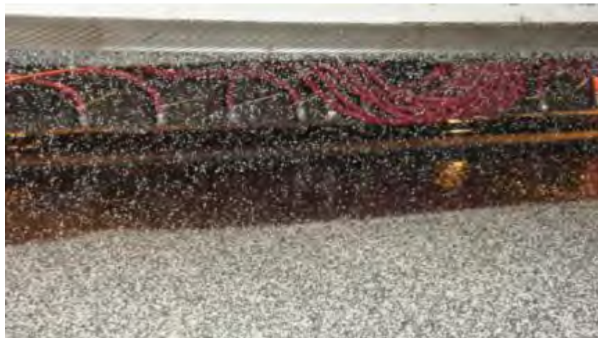
Figure 6. Aggregate dropping onto the extruded epoxy binder.
