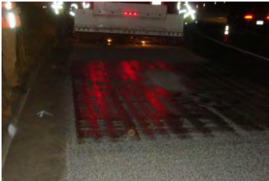
Figure 9. Location where aggregate spreader limited placement of material.
