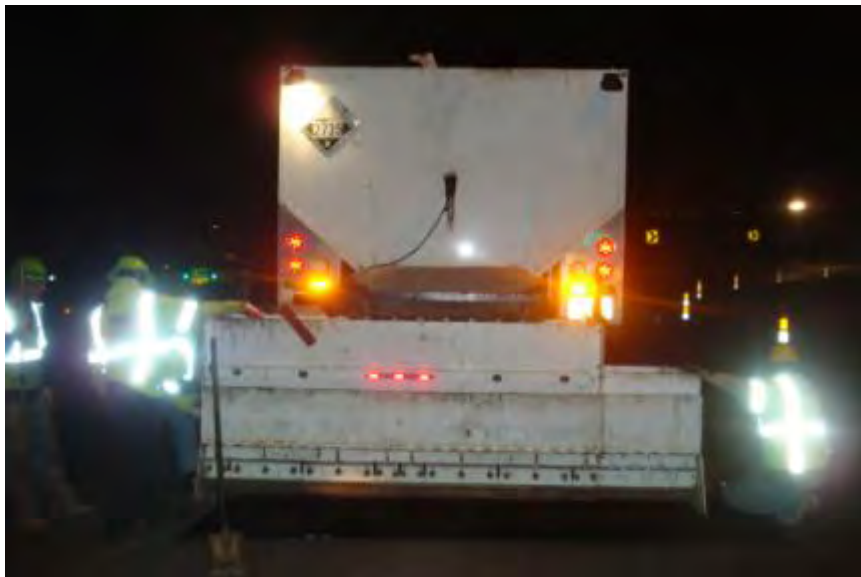
Figure 15. Application vehicle at start of the test section.
