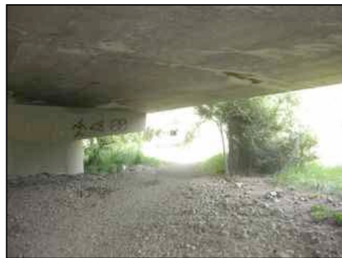
Figure 113. Trail under north structure
