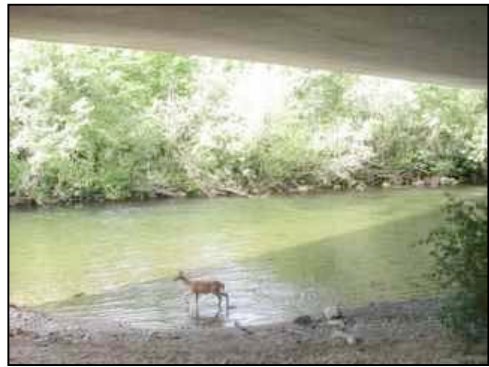
Figure 117. Doe crossing through structure along water's edge
