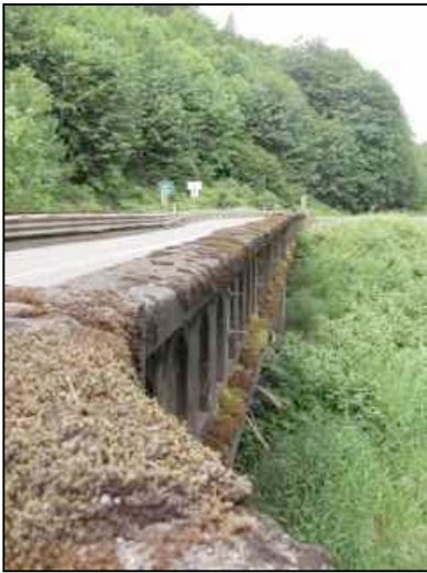
Figure 45. Bridge and adjacent forest
