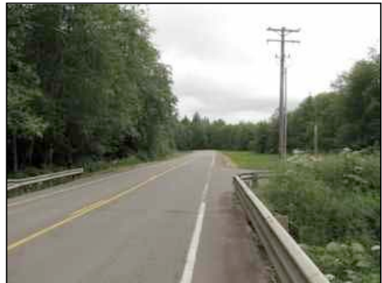
Figure 13. Rte 101 looking South
