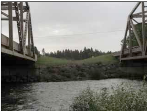
Figure 88. East side median
