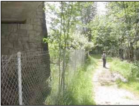
Figure 116. Chain link fencing
