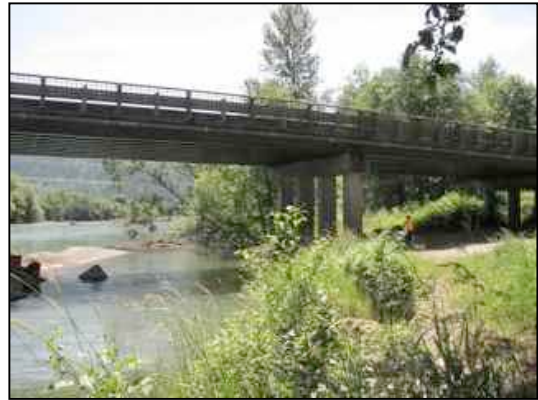
Figure 54. Looking towards inlet
