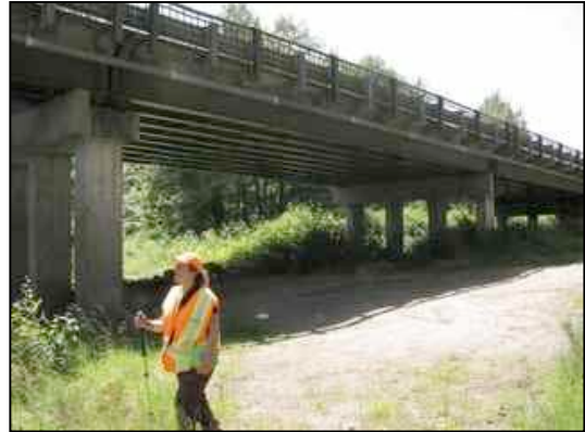
Figure 52. Terrestrial area beneath bridge
