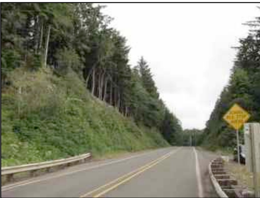
Figure 20. Roadway looking south
