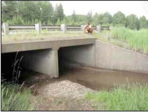
Figure 96. South side outlet
