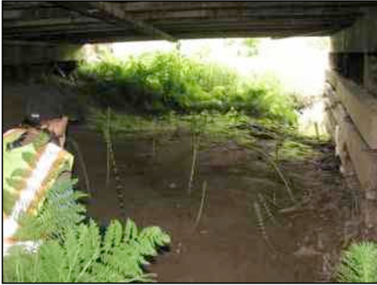
Figure 16. Stream bank under outside span
