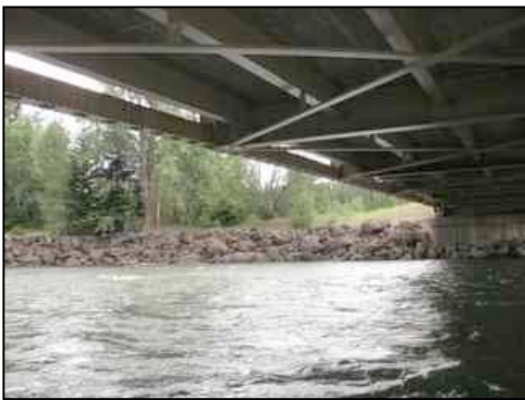
Figure 86. Riprap banks on east side of river
