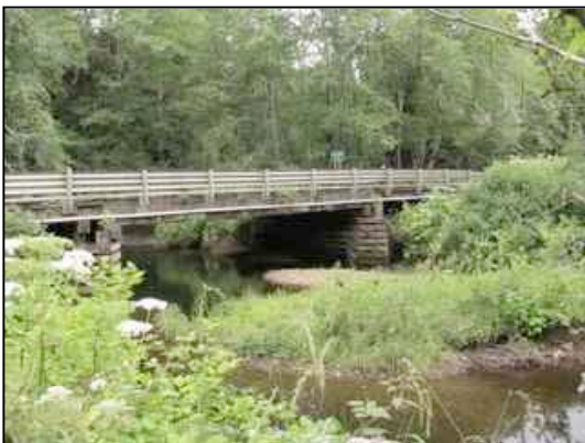
Figure 14. Bridge at Location 101_38.8_02
