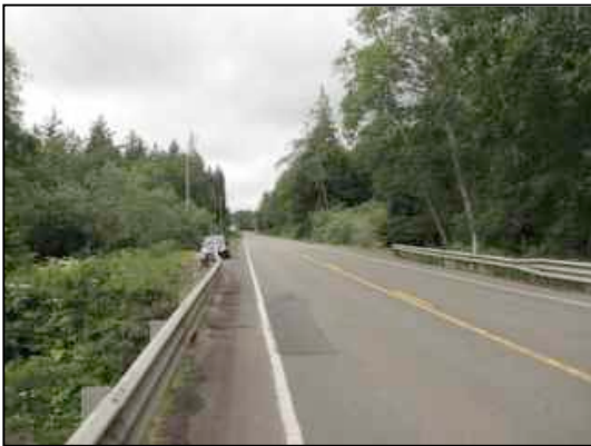
Figure 12. Rte 101 looking North
