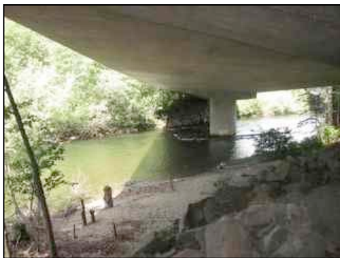
Figure 112. Beneath north structure
