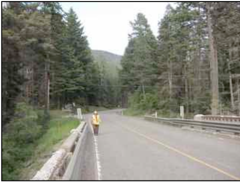
Figure 57. Roadway looking east
