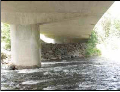
Figure 114. Riprap on west bank
