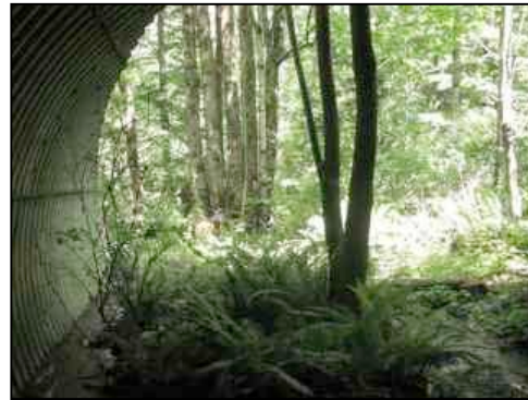
Figure 122. View from structure outlet
