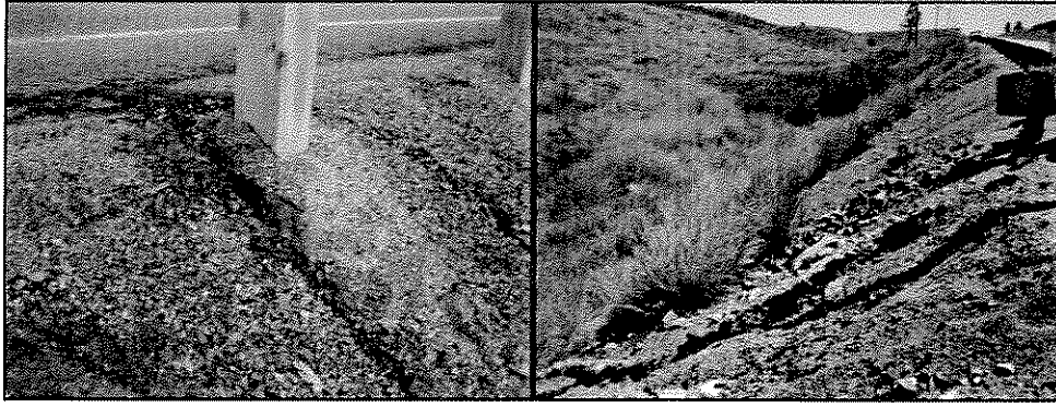
Figure 3.5 Erosion from Channelized Flow at Guard Rails
