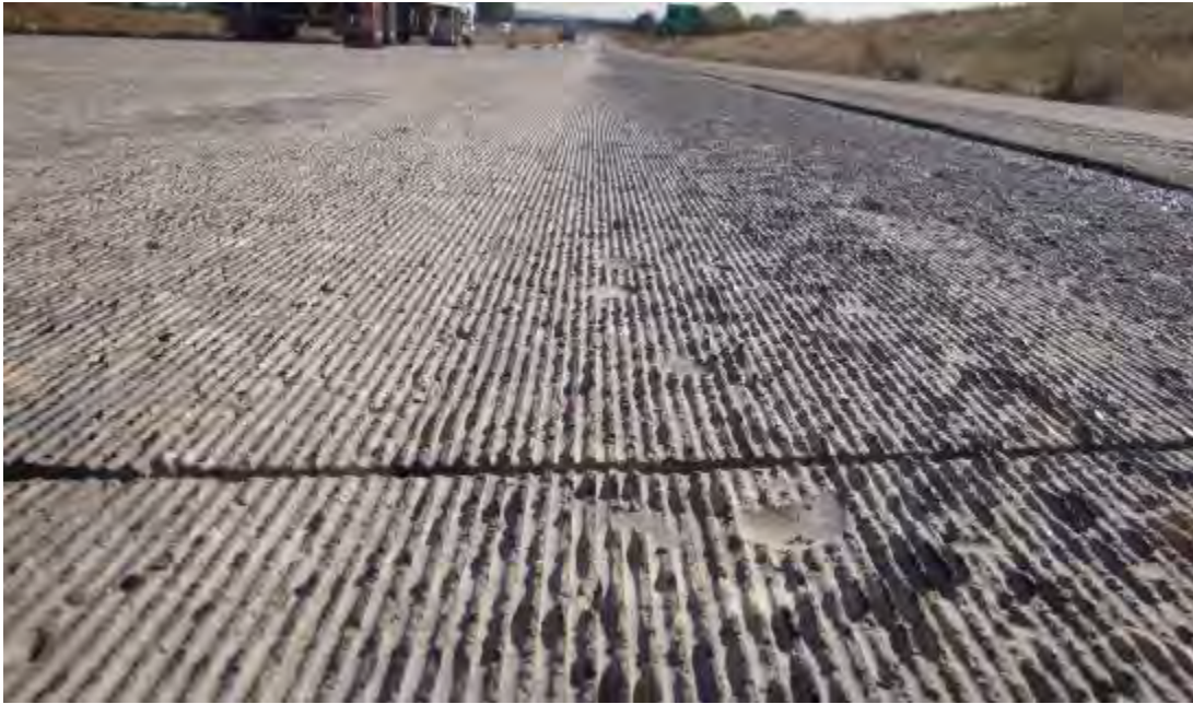
Figure 22. Roadway surface after conventional grinding.
