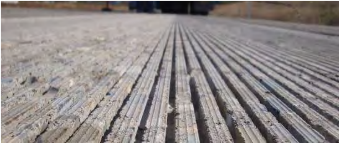
Figure 26. Pavement surface after tall blade grinding.
