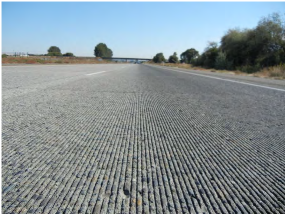
Figure 17. Another view of the attrition on the NGCS, note missing aggregate, October 2013.
