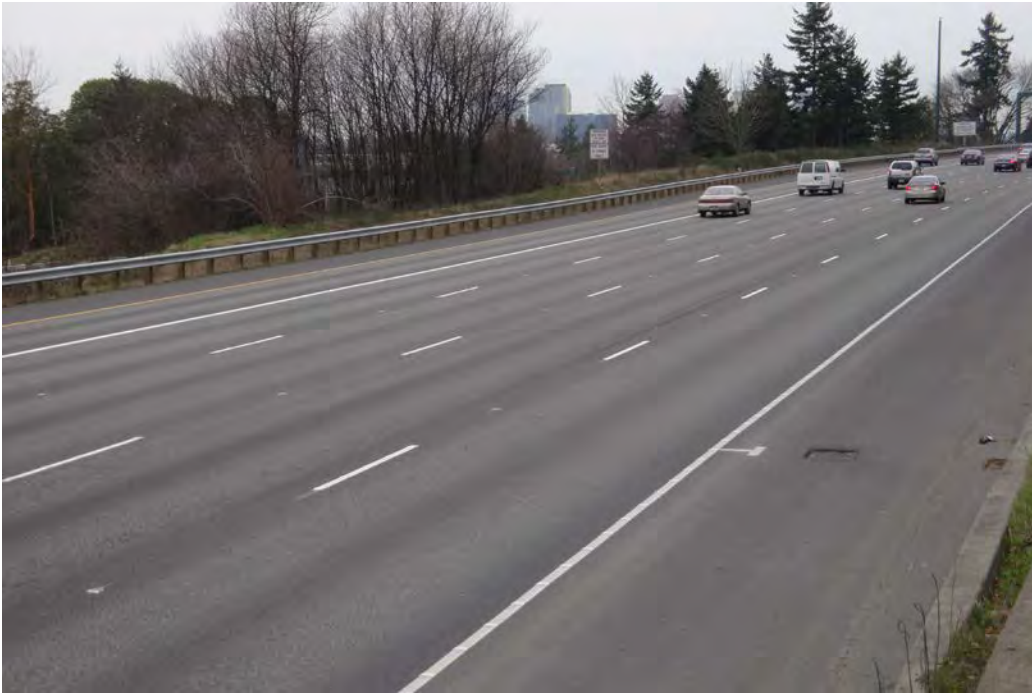
Figure 34. I-405 OGFC-AR section, note wear pattern in the wheel paths. (Photo taken 2/11/2011.)
