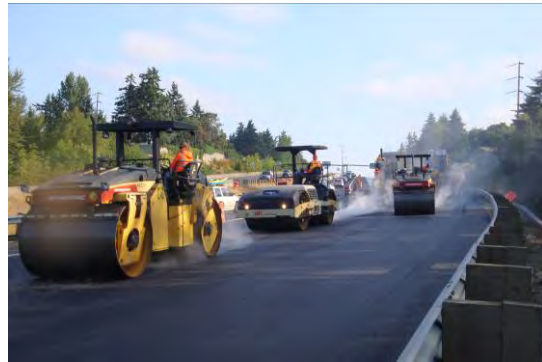
Figure 13. Rollers stayed close behind the paving machines.
