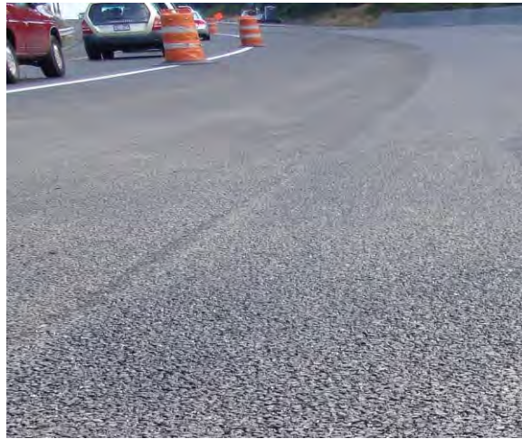
Image of the longitudinal joint
