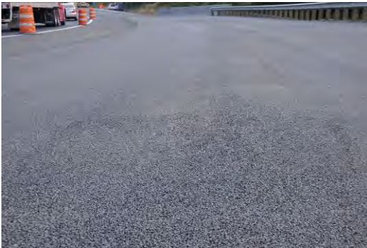
Figure 14. Finished OGFC-AR pavement.
