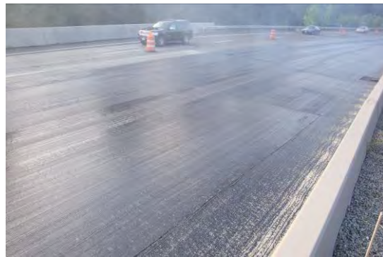
Figure 9. Tack coat application.
