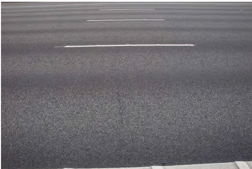
Figure 35. Transverse reflection crack from underlying concrete pavement in OGFC-AR section. (Photo taken 2/11/2011.)
