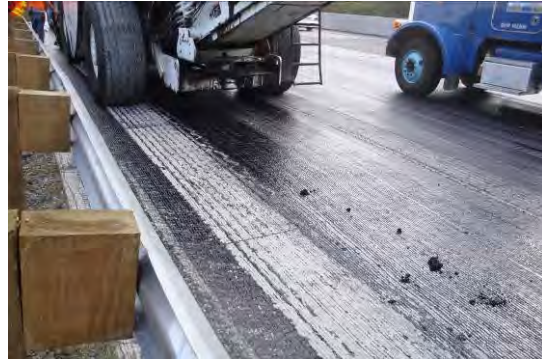
Figure 17. Bare streak left after PG asphalt tack picked up by Shuttle Buggy tire.
