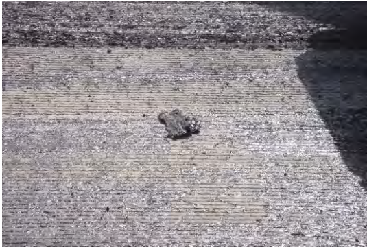
Figure 20. Piece of tack buildup from tires left in front of paver.
