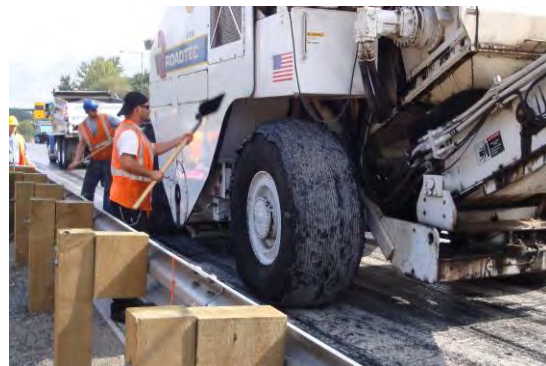
Figure 19. Members of paving crew removing tack buildup.
