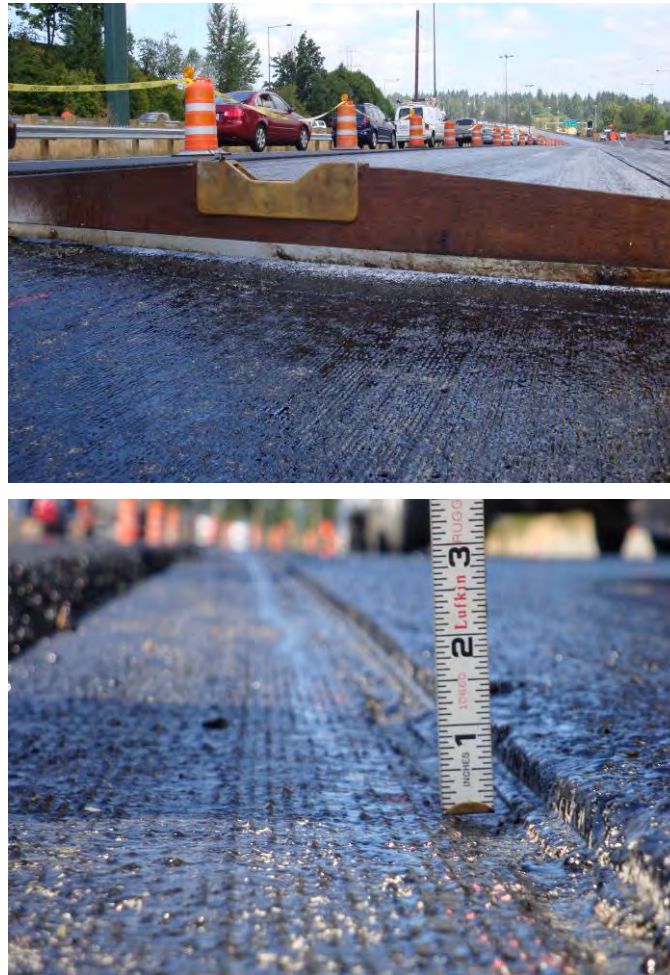
Amount of rutting present after milling
