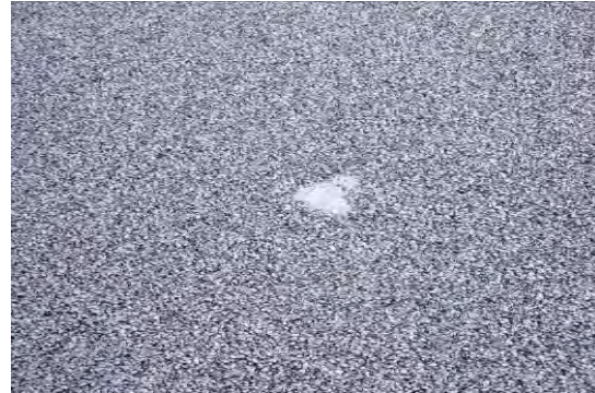
Figure 21. Fat spot resulting from a piece of tack buildup from tires.
