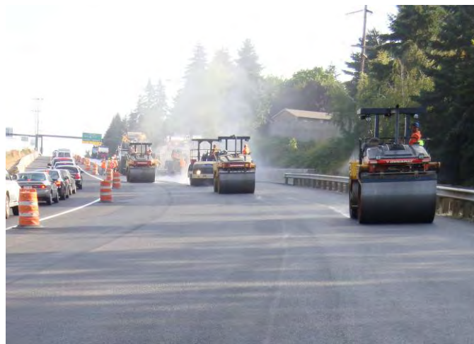
Looking at breakdown and intermediate rollers
