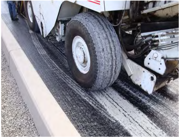
Image of tack pickup on new PCCP
