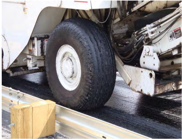
Pickup of tack when temperature was warmer
