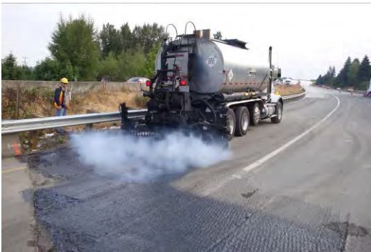
Figure 8. Distributor applying tack coat.
