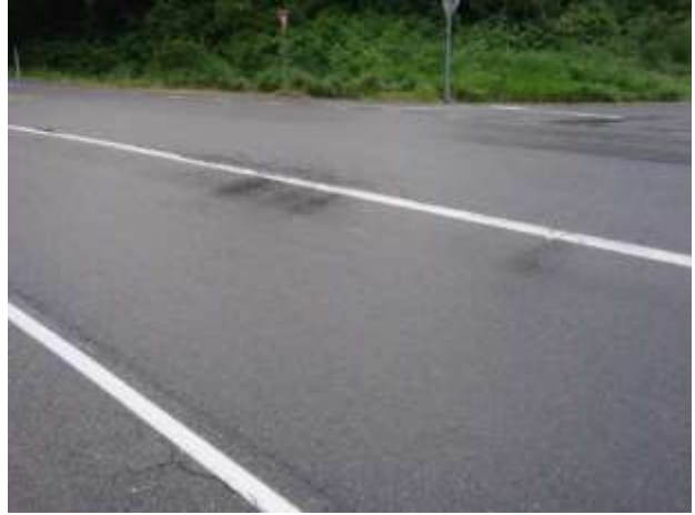
Figure 28. Alligator cracking at MP 14.5. (4818)
