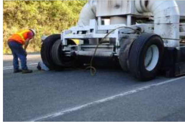
Figure 3. Removing rubber tires prior to paving.
