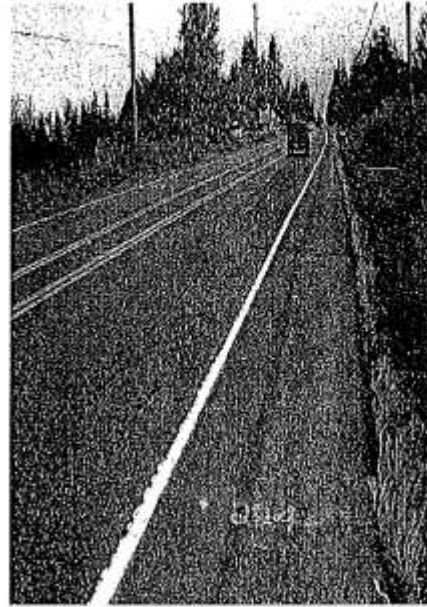
Photo 4 (~MP 7.05): Medium to high severity transverse and longitudinal cracking
