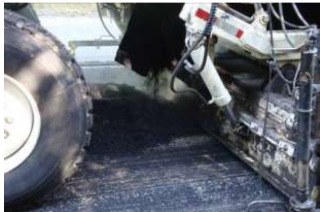
Figure 11. Windrowing of millings from unit B with millings from conveyer.
