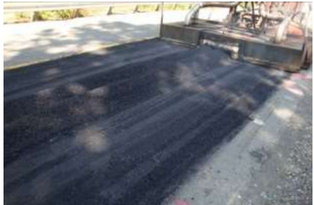
Figure 7. Milled HMA behind unit A is windrowed into the center of the lane.
