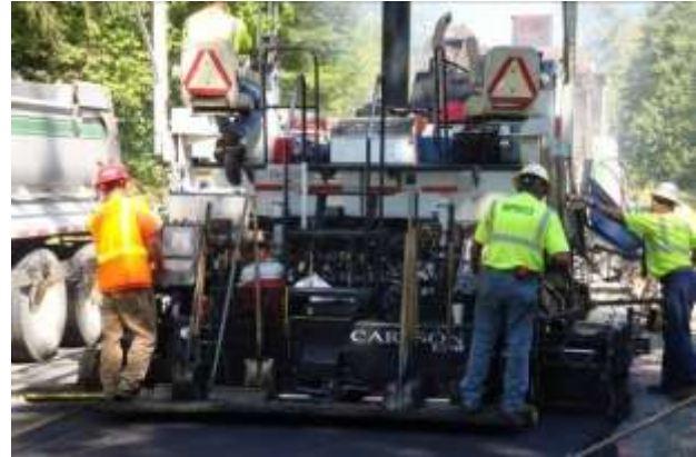
Figure 13. Rear view of RoadTec paving machine.
