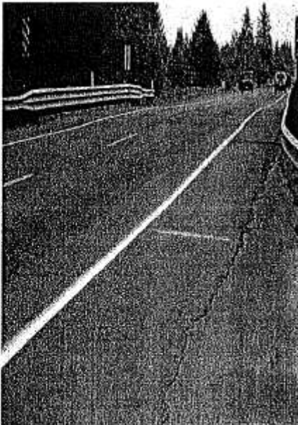
Photo 5 (~MP 11.29): Maintenance patching of HMA over the bridge deck # 542/016.
