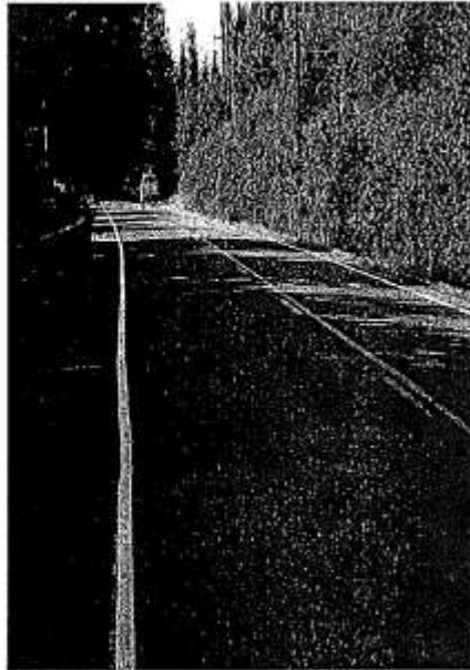
Photo 7 (~MP 16.65): Medium severity transverse and longitudinal cracking that was patched with HMA by maintenance crews.
