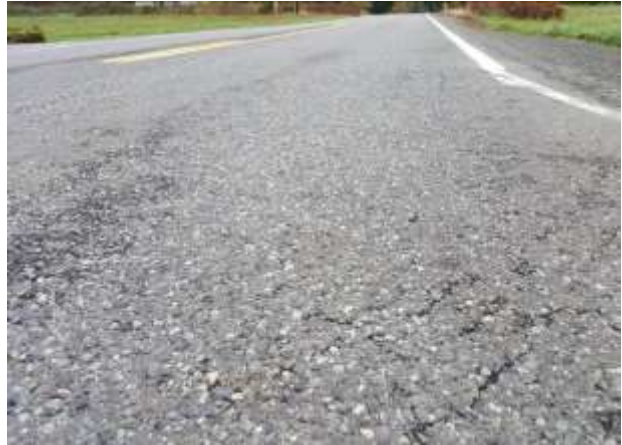
Figure 43. Close-up view at MP 17.2. (94003)
