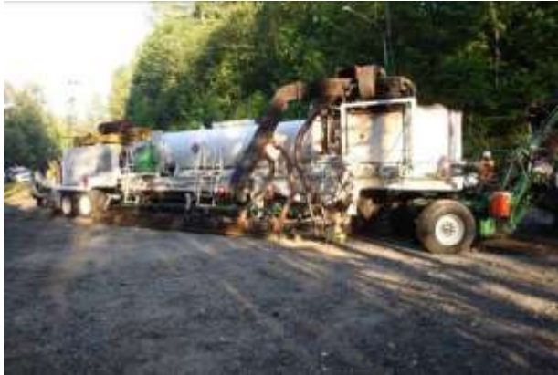
Figure 8. Left rear of unit B.
