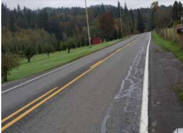
Figure 42. Sealed cracks at MP 17.1. (93723)
