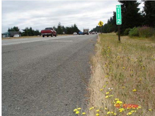
A sloping pavement edge takes the place of a gravel strip in this case and requires no maintenance.
