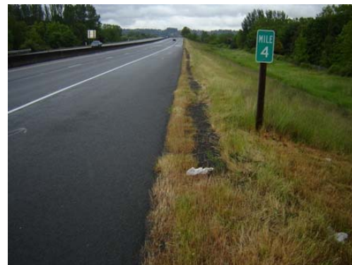
By the end of the study period six years after construction, the strip of compacted grindings is over 50% grass cover. Grass establishment could be prevented with Glyphosate treatments on a 2 to 3 year or as needed basis.
