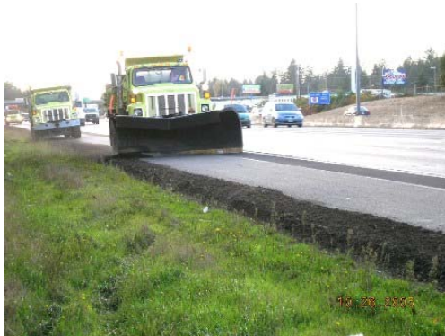
This photo shows how the operation of cultivation works. A plow truck pushes the turned material back into place and the two buffer vehicles drive over the edge, packing it back into place.
