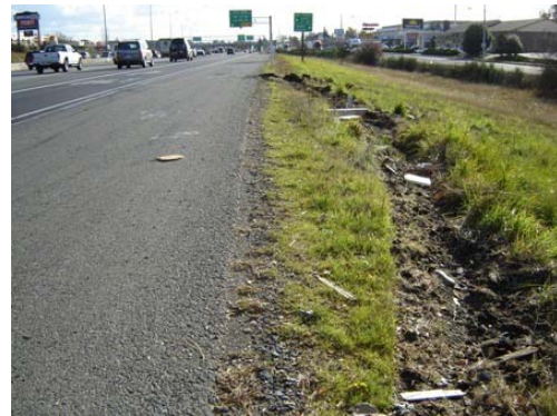
At one point an errant vehicle left and returned to the road right at the location where the monthly documentation photos were taken, illustrating the importance of having a solid and even transition between paved and non-paved shoulder.
