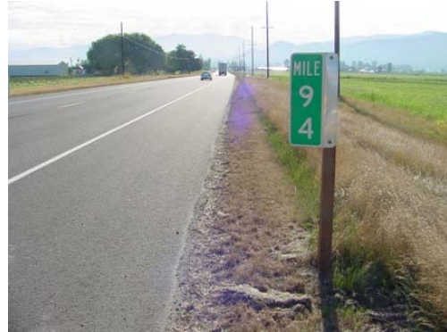
Where annual applications were skipped in certain years and locations, grasses became established. The presence of vegetation, even if dead tended to make subsequent applications less effective, because herbicide was tied up in organic matter on the surface. Also, even dead vegetation at the pavement edge contributes to edge buildup.
