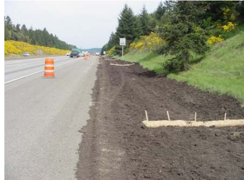
A compost blanket was added to outside shoulders and median for enhanced stormwater management and pollution control along the section of freeway draining toward the Nisqually Delta.
