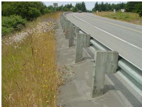
On the north end of Whidbey Island the same product was installed by a contractor along with a new section of guardrail in 2006. At the time this photo was taken in June of 2009 it appears to be holding up well without maintenance attention.
