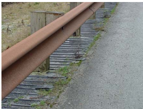
Tiles were damaged by snow and ice thrown by passing plow trucks.
