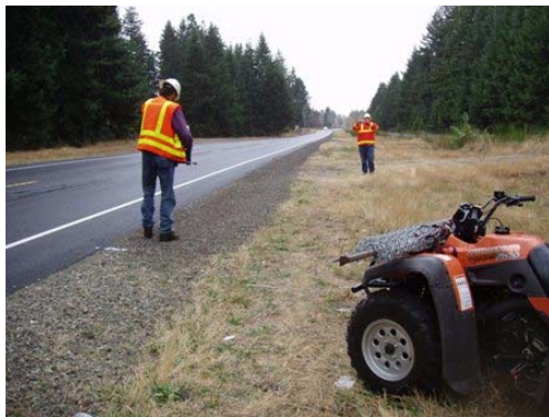
Spreading seed by hand and raking in with an ATV and chain link proved effective and less expensive than hydro-seeding.
