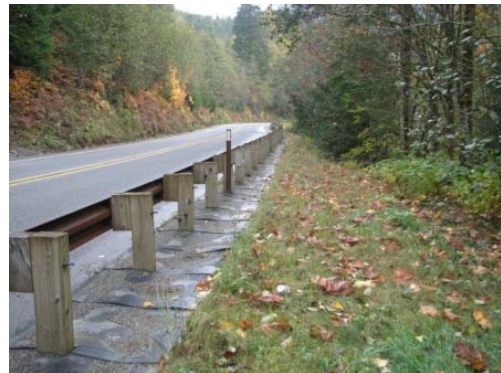
This is the mat after three years. Some sand build-up, but it seems to blow or wash off over the course of each summer, no maintenance has been done at this location.
