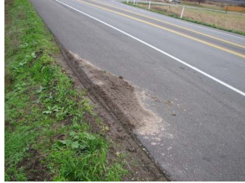
Tires tend to sink into shoulder when vehicles drive off pavement and even got stuck in wet conditions.
