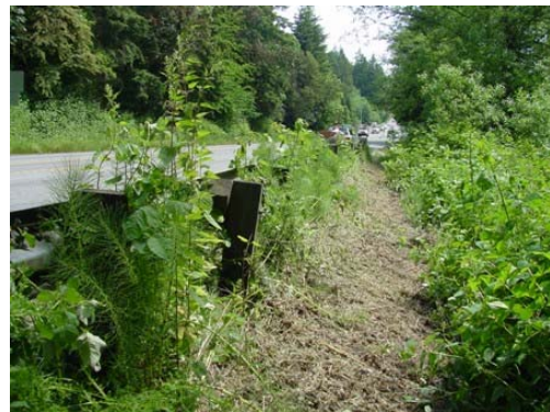
Two years after reconstruction low growing grass seeded on the shoulders and under guardrail is overgrown by weeds and blackberry vines throughout most of the highway corridor on the island.
