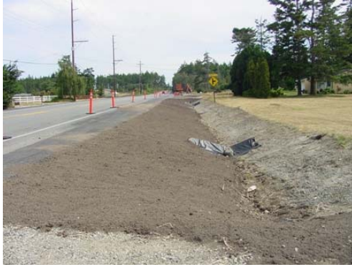
Topsoil placed during construction was subject to erosion due to the fine particles in soil structure.
