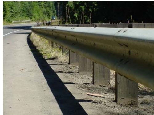
Vegetation and buildup under guardrail has been removed manually on a three year cycle since herbicide use was discontinued in the early 1990's.
