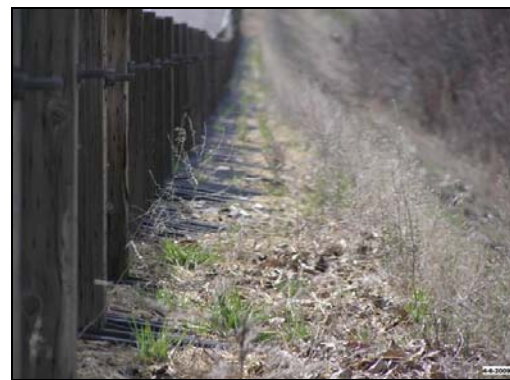
SR 826, fall 2009- Cracked and damaged matting with vegetation growing up through the mats.
