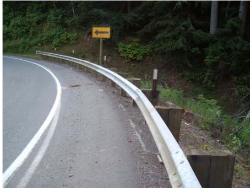
These pictures, taken at the same time three years after installation show the difference in accumulation of debris between inside corner with curb on the edge of pavement and the outside corner.
