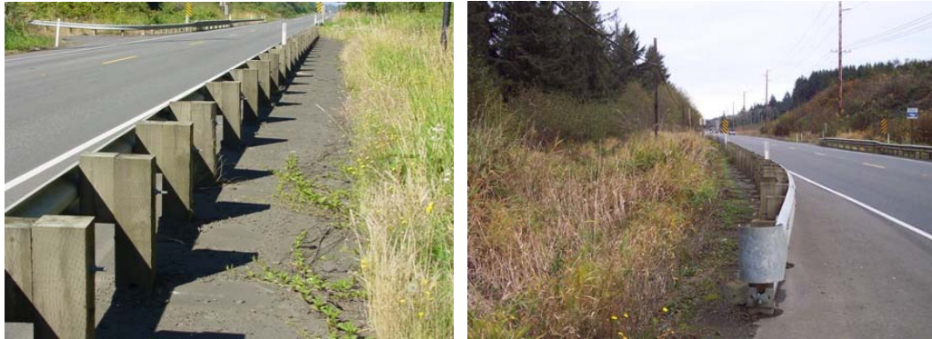
New pavement and guardrail was installed in 2003. Photo on the left shows condition in 2005 after two years, photo on the right is from 2007 showing debris accumulation after four years. Rails along this section of SR 105 were cleaned in 2008.
