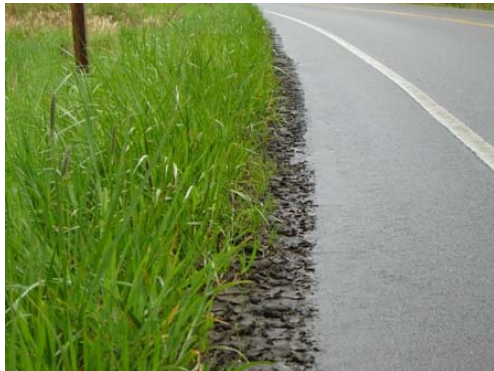
Sediment buildup tends to accumulate along the edge of pavement more rapidly at low spots and insides of curves.
