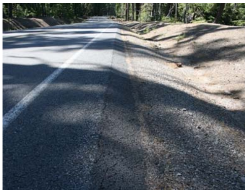
On SR 62 in Oregon (Crater Lake Highway) a safety edge is used in combination with an adjacent shoulder free of vegetation.
