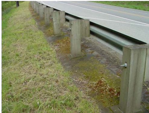
At about 5 years after installation in this case, moss growth became a significant factor. Moss in combination with debris from falling leaves and cut grass and brush serves as a seed bed unless annual cleaning is done.
