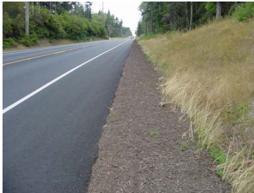
A compost layer is less expensive than top course crushed rock and aids in stormwater management. Course grade material compacts for a drivable surface.
