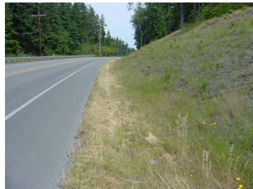
5 years after construction this location has a well established grass stand and less edge buildup than other locations, shown here recently mowed with sickle bar.
