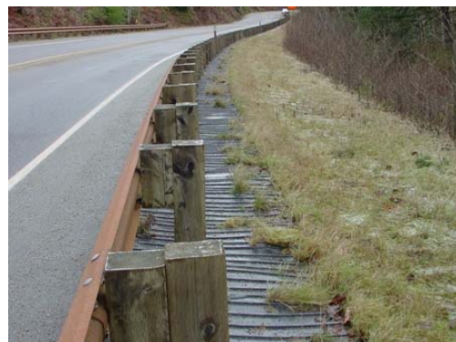
Grass came through where the panels joined together and where the material cracked.
