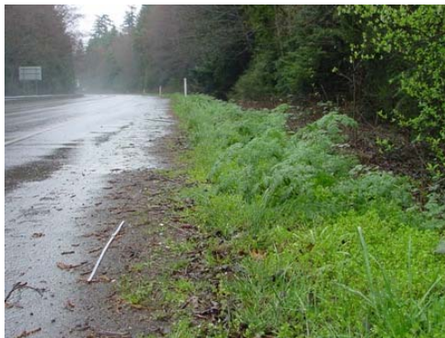
Although this image does not show guardrail it does the amount of debris that accumulates on the shoulder and the amount of weed growth two years after shoulder reconstruction.
