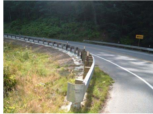
These pictures, taken at the same time three years after installation show the difference in accumulation of debris between inside corner with curb on the edge of pavement and the outside corner.
