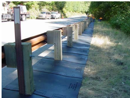
The Traffix Weed Mat were the easiest of the under guardrail products to install. This is the product being installed in 2006.
