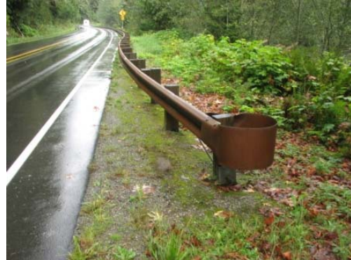
Three years after installation the mat is buried in sand and debris. Vegetation is beginning to establish over the top of the mat but growth is inhibited.
