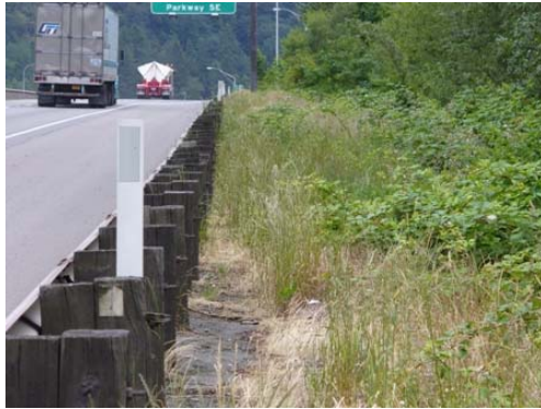
Six years since the site was last cleaned, enough dirt and debris has deposited to support a grass stand over the pavement.
